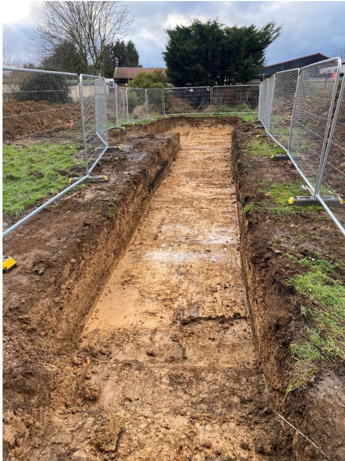
Plate 3: Trench 3 facing northwest
