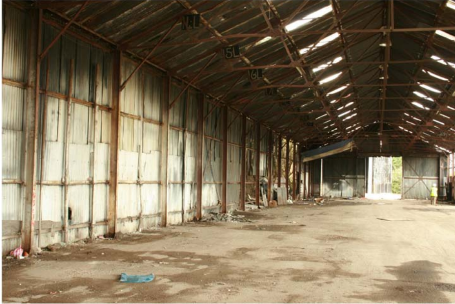
Plate 9 General internal view of Shed 1, looking north-west
