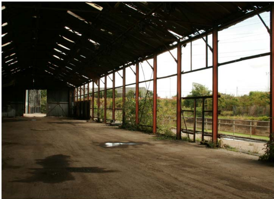
Plate 4 Internal view of north end of Shed 1, looking north-east
