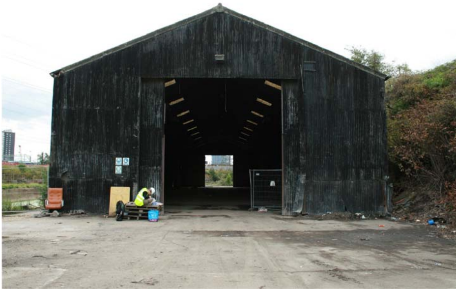
Plate 13 North-west elevation of Shed 2, looking south-east
