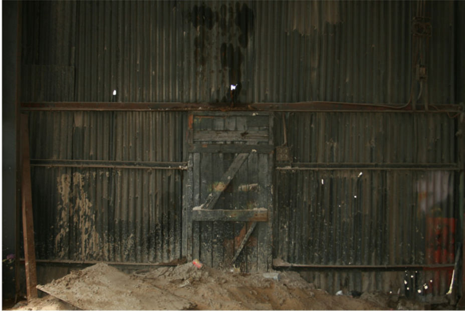
Plate 3 Pedestrian access door in Shed 1, looking south
