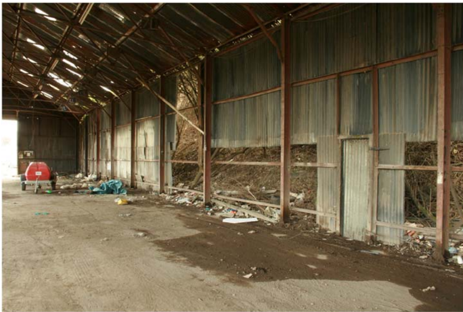
Plate 6 Internal view of south-west corner of Shed 1, looking south-west
