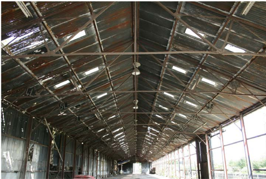
Plate 8 Roof trusses, skylight types 1 and 2 and artificial lighting in Shed 1
