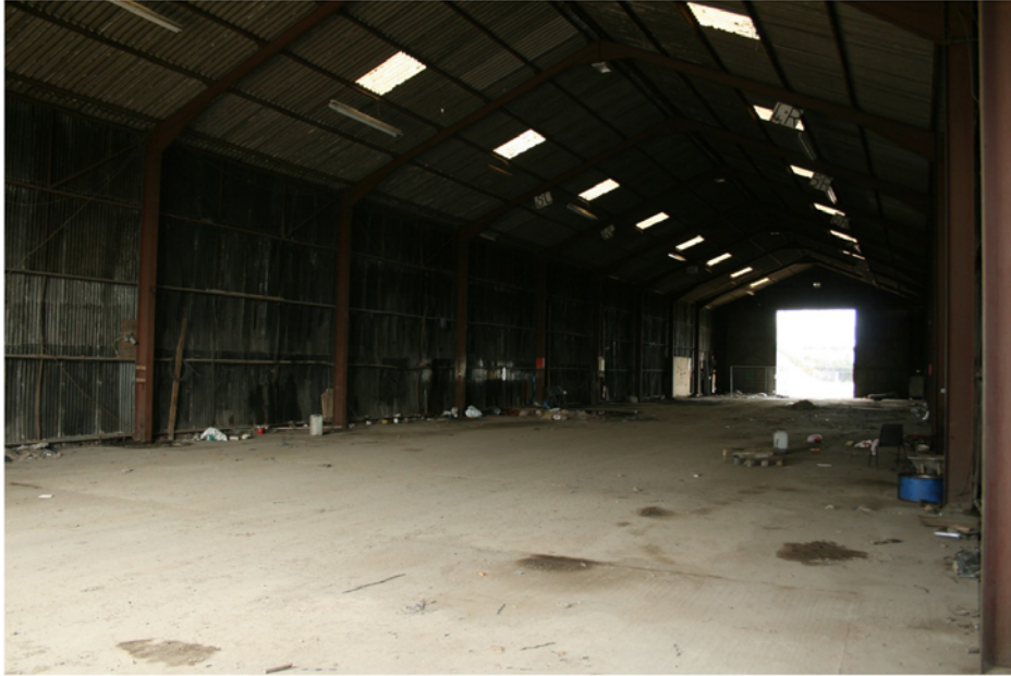
Plate 14 General internal view of Shed 2, looking north-west
