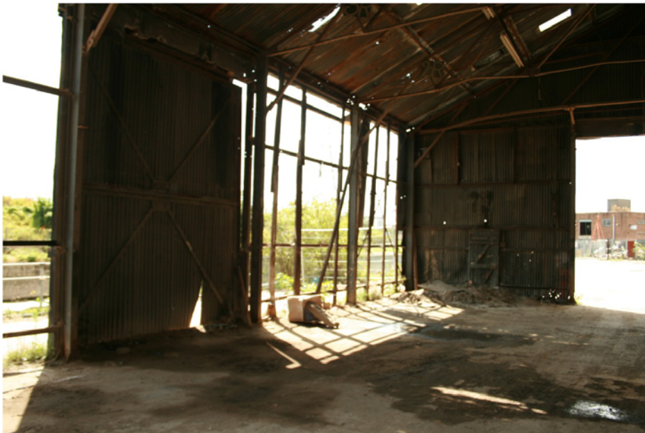
Plate 2 Internal view of south-east corner of Shed 1, looking south-east
