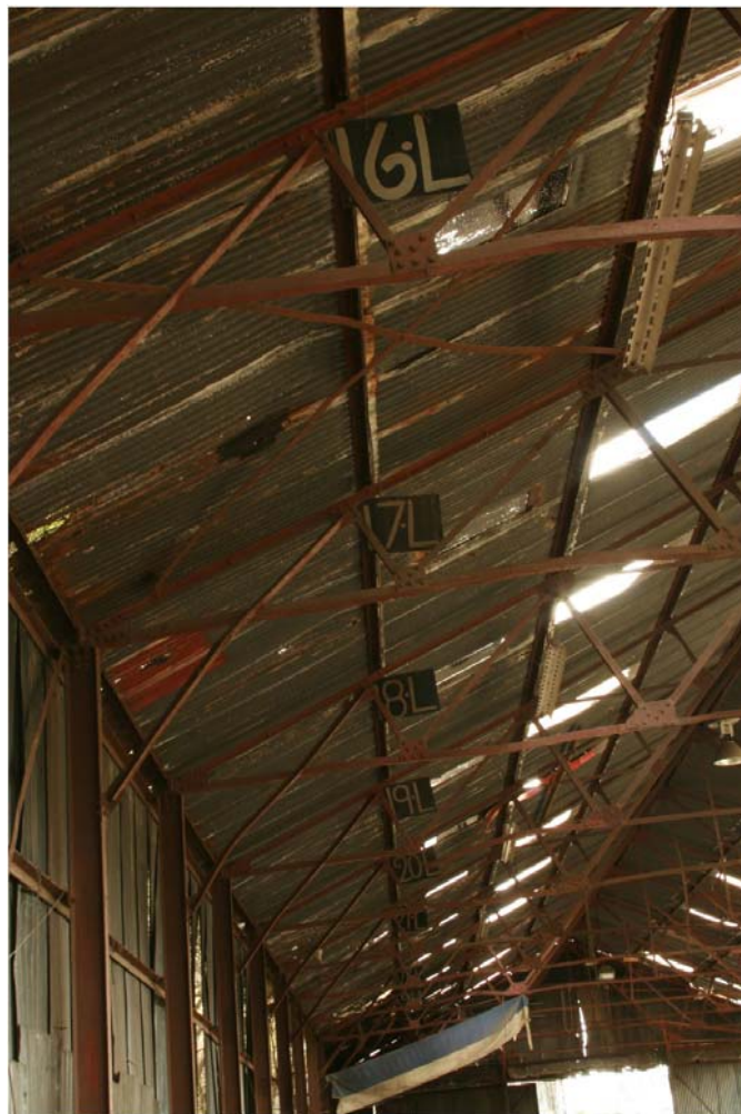
Plate 10 Numbered plates hanging from trusses in Shed 1
