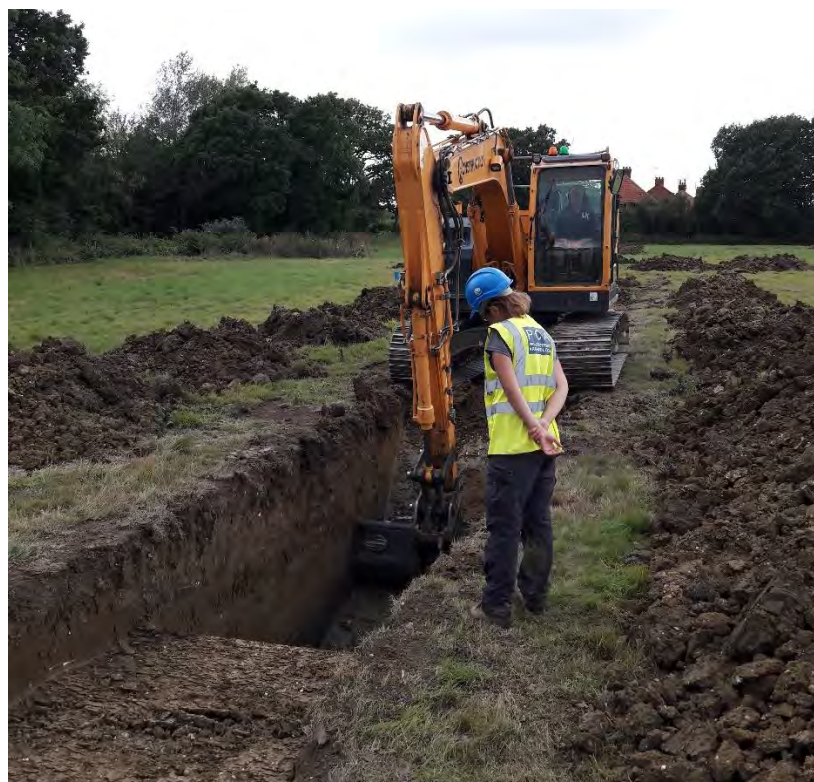
Plate 8: Machine excavation of pond [612] to reach lower deposits.
