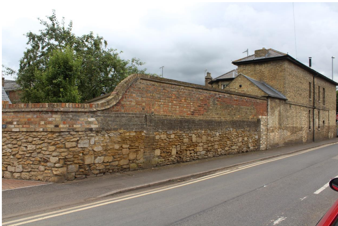
Plate 6: View of wall on south side of Victoria Street; view south-east
