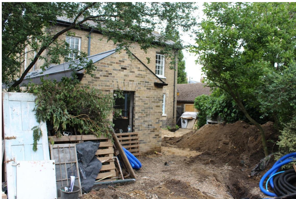
Plate 1: View of house, view north-west
