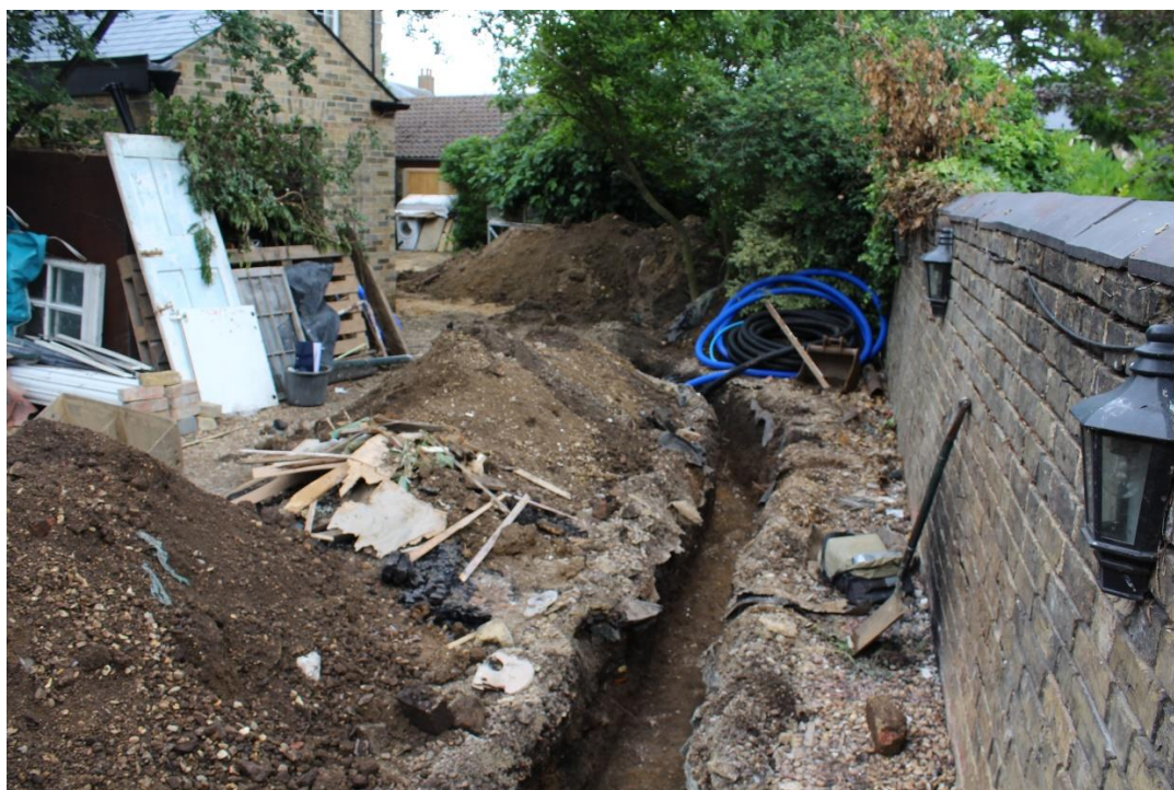
Plate 5: The pipe trench, view north
