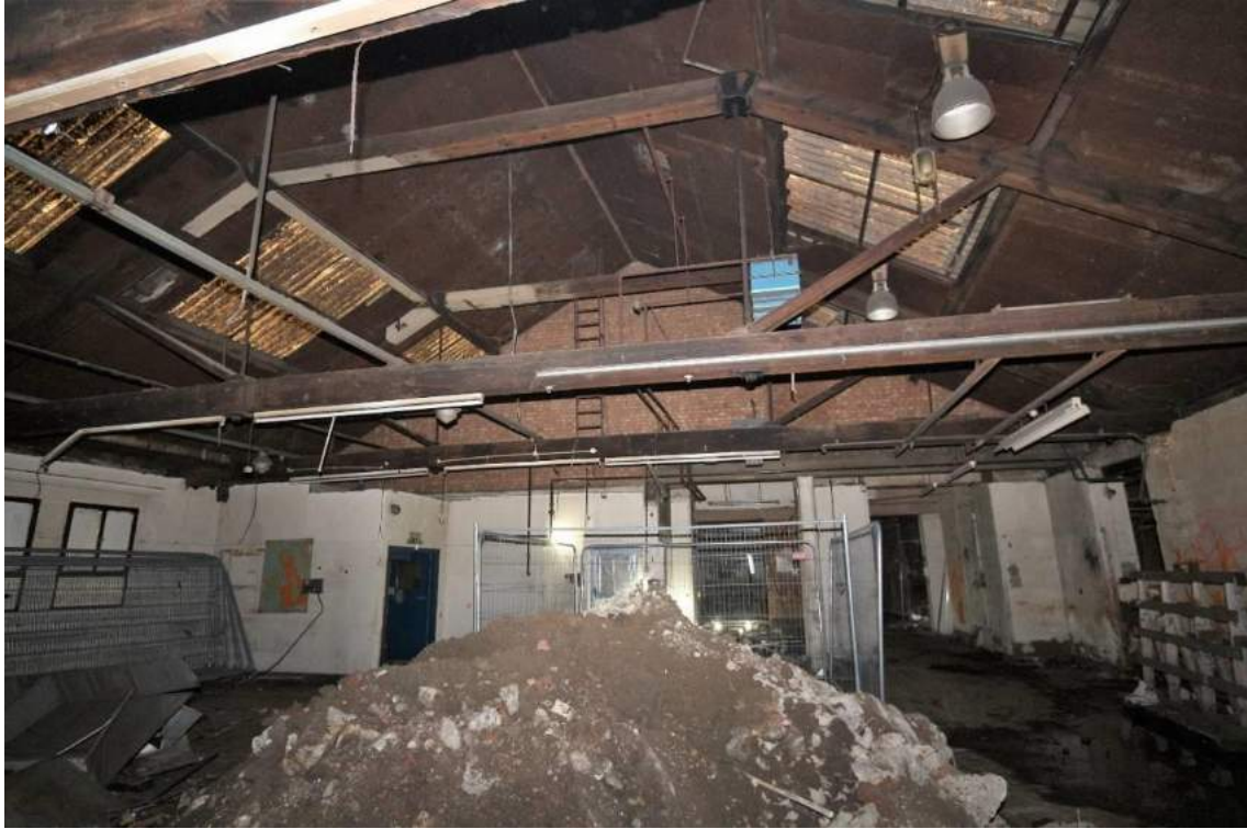
Plate 17 Beam House (B) looking east, showing trusses
