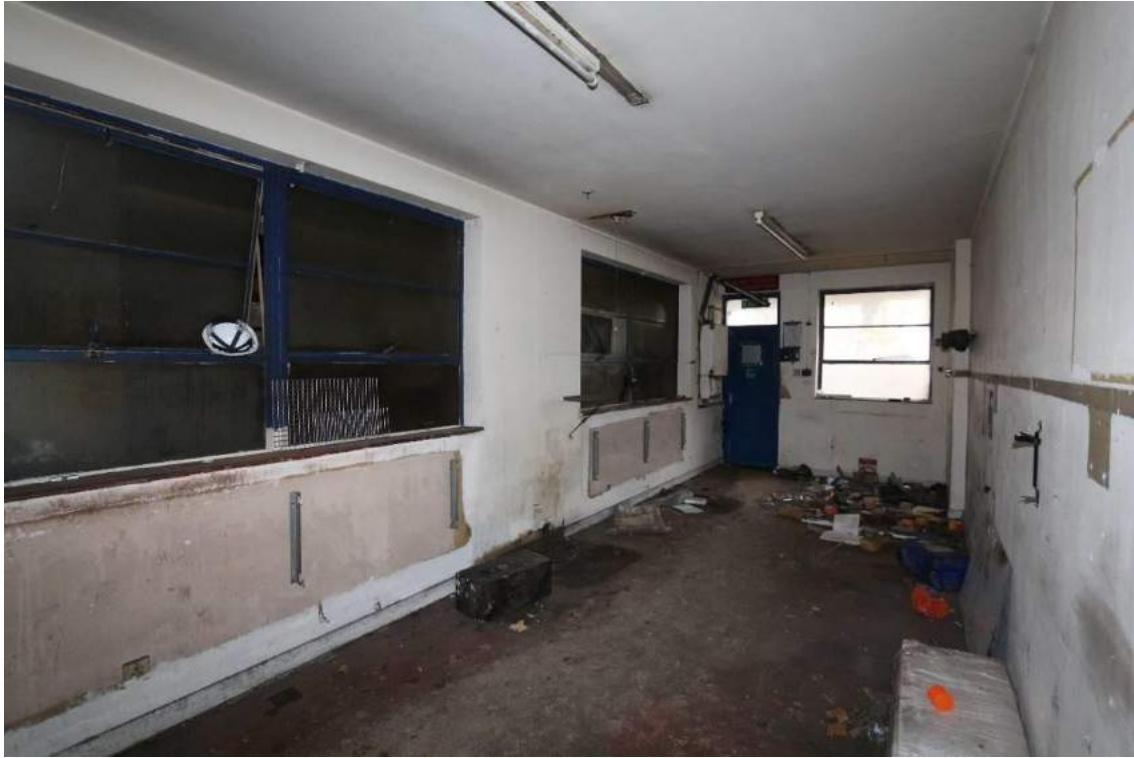
Plate 23 Office in (D1A) looking south
