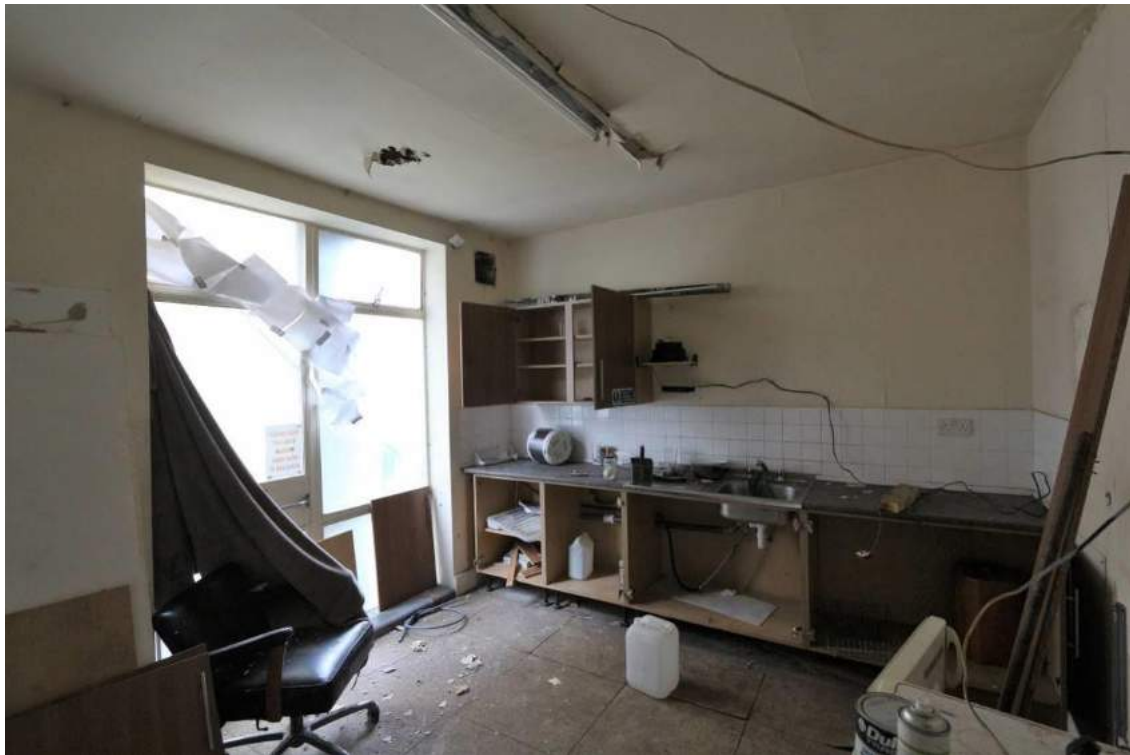
Plate 30 Kitchen (E5) looking south-east
