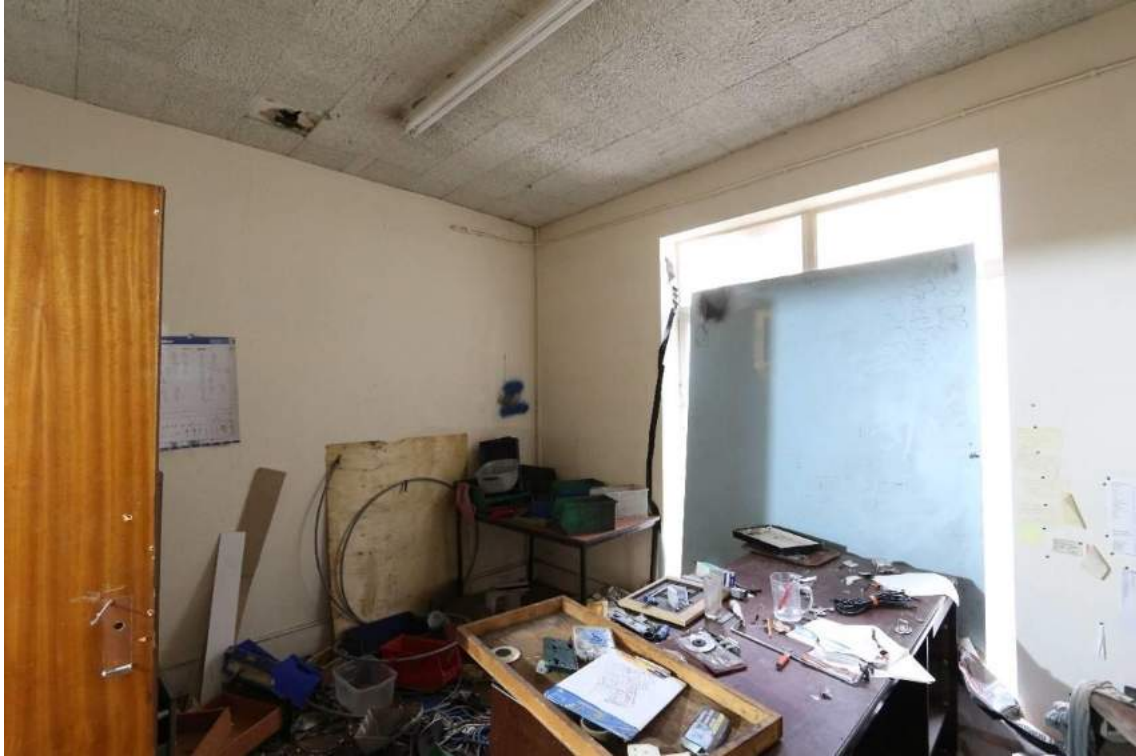
Plate 29 Office (E1) looking north-east
