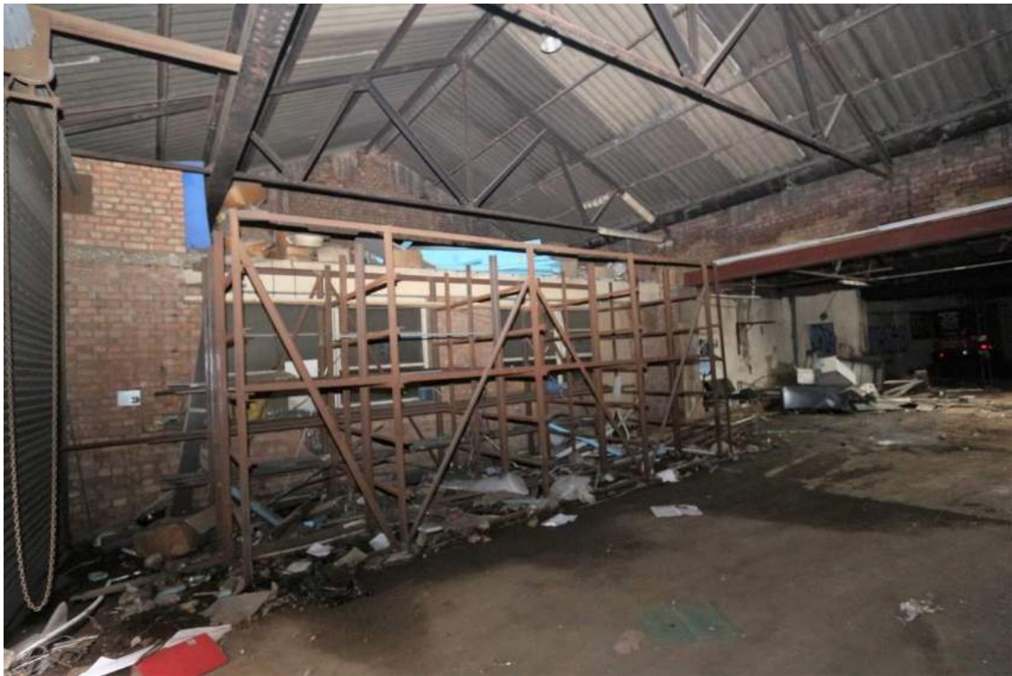
Plate 22 Shed (D) western bays, looking north-west towards office
