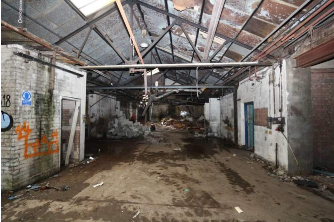
Plate 19 Shed (C), western bays looking east
