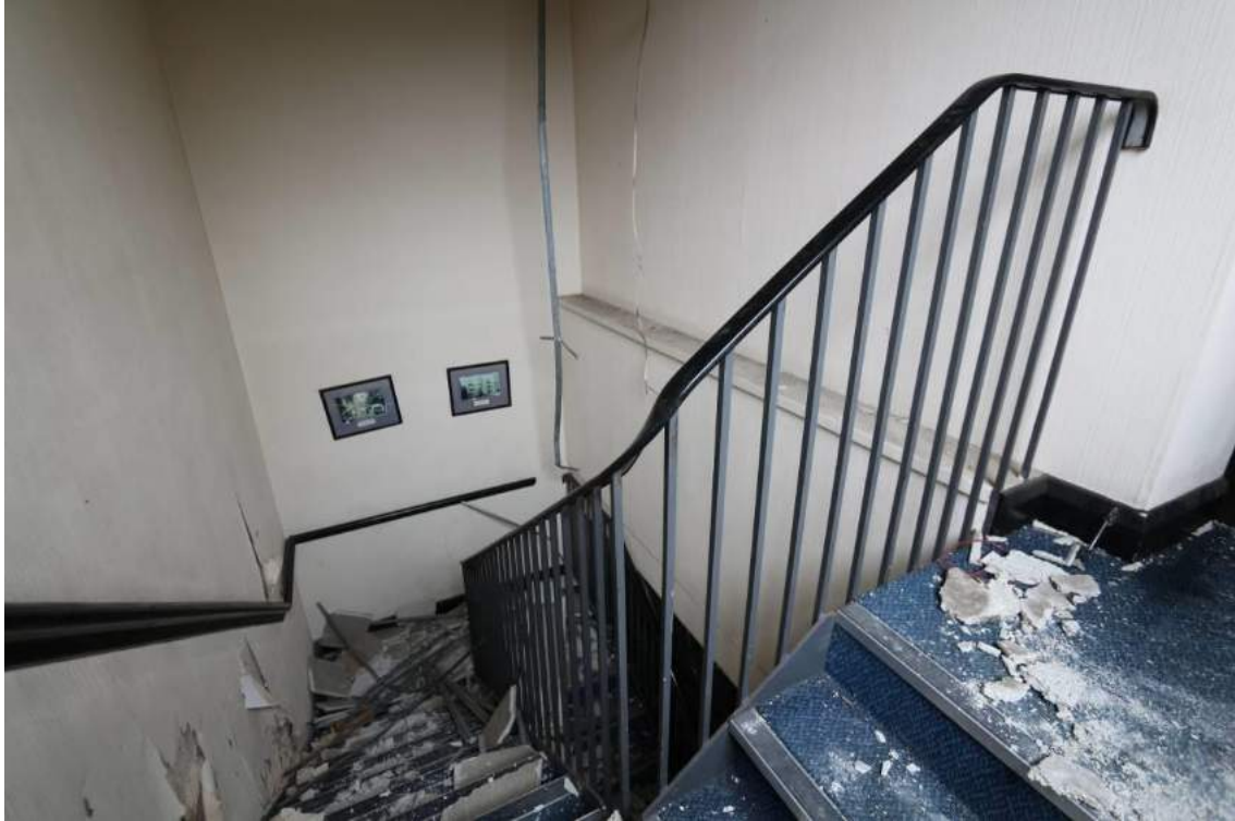
Plate 33 Stair to first floor offices (F)
