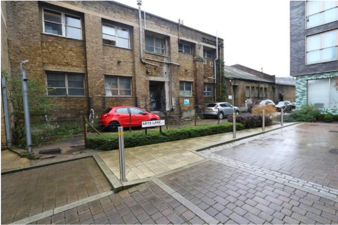
Plate 8 Northern elevations, Beam House (A) and (B), looking south-west
