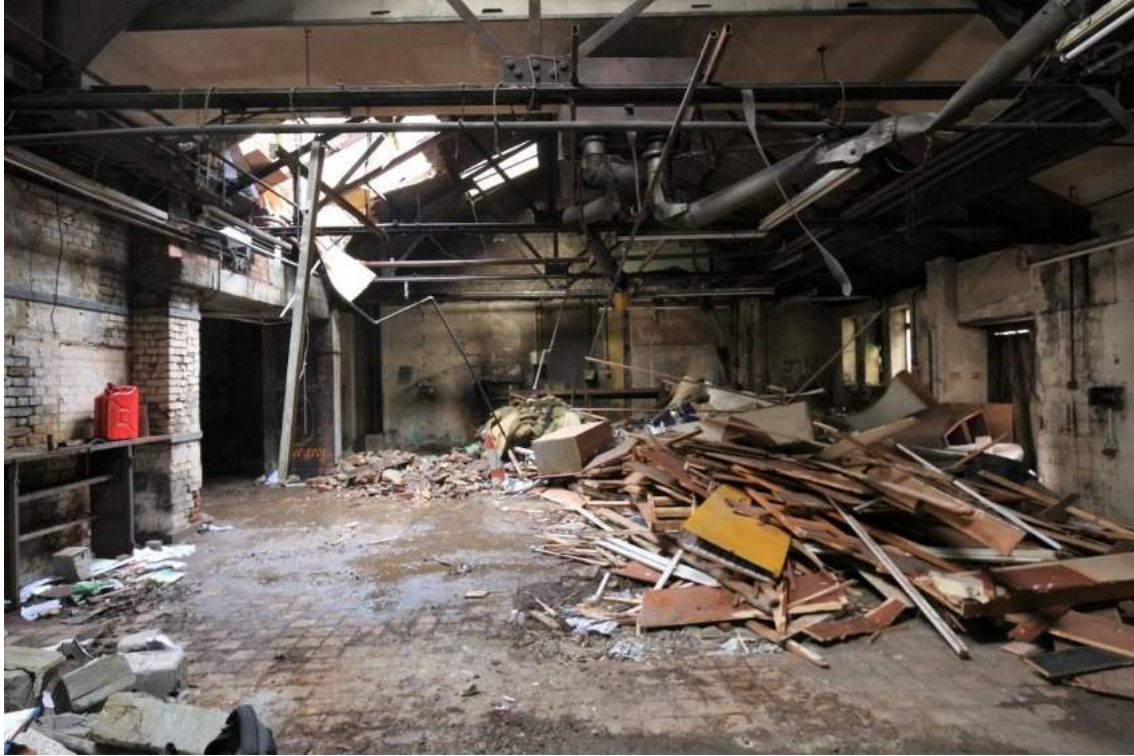
Plate 21 Shed (C), eastern bays looking east
