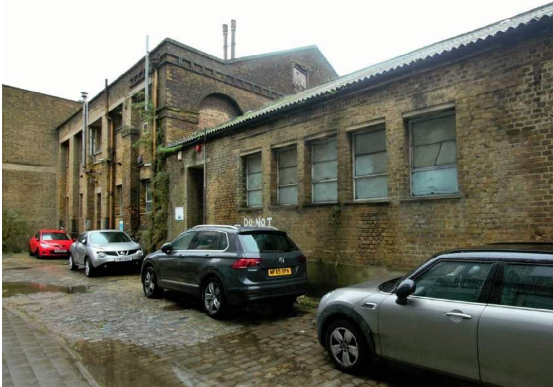
Plate 9 Northern elevations, Beam House (A) and (B), looking south-east
