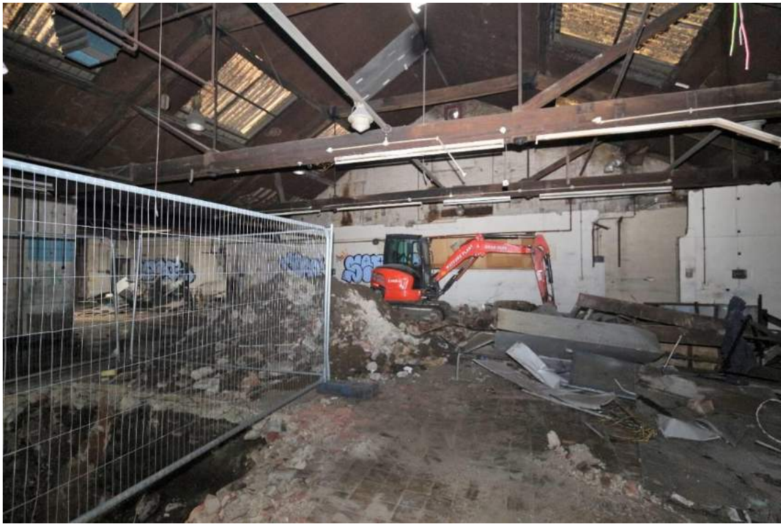
Plate 18 Beam House (B) looking west
