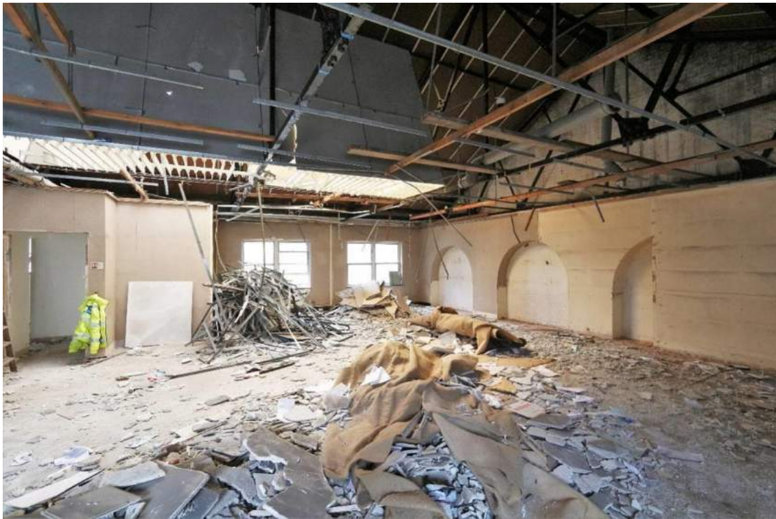
Plate 14 Beam House (AF1), first floor, looking north-east
