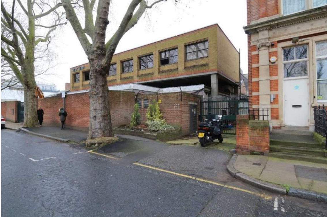
Plate 1 Spa Road site looking north-west
