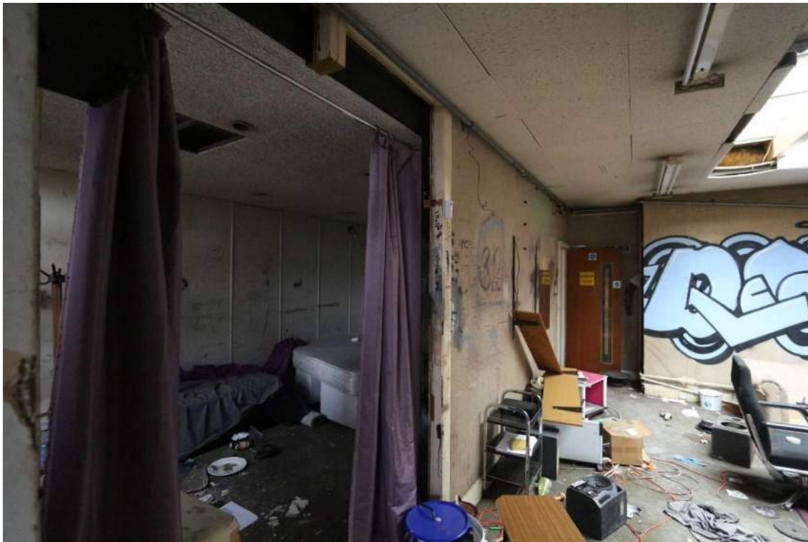
Plate 32 Rooms (E4 and E6) looking east
