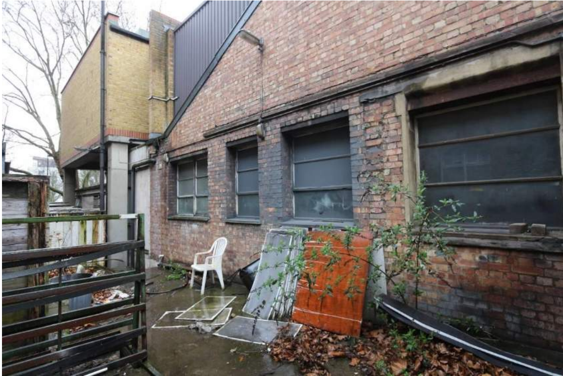
Plate 5 Eastern elevations, Shed (D) and Office range (F) looking south-west
