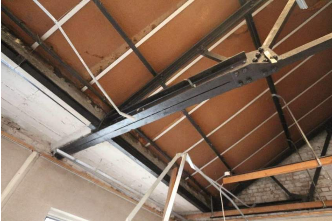
Plate 15 Adapted roof truss, north side, (AF1), looking north-east
