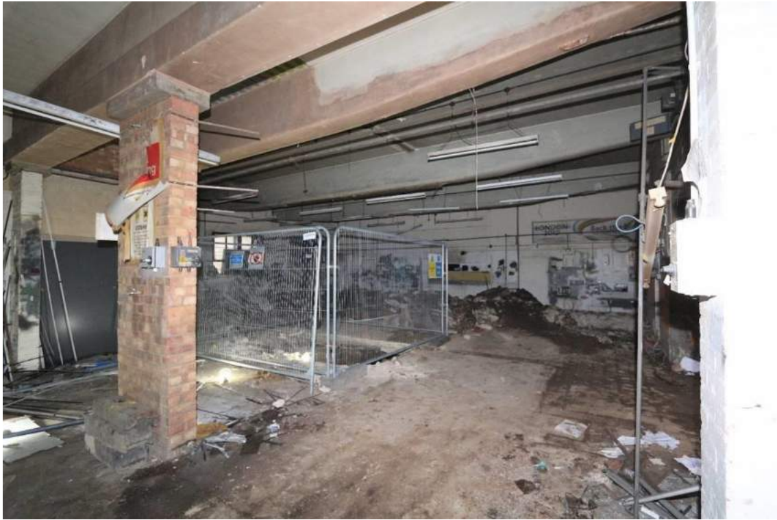
Plate 10 Beam House (A) Ground Floor, looking north-east
