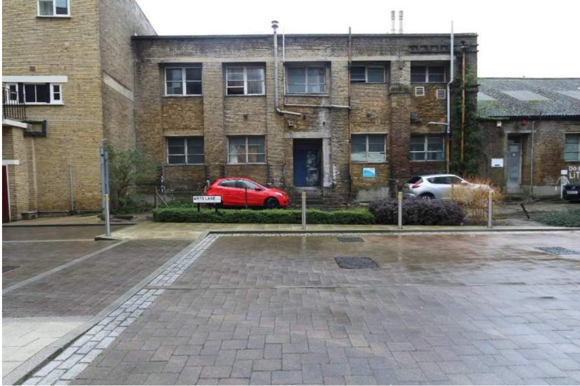
Plate 7 Northern elevations, Beam House (A), looking south
