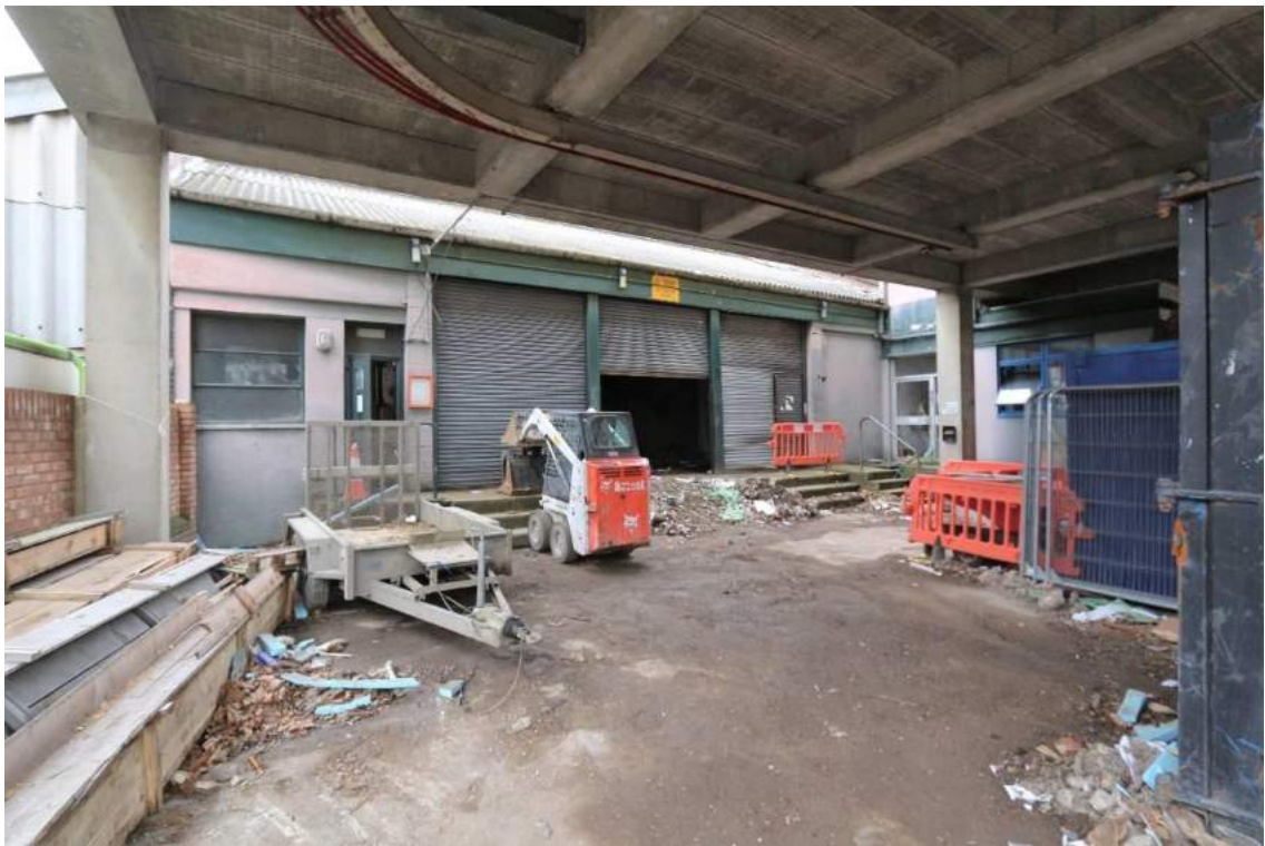
Plate 4 View north-east from front yard area towards southernmost shed (D)
