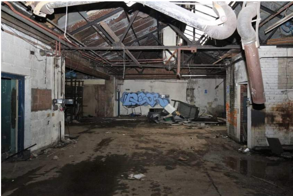
Plate 20 Shed (C), western bays looking west
