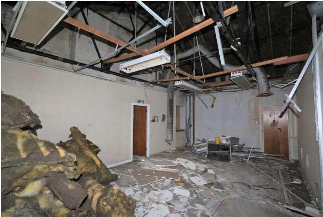
Plate 16 Beam House (AF2) looking north-west towards boiler room and stair
