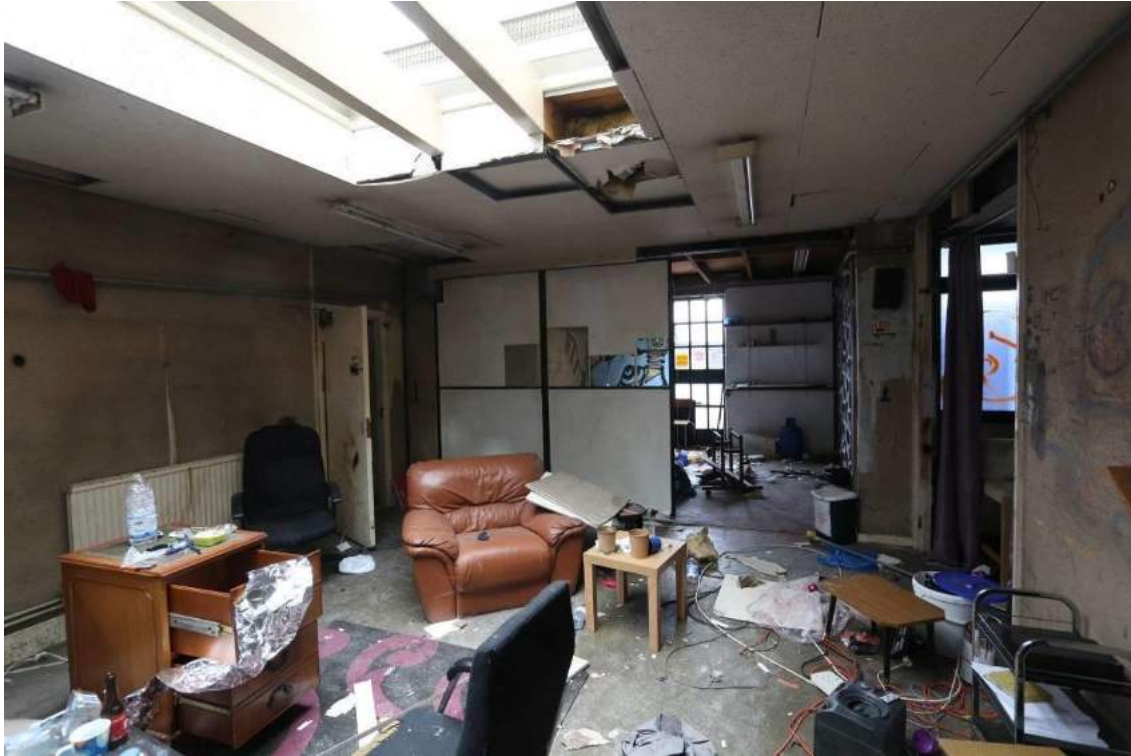
Plate 31 Room (E6) looking south-west
