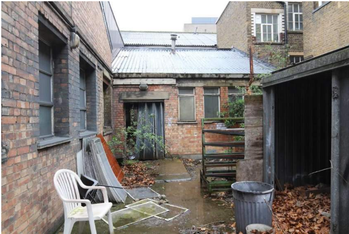
Plate 6 Eastern elevations, Shed (C) looking north
