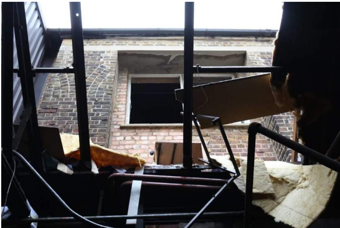
Plate 12 Rebuilt southern elevation (A) at first floor level, looking north
