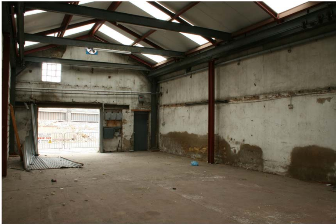
Plate 19 General view of Building 2, central bay, looking west
