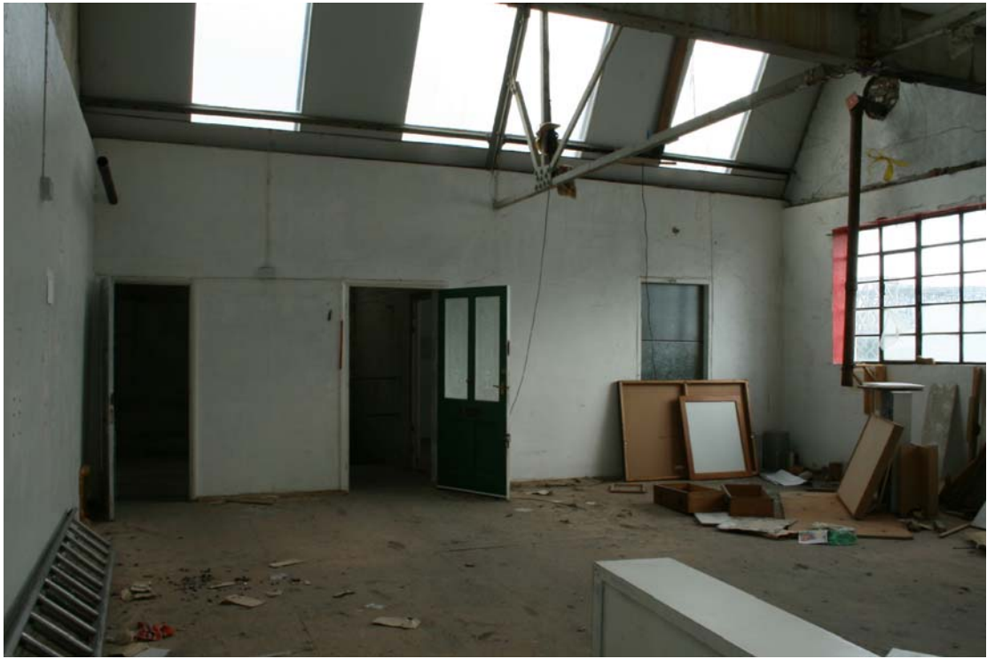
Plate 17 General view of first floor, Building 2
