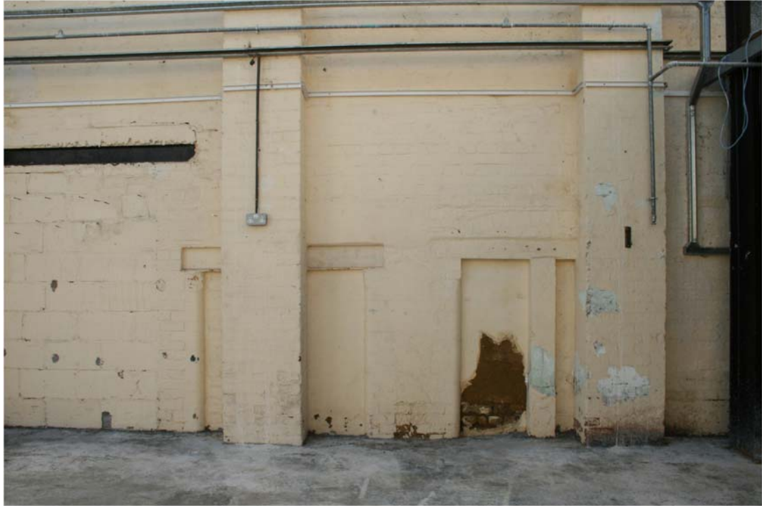
Plate 8 Blockings in south-west wall of Building 1, looking south-west
