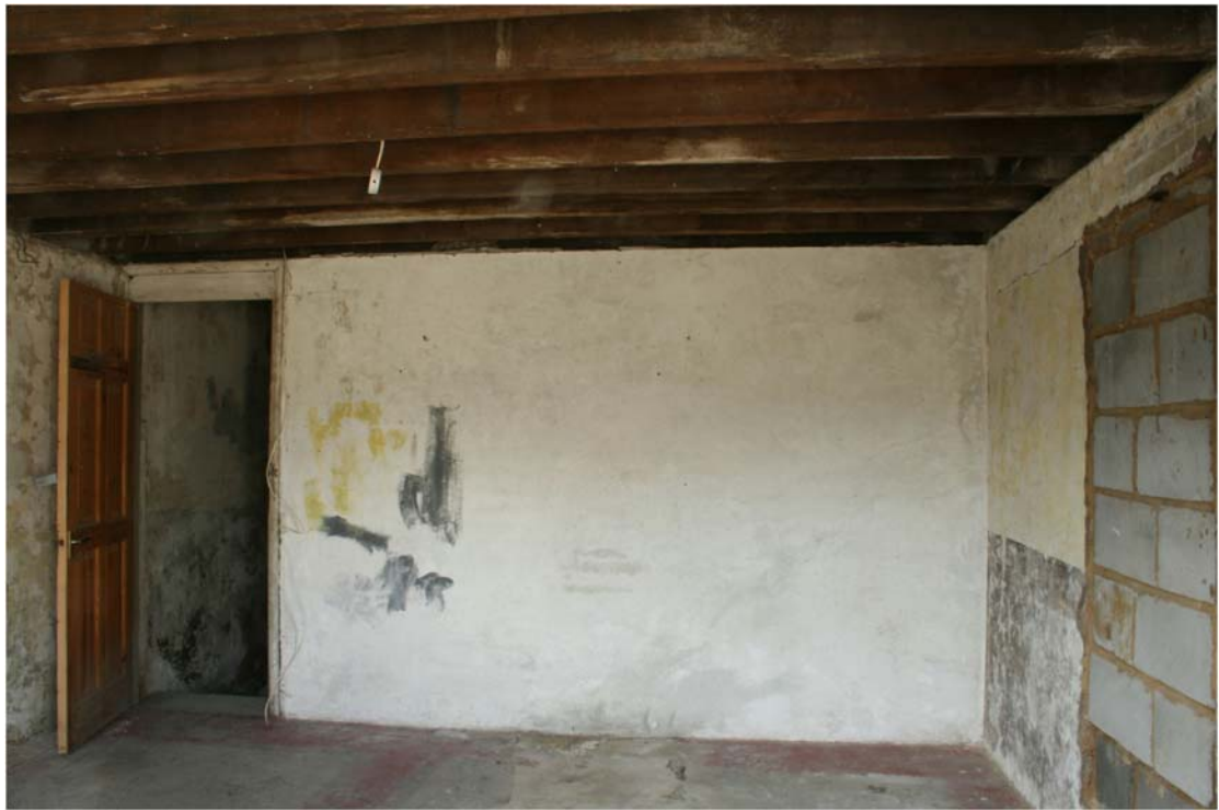
Plate 15 General view of Room 1, Building 2, looking north-west
