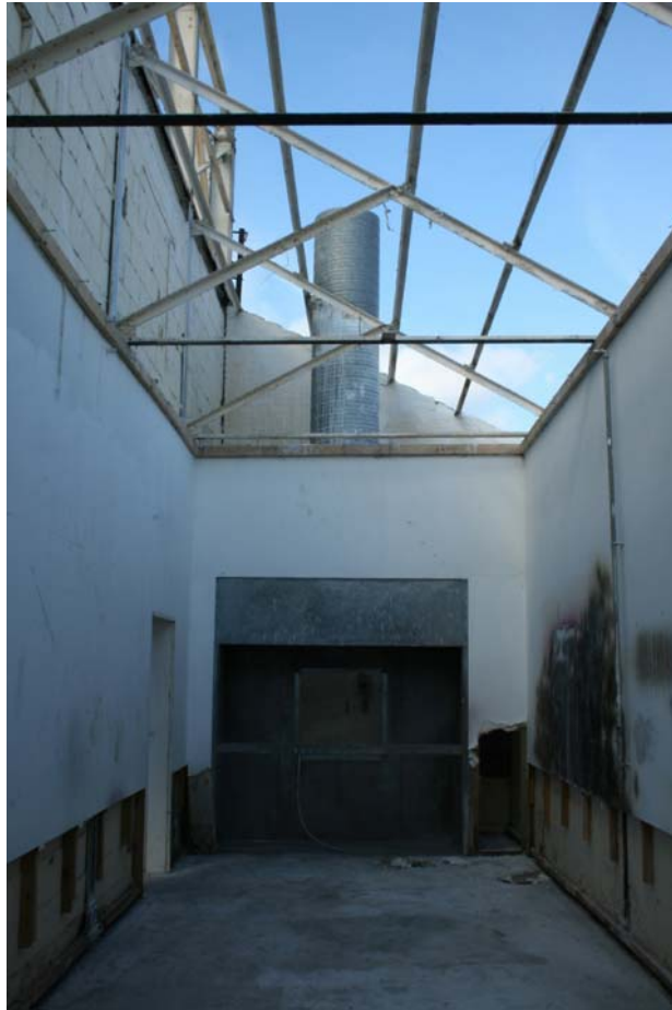
Plate 10 Internal view of Building 1, north-east aisle, looking north-west
