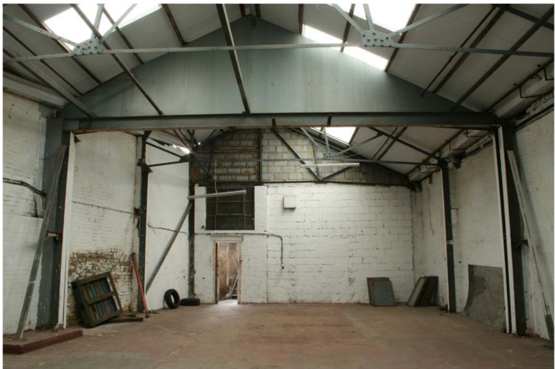
Plate 18 General view of Building 2, north-west bay, looking north-east
