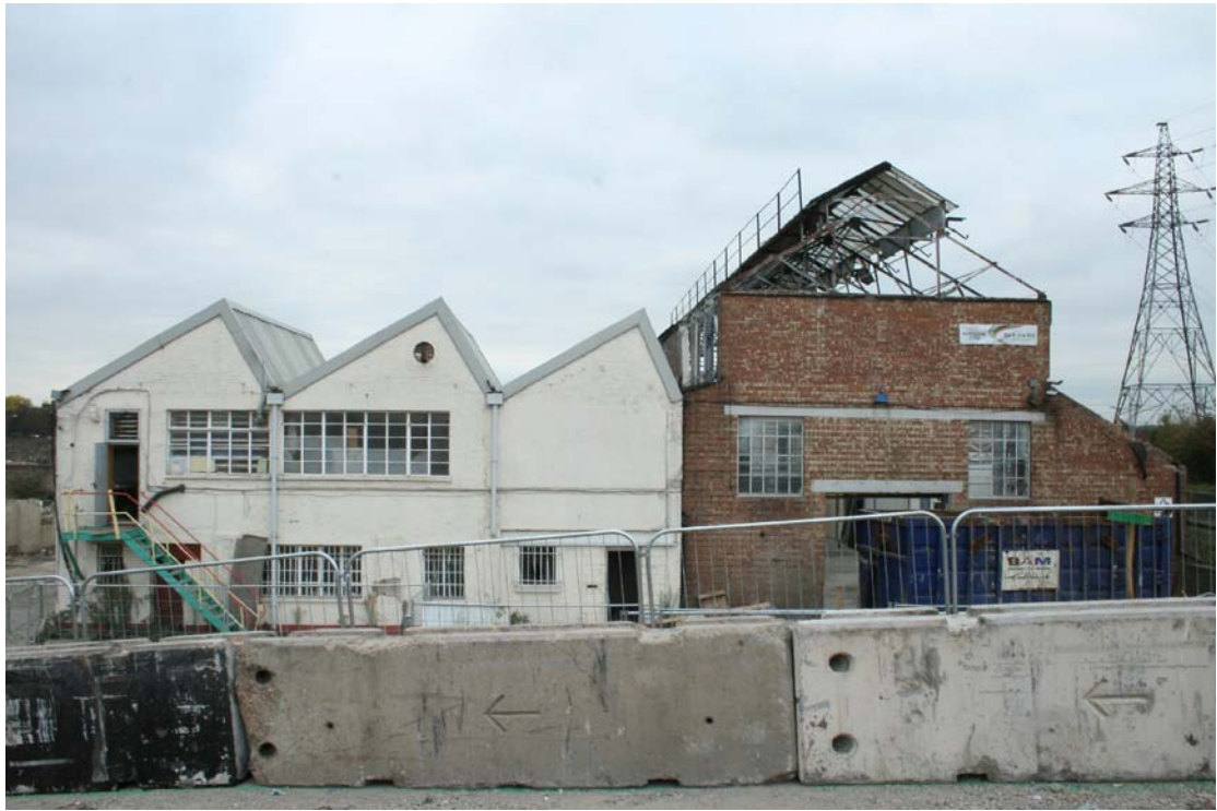
Plate 4 View of Buildings 1 and 2, looking north-west
