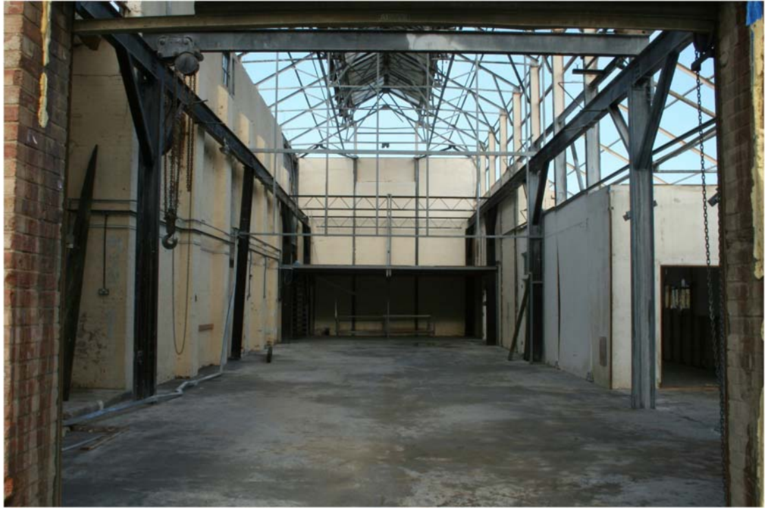
Plate 6 Internal view of Building 1 looking north-west, showing principal space, frame and roof trusses
