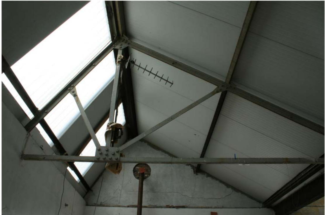
Plate 13 Truss supporting sawtooth-roofed section of Building 2, looking south-east
