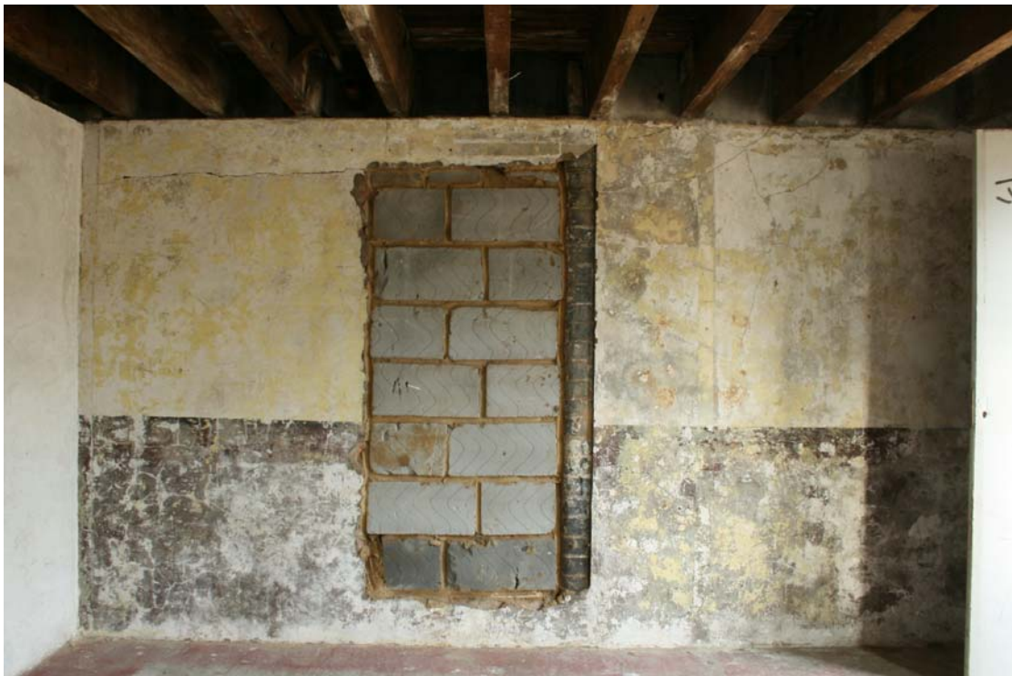
Plate 9 Blocked doorway in north-east wall of Building 2, looking north-east
