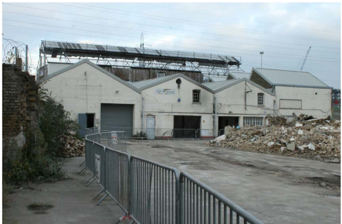
Plate 14 South-west elevation of Building 2, looking east
