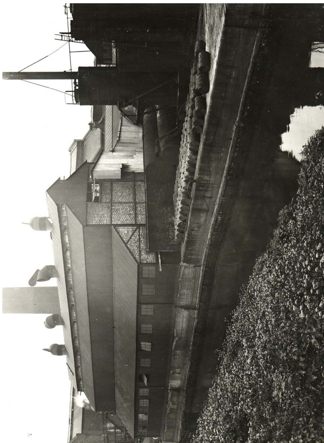
Plate 1 View of Buildings 1 and 2: "T.H. Harris & Son's Works, Marshgate Lane, Stratford- frontage to City Mill River. May 1930", looking south-west
