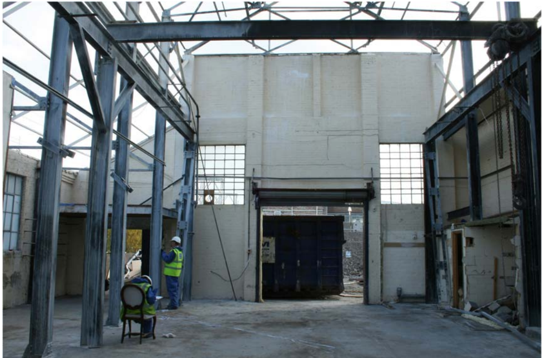
Plate 7 Internal view of Building 1 looking south-east, showing south-east wall and frame
