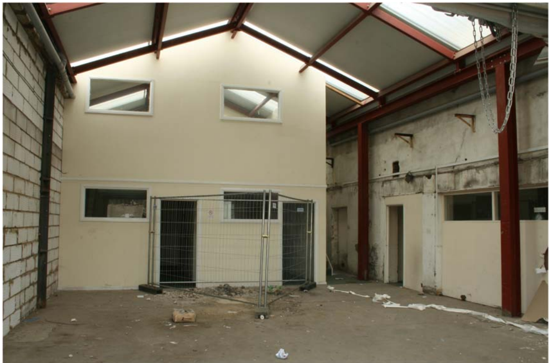
Plate 22 Internal view of south-east bay, Building 2, looking east
