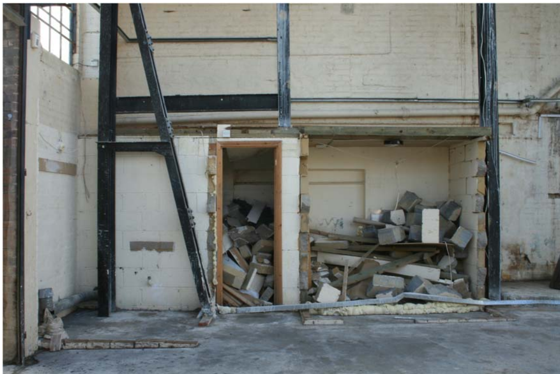
Plate 11 Partially demolished partitioned rooms in south-west corner of Building 1, looking south-west
