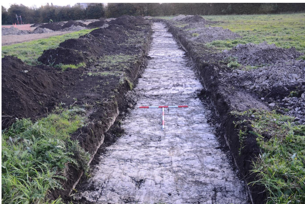
Plate 10: Trench 6, view north
