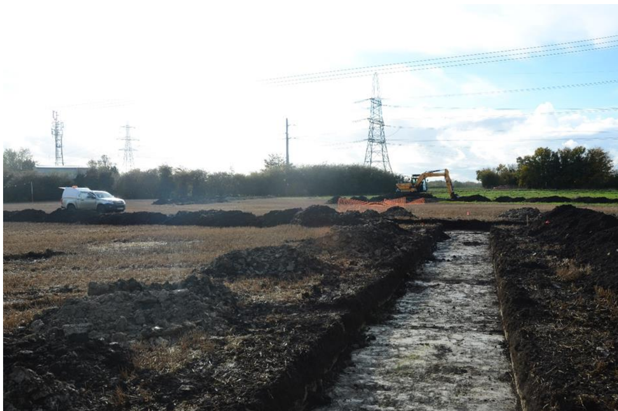
Plate 1: The site, view south-west towards Weirs Drove
