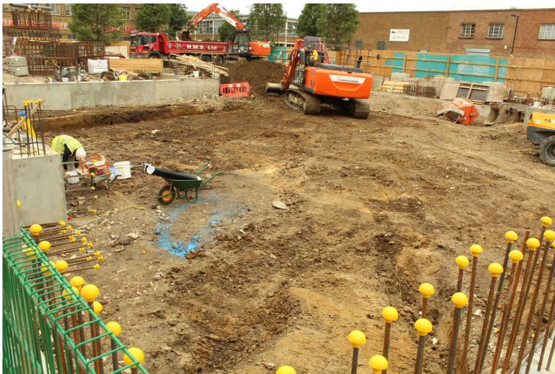
Plate 9: general view of basement area (Trench 3), looking north-west.
