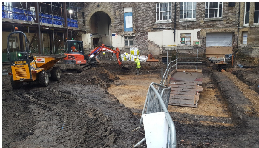
Plate 4: Northern extent of Area 4, facing north
