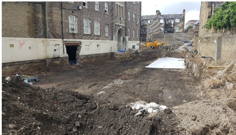
Plate 2: Area 1, facing west
