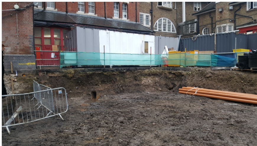
Plate 5: Southeastern end of Area 4, facing southeast
