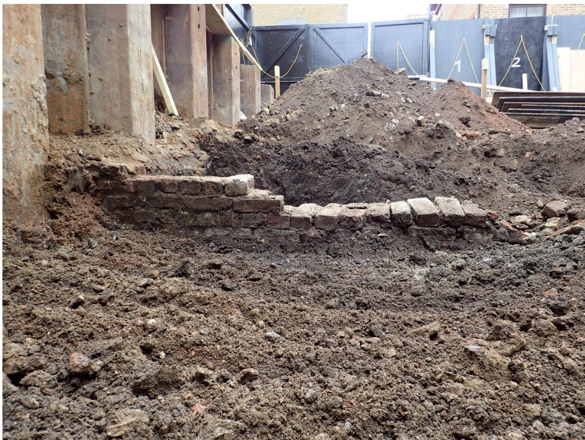
Plate 6: Brick lined pit. Looking southeast.
