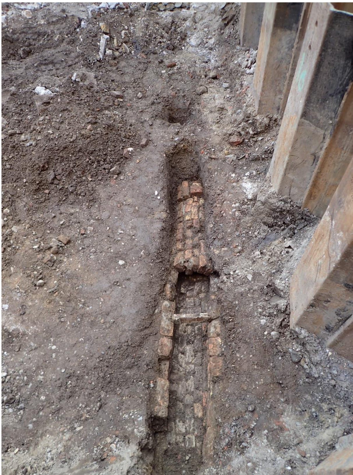
Plate 8: Brick lined culvert. Looking southwest.
