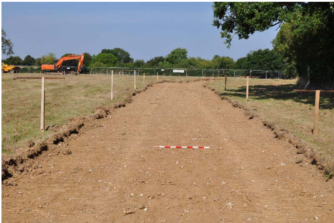
Plate 2. A section of the access drive, taken looking northwest.
