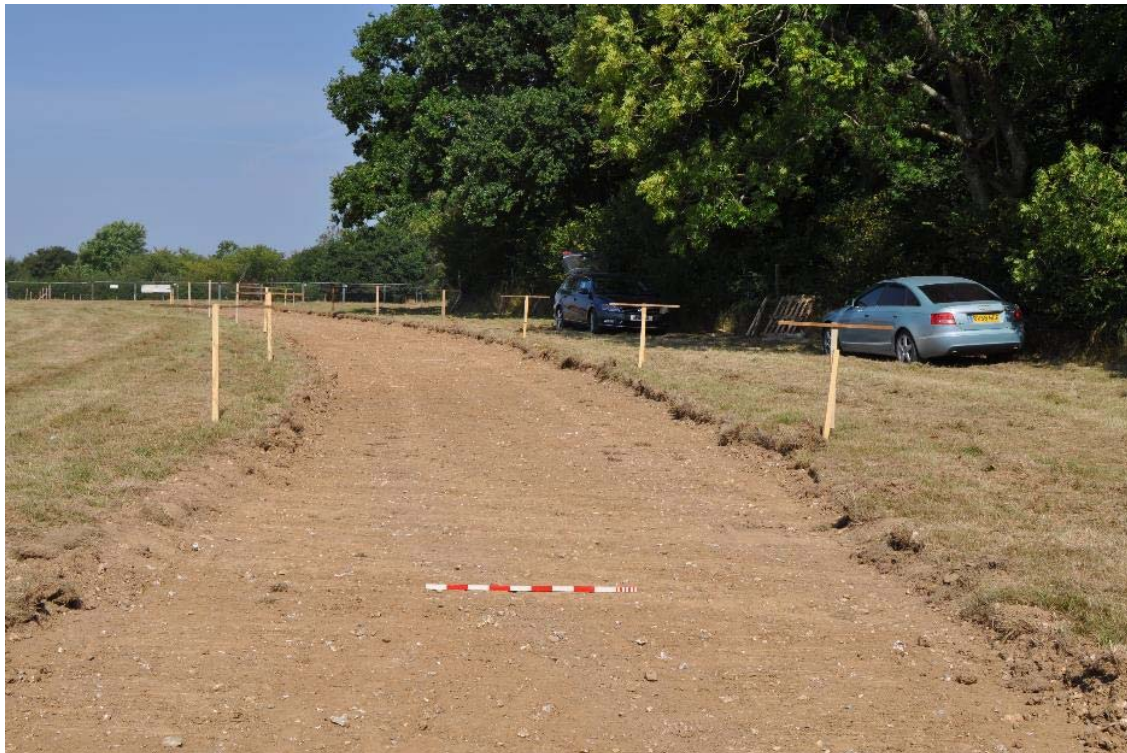
Plate 1. A section of the access drive strip, taken looking northwest.
