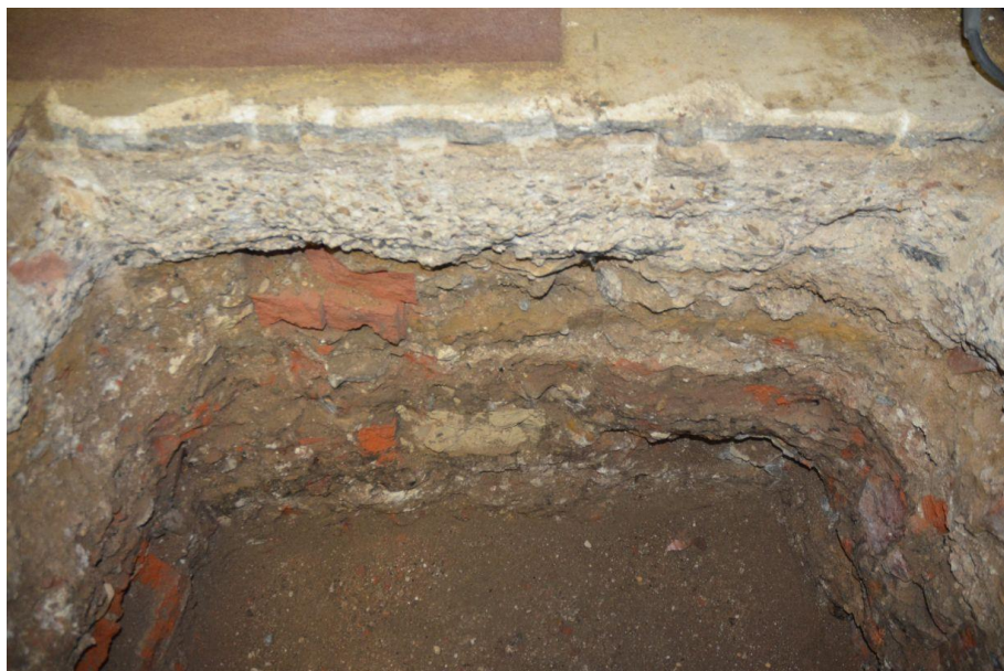
Plate 7: Pad foundation fully excavated. Layer (113) in base.
