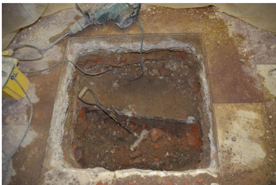
Plate 6: Pad foundation under excavation
