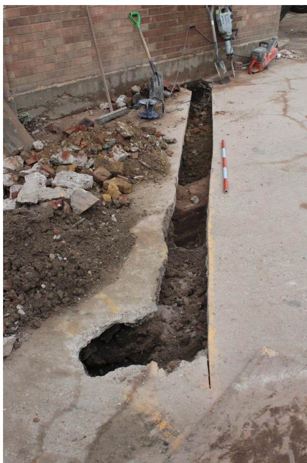
Plate 8: Service trench in courtyard
