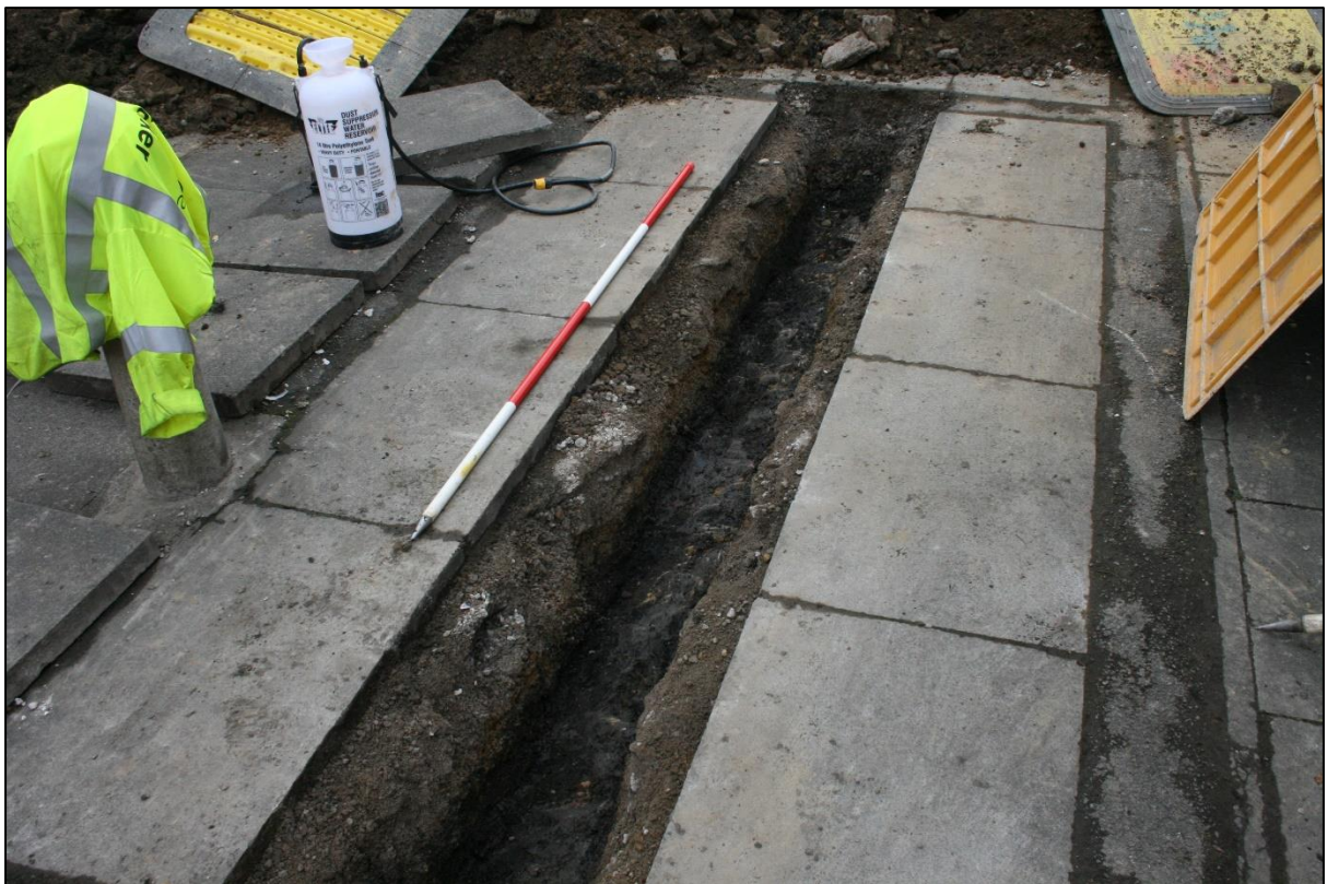
Plate 4: Trench 5 showing sandstone rubble deposit (504), direction of view South, scale: 1m.
