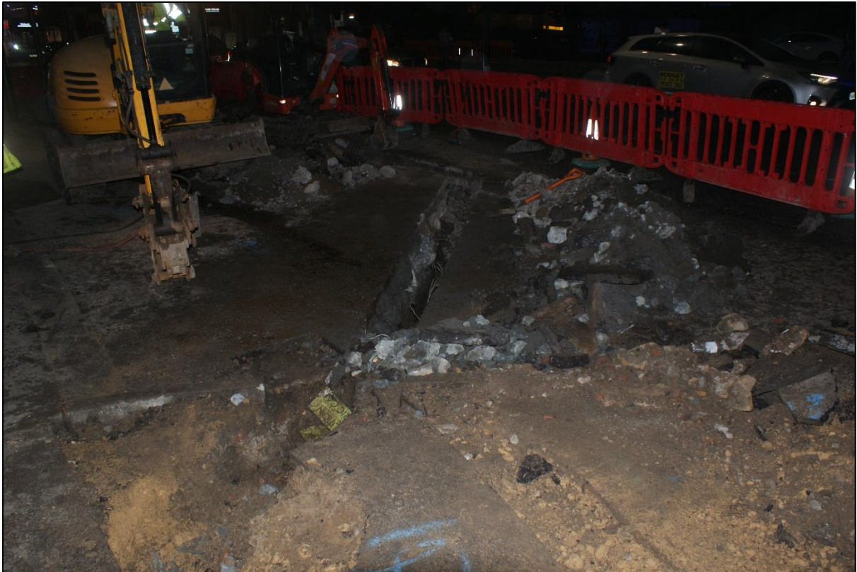
Plate 3: Trench 3, direction of view NW.
