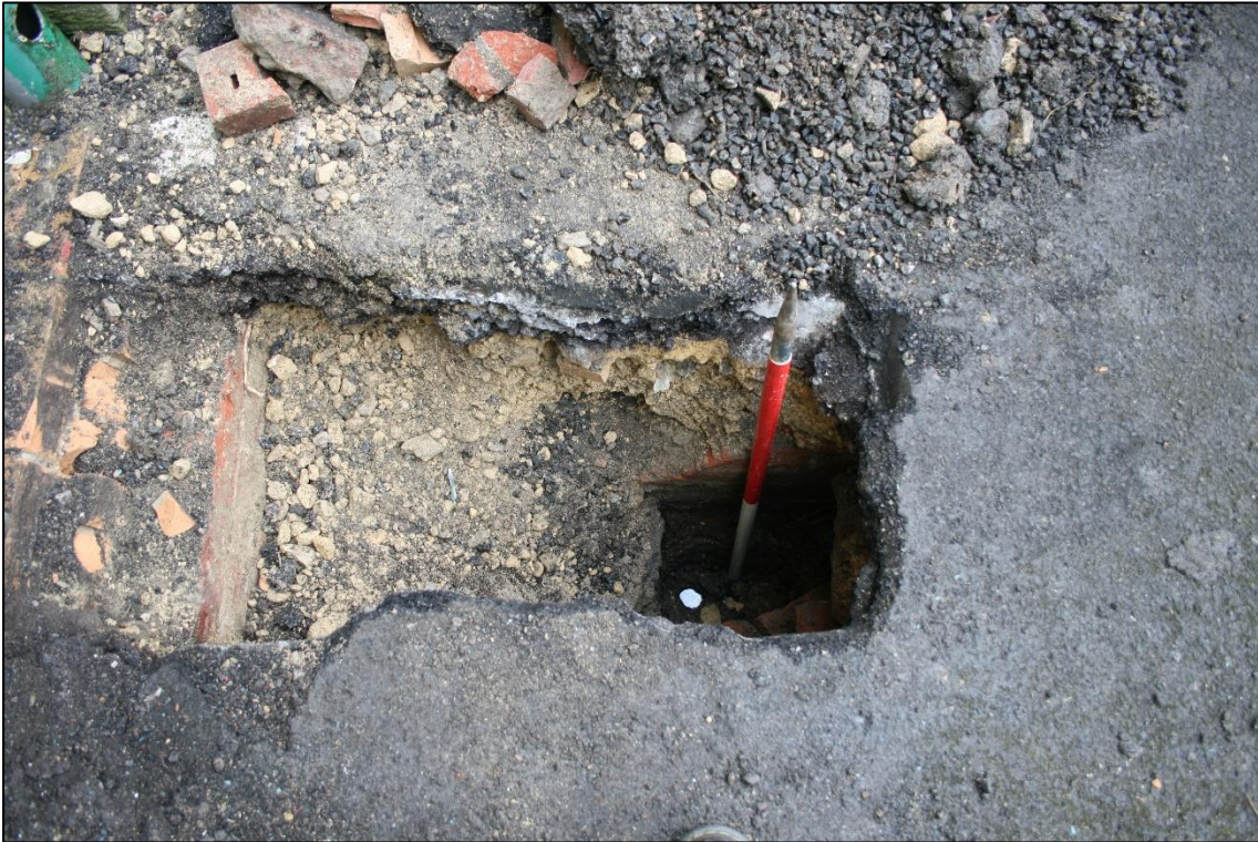
Plate 1- Test Pit 01 showing walls [006] and [010]. Facing southwest, 1m scale.
