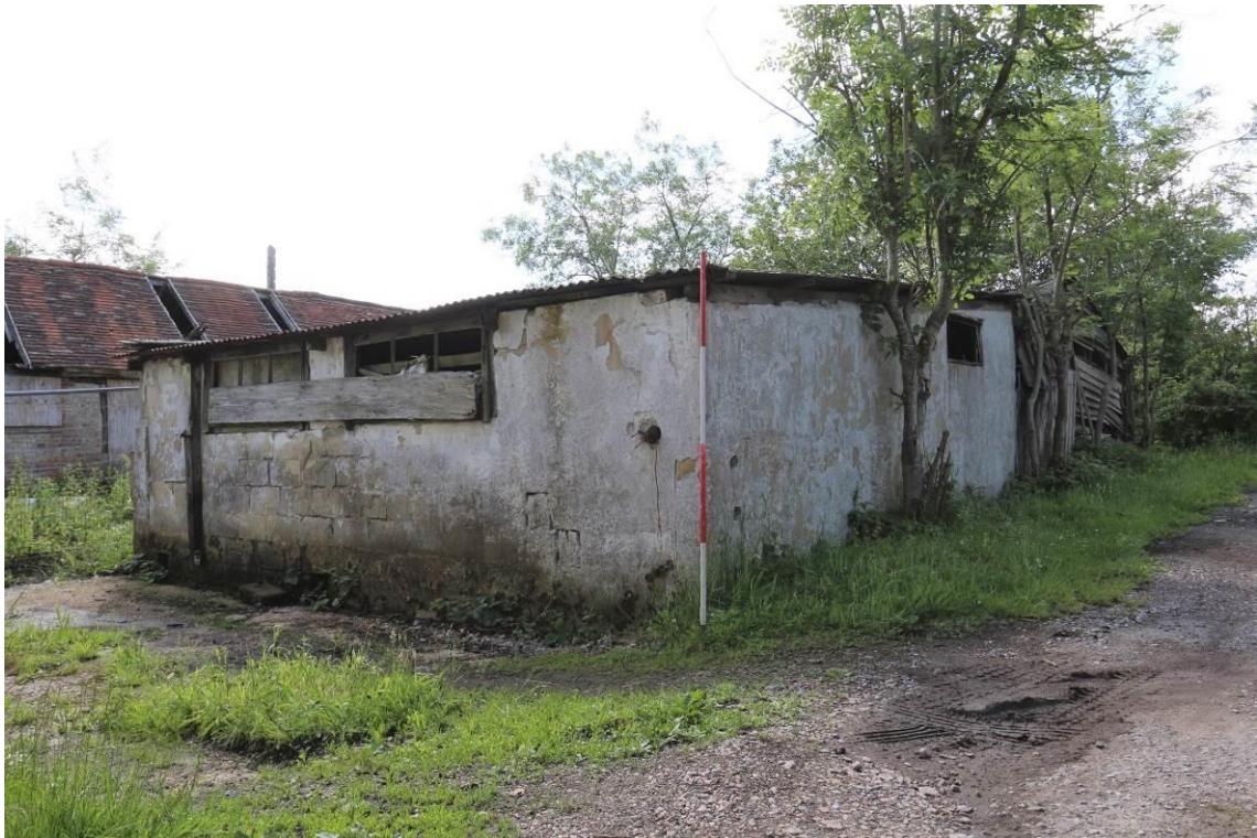
Plate 9 Building 2, looking south-east
