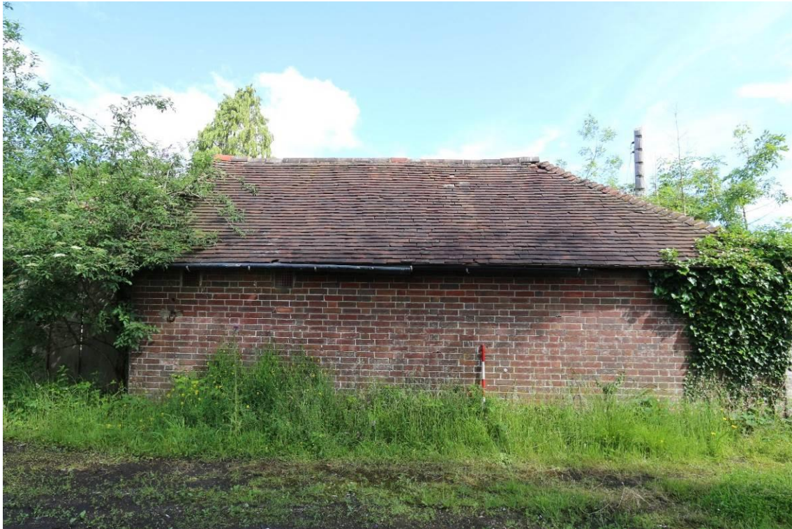
Plate 1 Building 1 southern elevation, looking north
