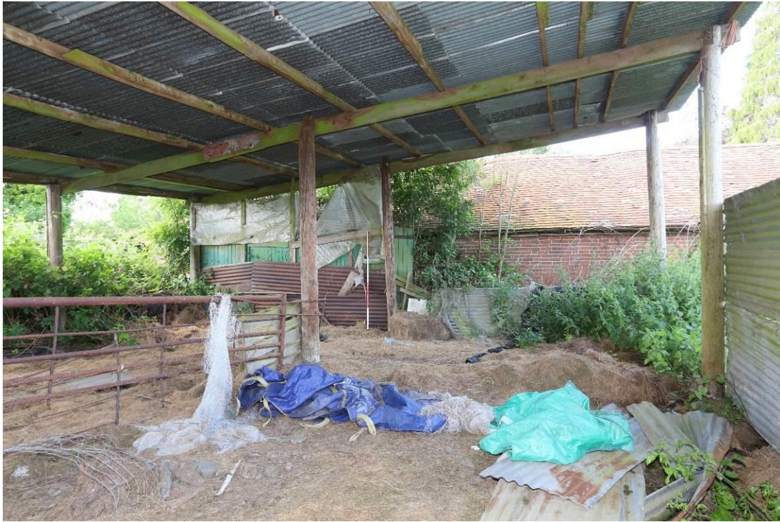
Plate 14 Building 3, Pole Barn, looking south-west
