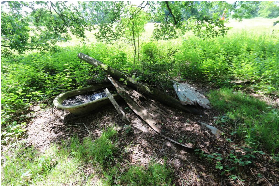
Plate 21 Remains of Building B, looking south
