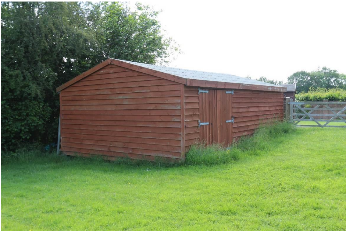
Plate 17 Building 5, looking south-east
