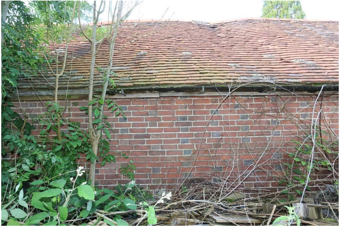
Plate 6 Building 1, eastern return, looking west
