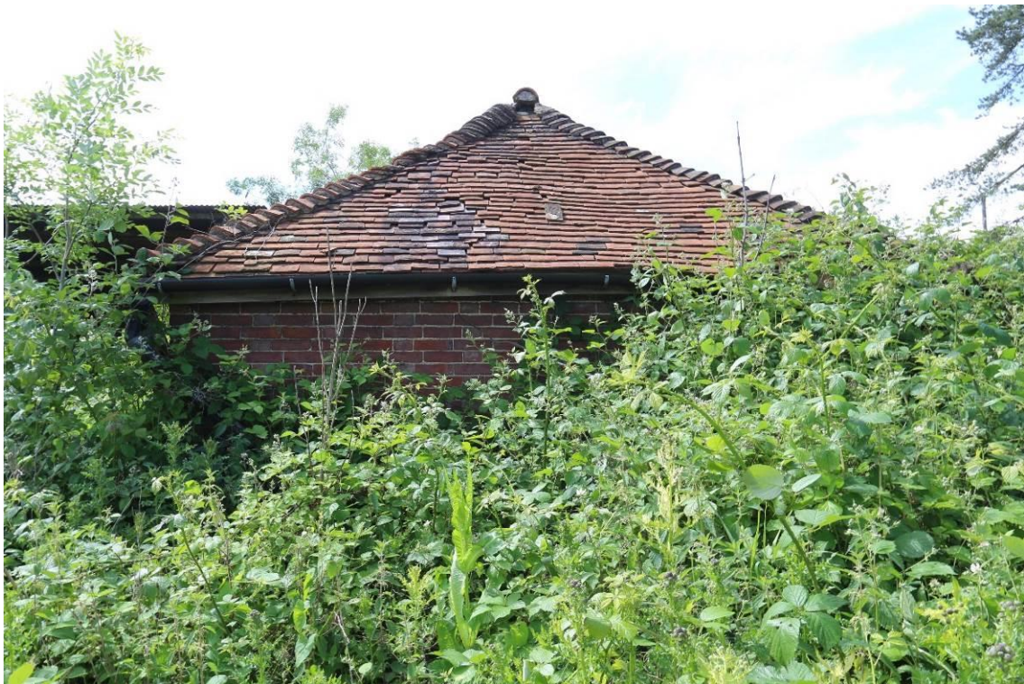
Plate 2 Building 1 northern elevation, looking south
