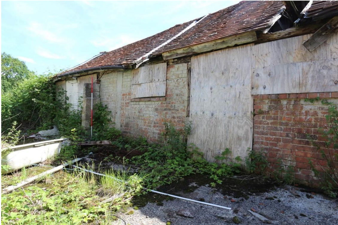
Plate 3 Building 1 Western elevation, looking north-east
