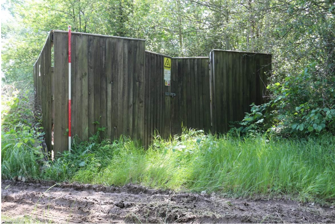
Plate 20 Building 7 Electricity Sub-station, looking east
