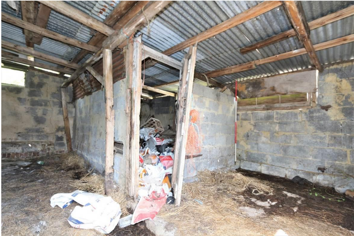
Plate 10 Building 2, northern bays, looking north-west
