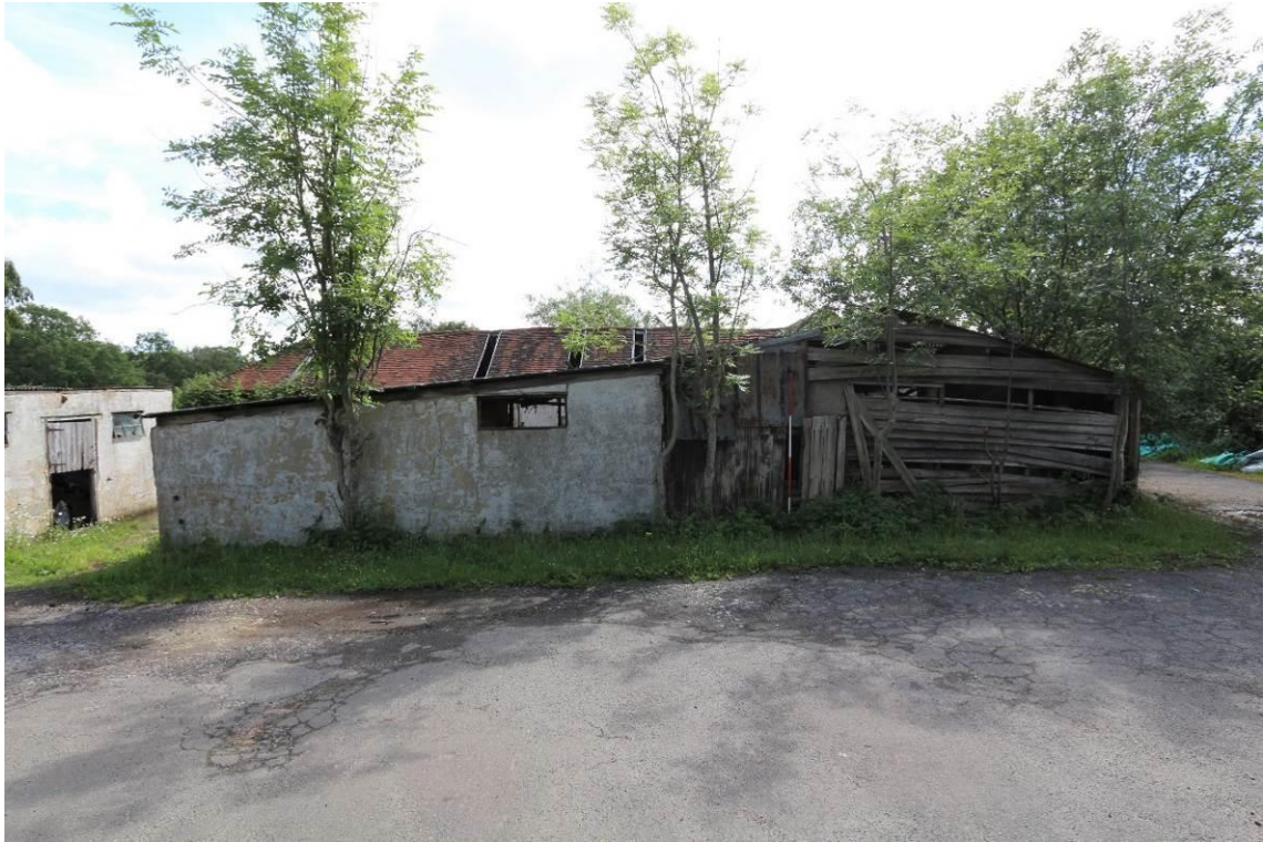
Plate 8 Building 2, looking east
