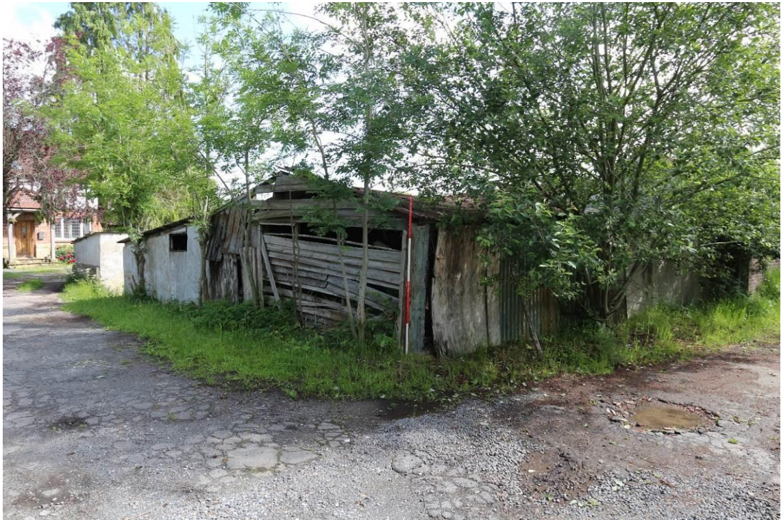
Plate 7 Building 2, looking north-east
