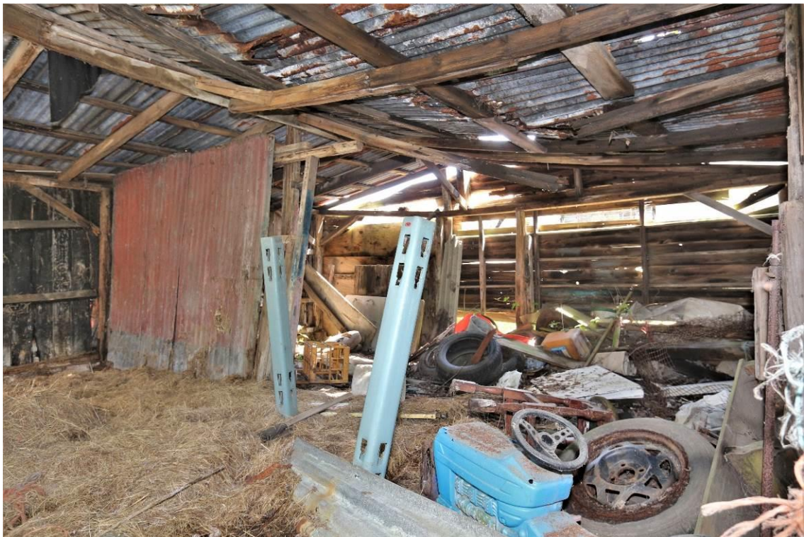
Plate 11 Building 2, southern bays, looking east
