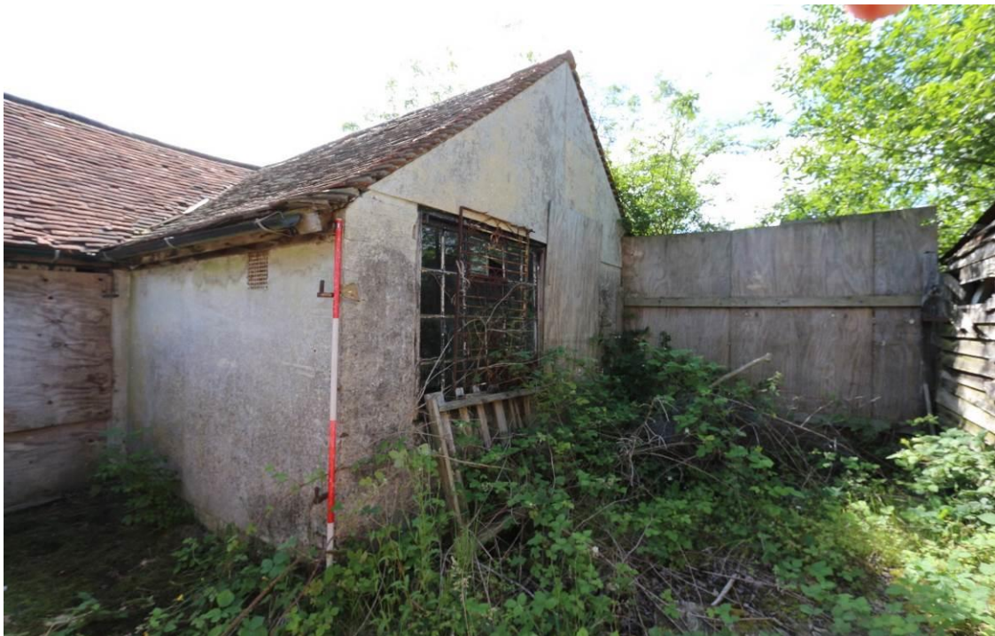
Plate 4 Building 1, southern return, looking south-east
