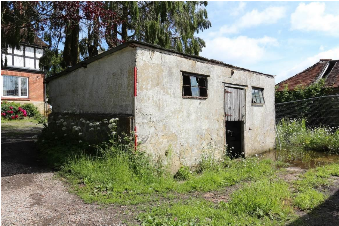
Plate 15 Building 4, looking north-east
