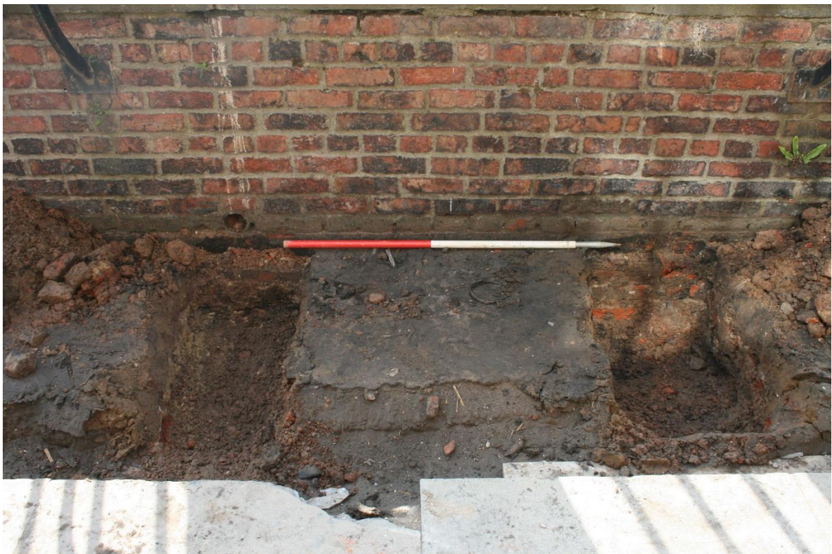
Plate 4: Trench 3 view of short service trench runs, facing WSW, 1m scale.
