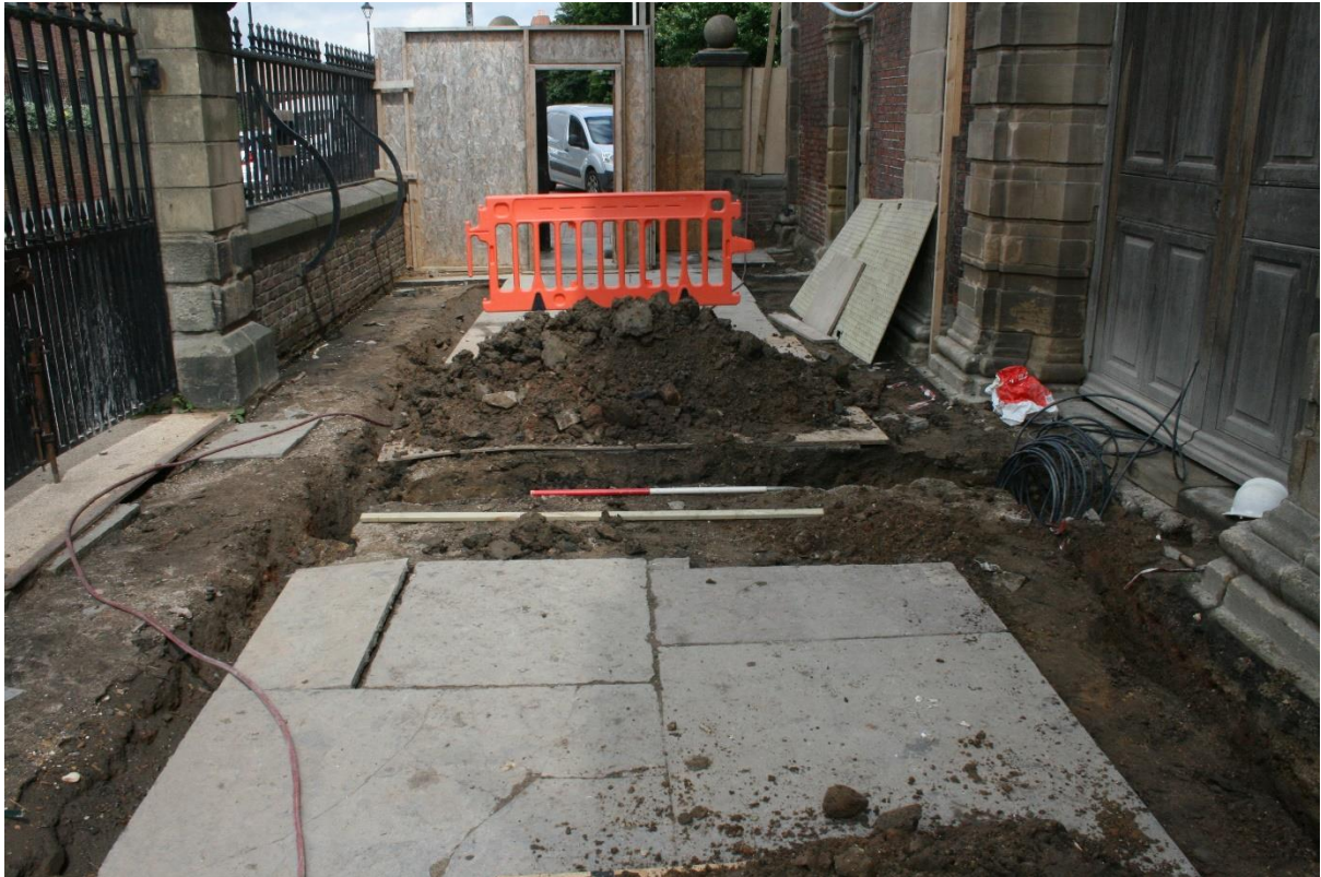
Plate 3: Trench 3 view of service trench runs, facing NNW, 1m scale.
