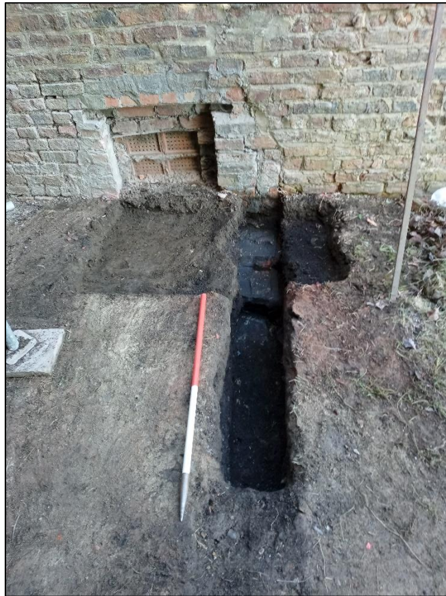
Plate 1: Trench 1 View of wall [152], facing NNW, 1m scale.
