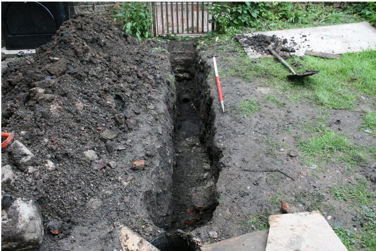
Plate 2: Trench 2 view of service trench run, facing NNW, 1m scale.
