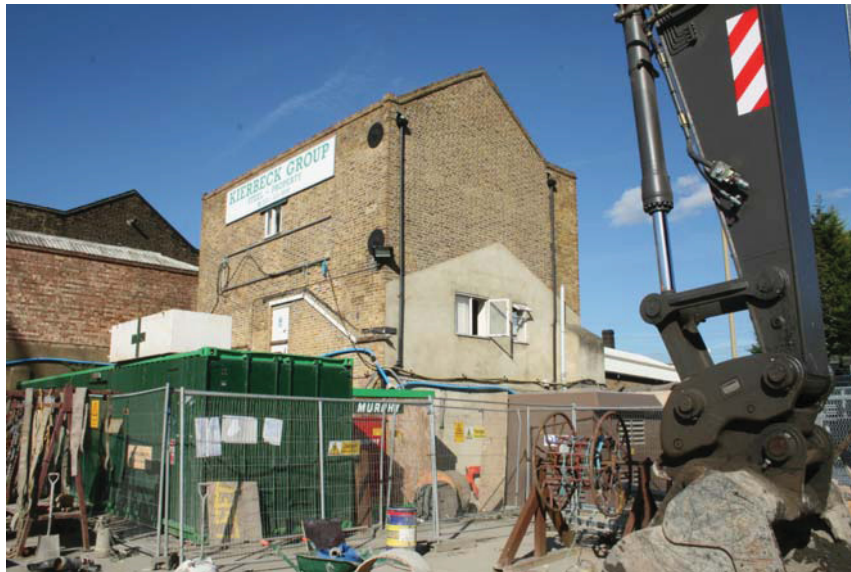
Plate 4 View of rear of Building 1, looking north-northeast
