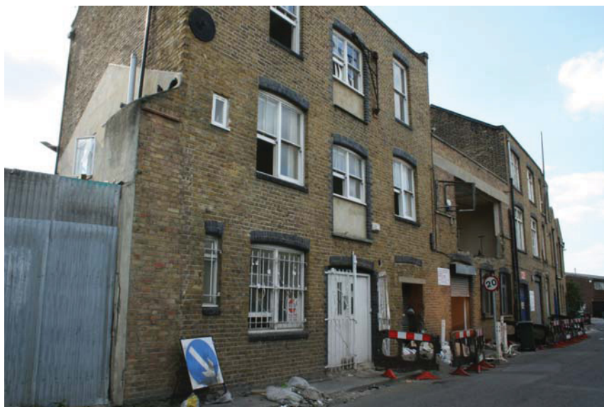
Plate 2 View of Building 1 in foreground and Buildings 2, 3 and 4 in background, looking north-west
