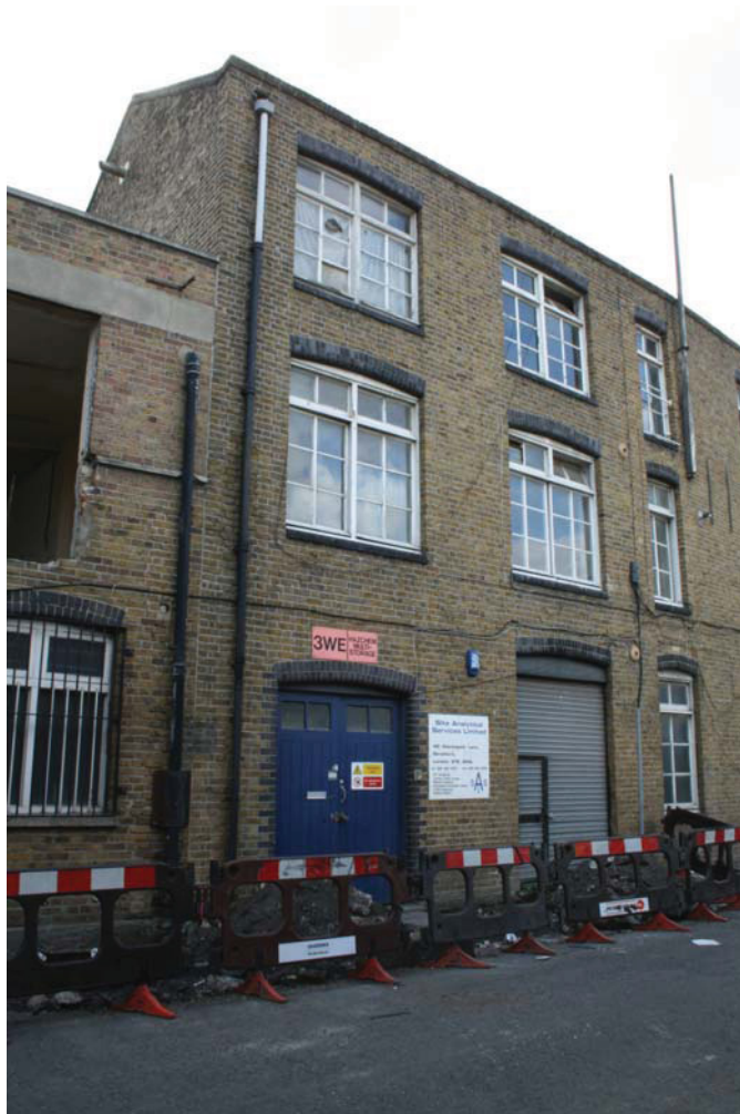
Plate 13 View of Building 3, looking north-west
