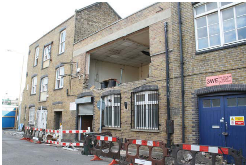
Plate 8 View of Building 2 in foreground and Building 1 in background, looking south-east
