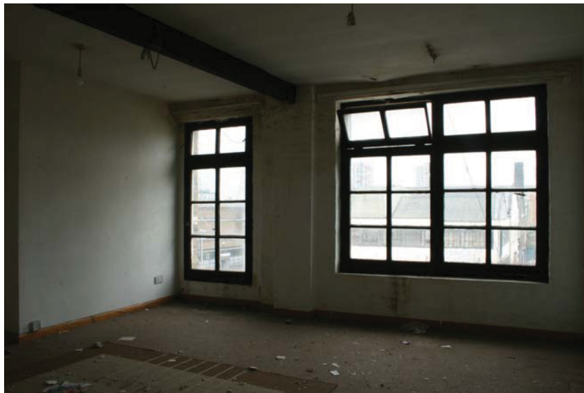
Plate 16 Internal view of Building 3, showing general layout of second floor rooms with original timber beams
