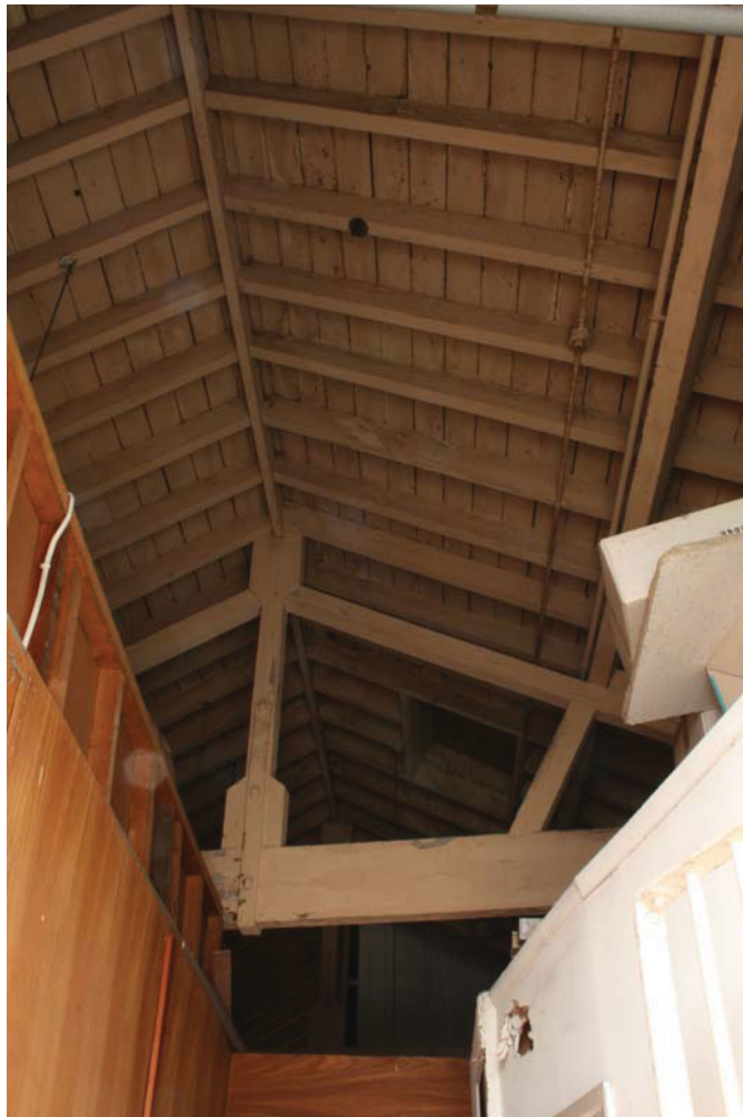
Plate 20 Internal view of Building 4, showing king-post roof truss, looking north-east
