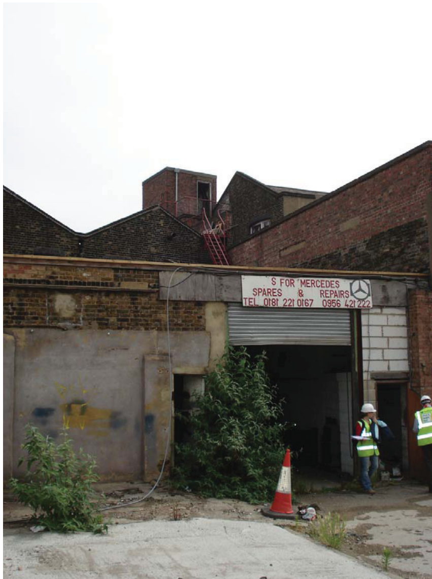
Plate 21 View of Building 5, looking east
