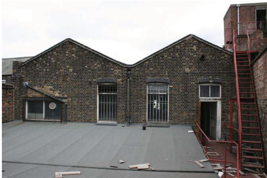
Plate 18 View of rear of Building 4 and roof of Building 5, looking north-east
