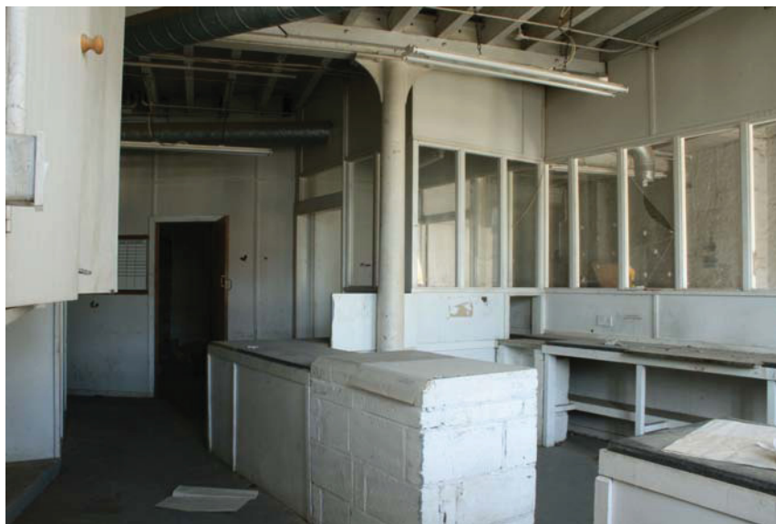
Plate 19 Internal view of Building 4, showing general layout and partitioning, looking south-west
