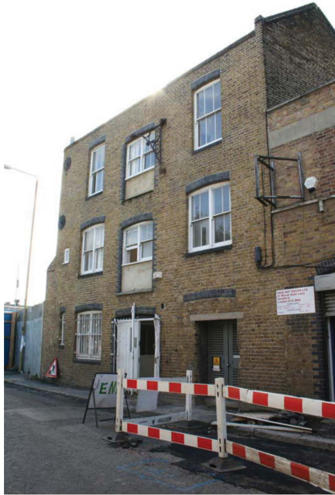
Plate 3 View of Building 1, looking south
