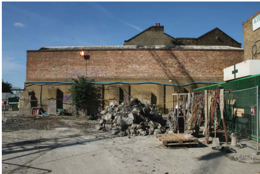
Plate 9 View of the south-east elevation of Building 2, looking north-west
