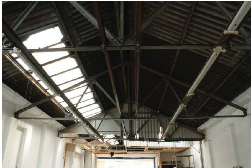
Plate 12 Internal view of Building 2, showing fink truss, looking north-east
