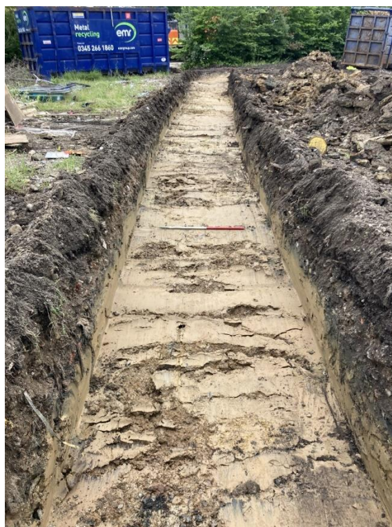
Plate 2. Overview of Trench 2, facing east, 1m scale
