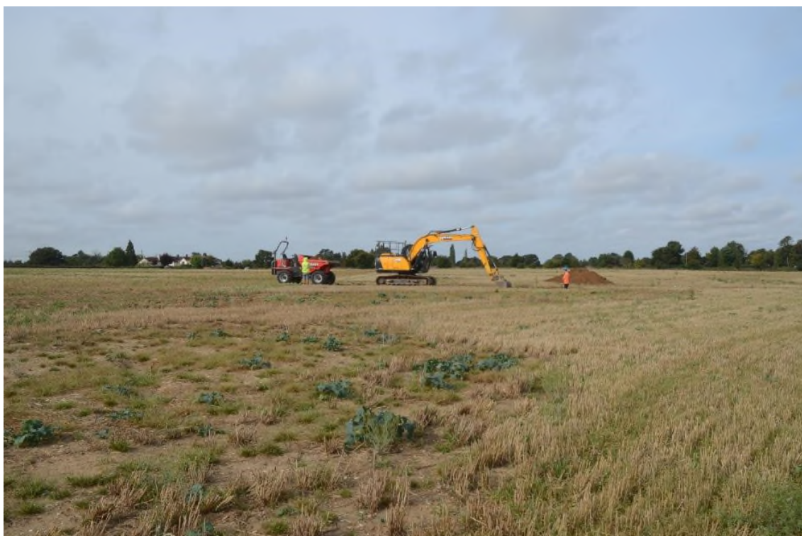
Plate 1: General view of the excavation area, looking west
