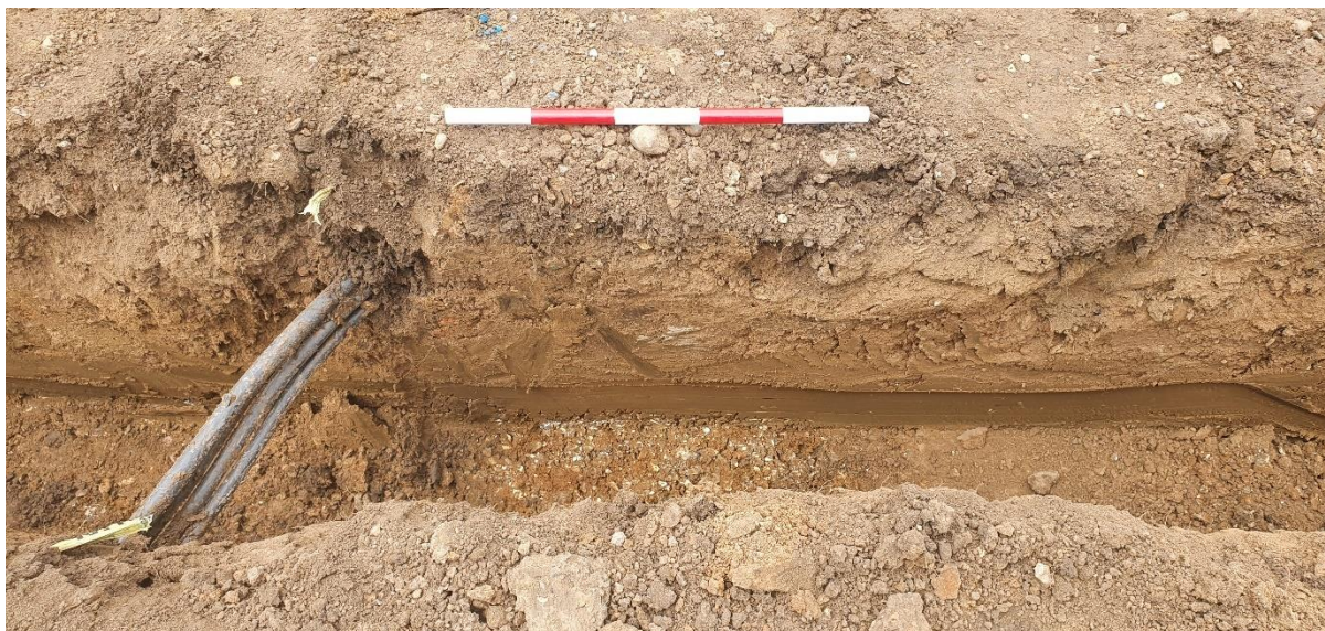
Plate 1: Layer [4] below matted material on surface, with underlying gravels [6] at the bottom of the trench, Section 1, looking west; 0.5m scale
