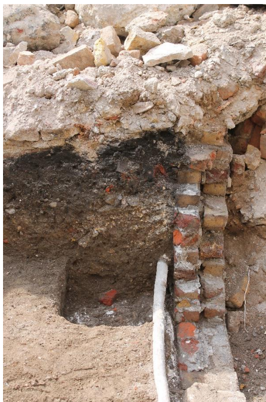
Plate 3. North facing section, in Trench 3, showing cellar wall [8], parallel running lead pipe [17] and chalk surface [16] observed in test pit (looking south)
