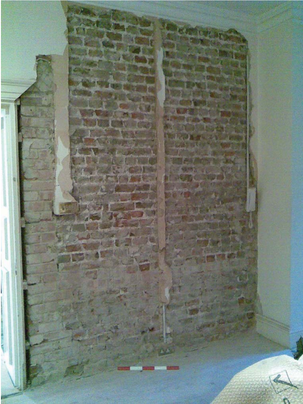
Plate 3. Ground Floor, Inner Hall, wall [11]. Scale is 0.50m
