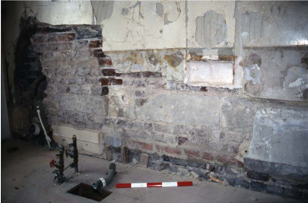
Plate 4. Second Floor, North Bathroom, wall [18]. Scale is 0.50m
