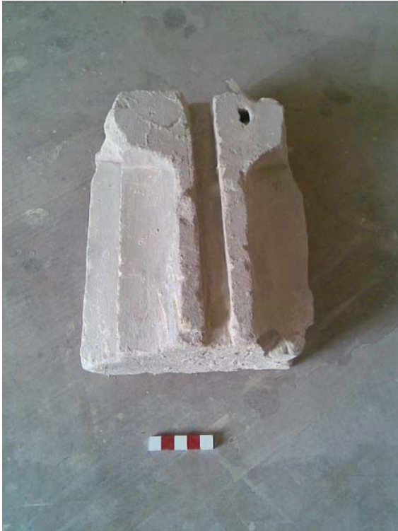
Plate 16. Stone 15, from 2 nd floor, main landing [11]. Taynton Stone. Medieval window moulding.
