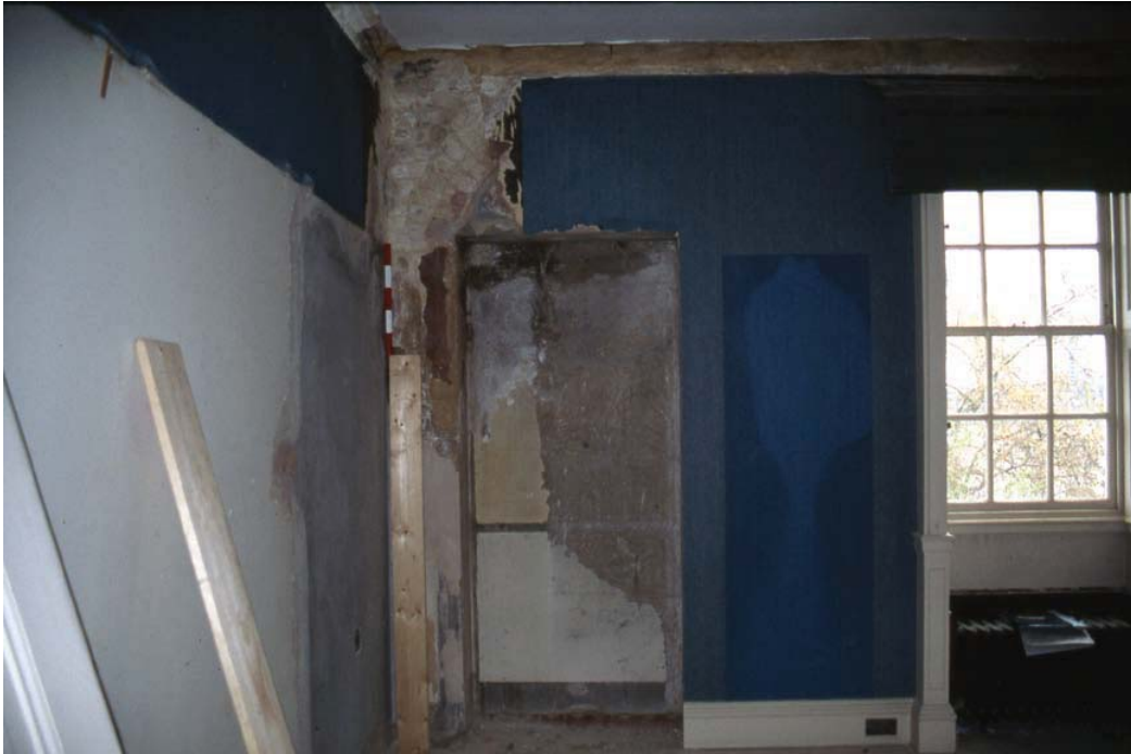
Plate 7. Second floor, bedroom 5, south wall. Scale is 0.50m
