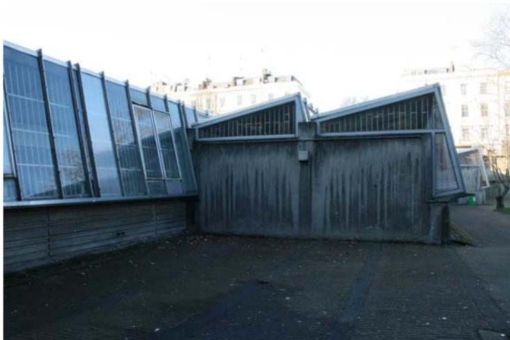
Plate 8 View of shutter marks on concrete, looking north-northwest
