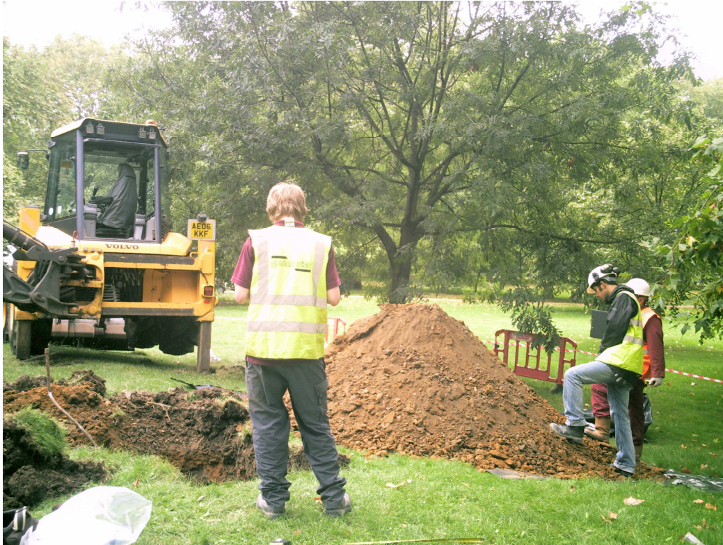
View of work on Test Pit 2, looking southwest.
