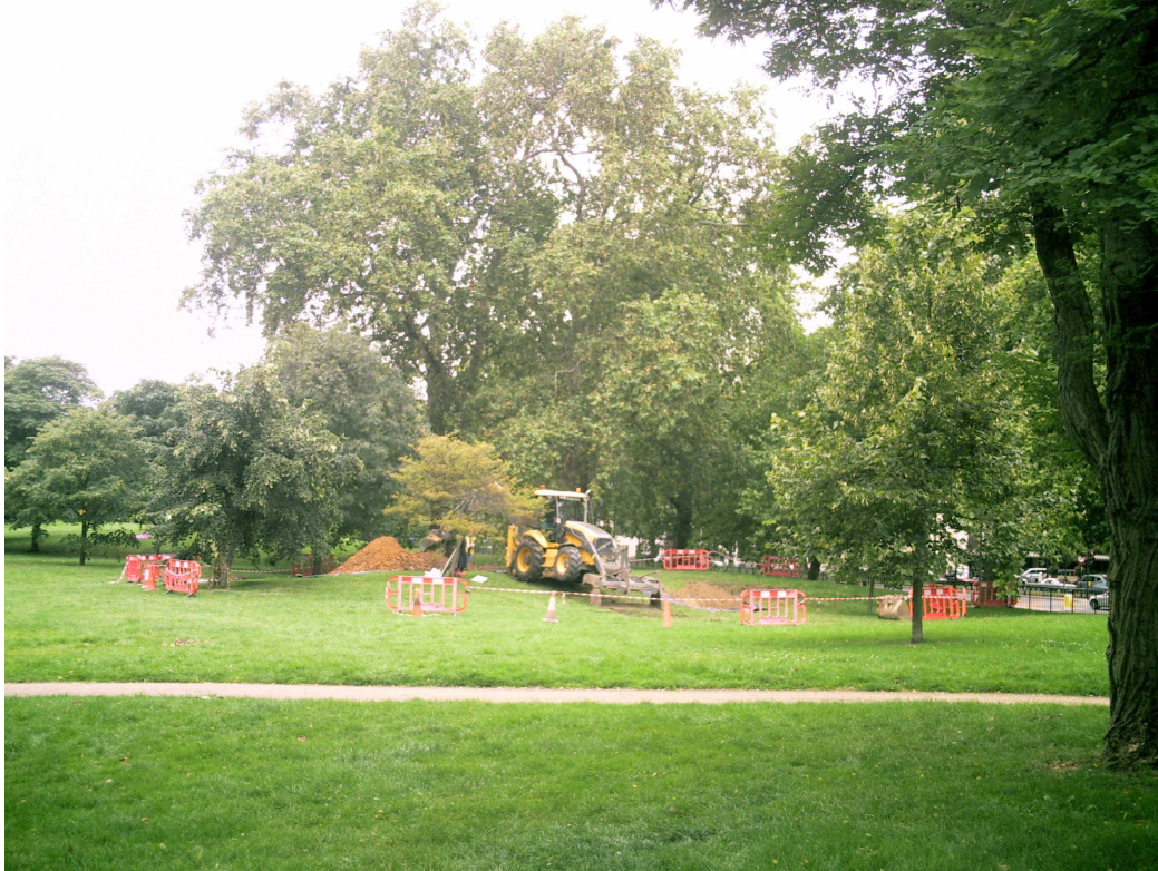
View of the site location, looking northwest.
