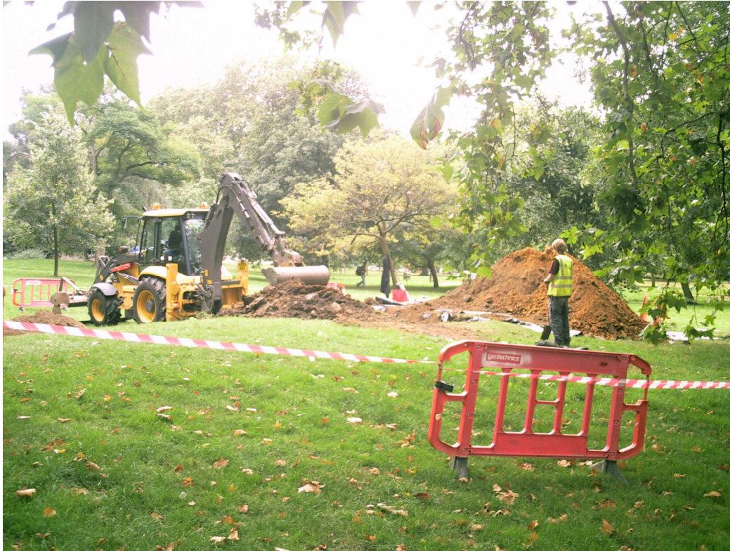
View of work on Trench 2, looking west.
