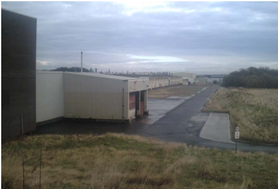
Plate 14. Road corridor south of factory, looking east.
