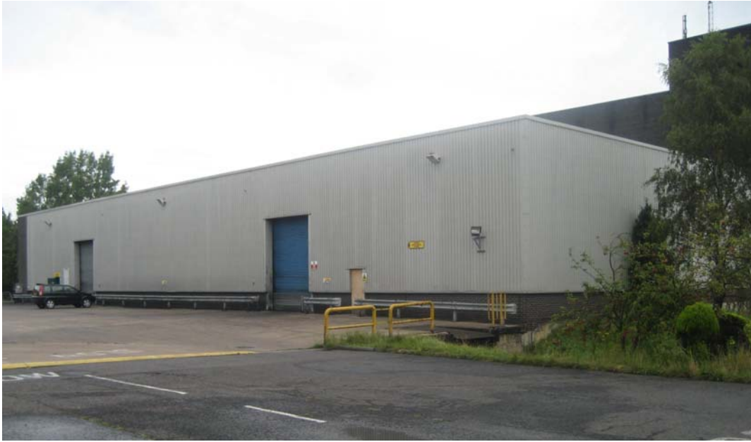
Plate 1. The tyre factory, western extension, looking north-east.
