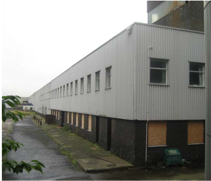
Plate 9. The tyre factory, west end of north elevation, looking south-east.
