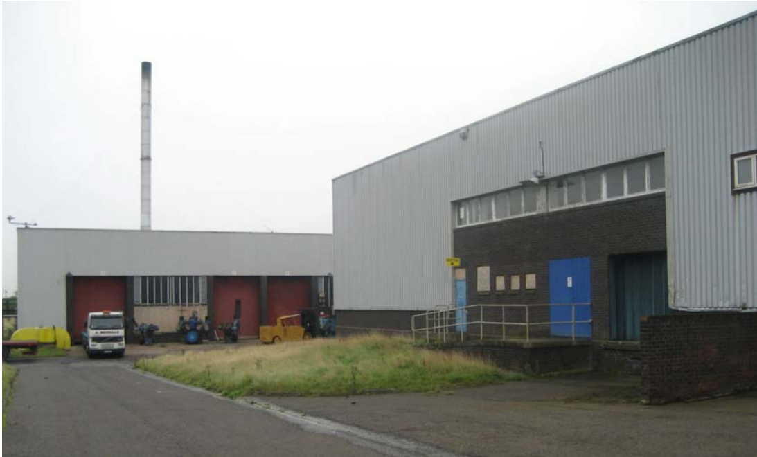
Plate 12. The tyre factory, north elevation, loading area detail, looking east.
