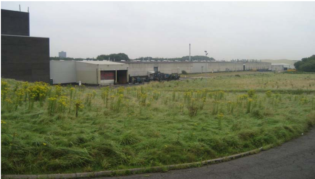
Plate 2. The tyre factory, south elevation, looking north-east.
