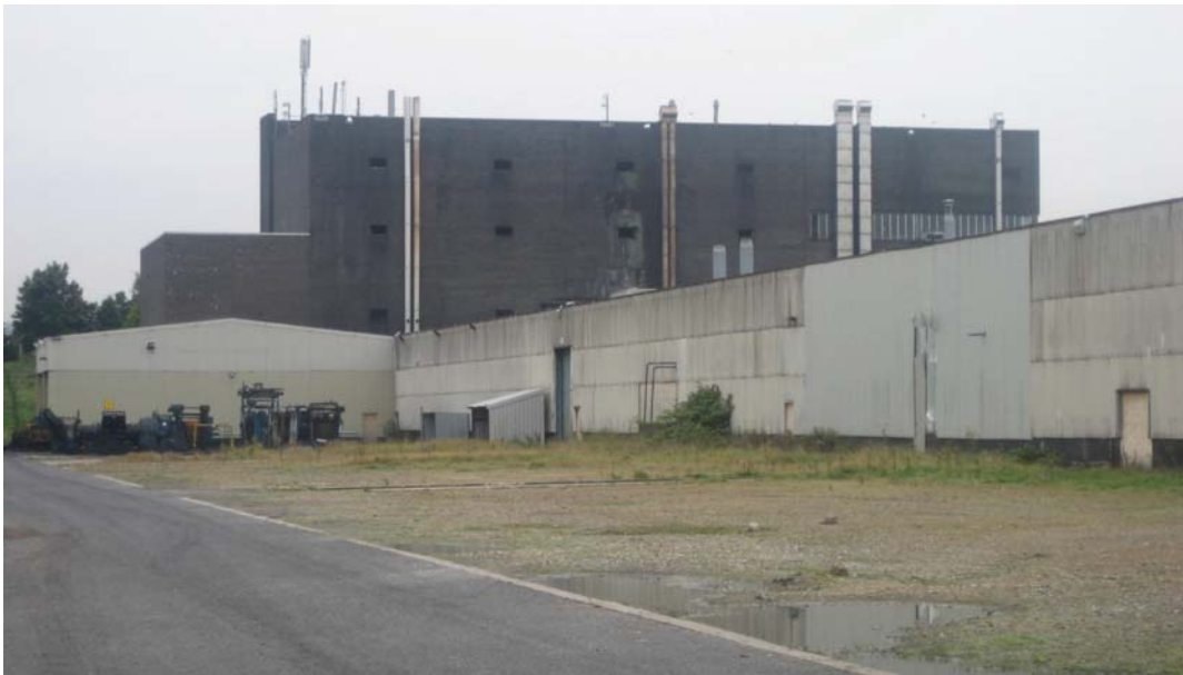
Plate 4. The tyre factory, south elevation detail and east elevation of brick block, looking north-west.
