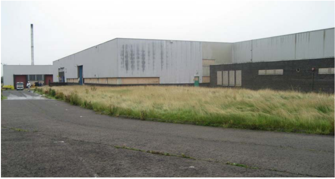
Plate 11. The tyre factory, extension to north elevation, looking east.
