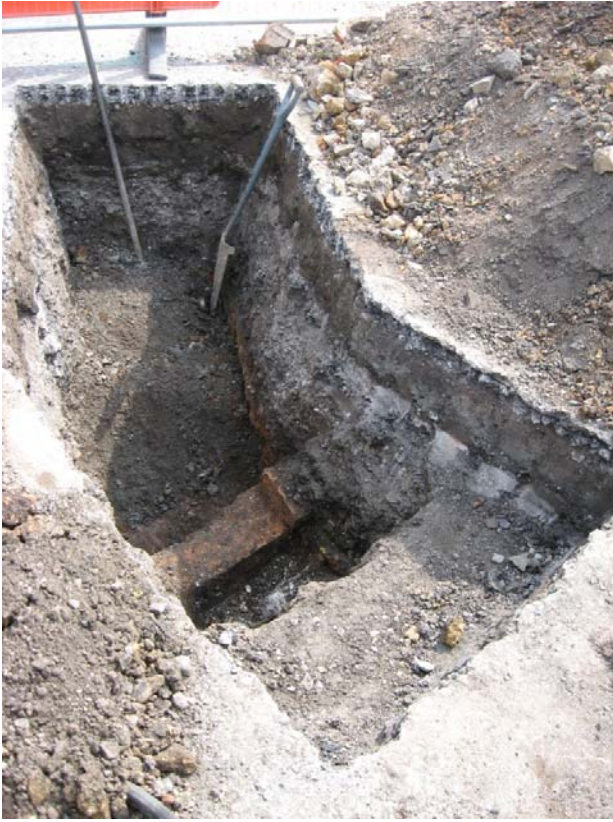
Plate 1-Test Pit 2 looking west
