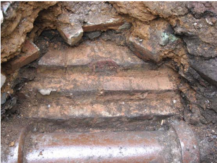
Plate 2-Test Pit 2 pipe and footings looking south-east
