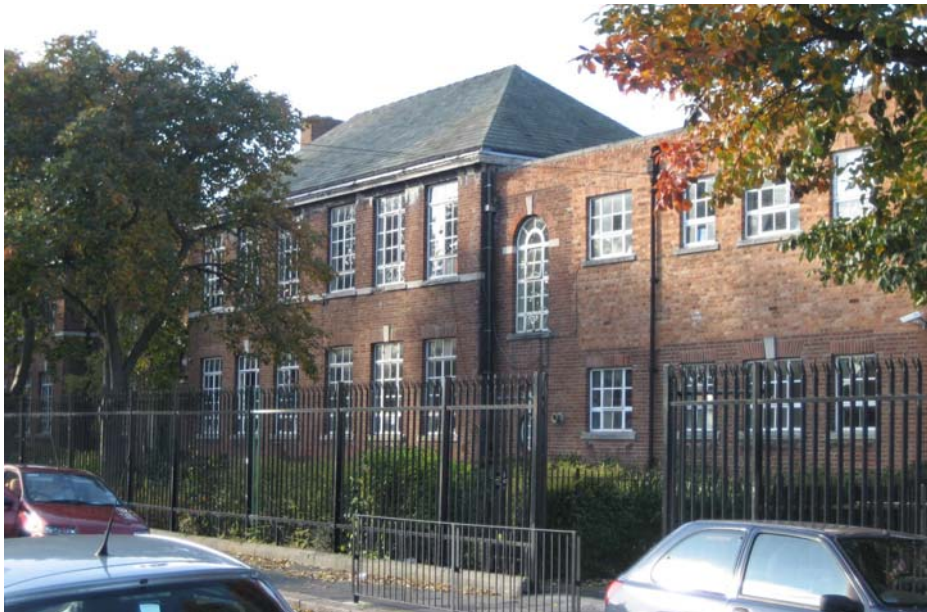
Plate 2. Original school building, south elevation, detail, looking north-west.
