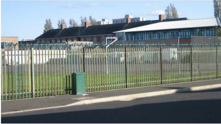
Plate 5. School complex, looking south-east.
