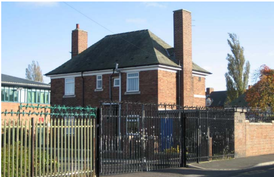
Plate 4. School House, north elevation, looking south-east.
