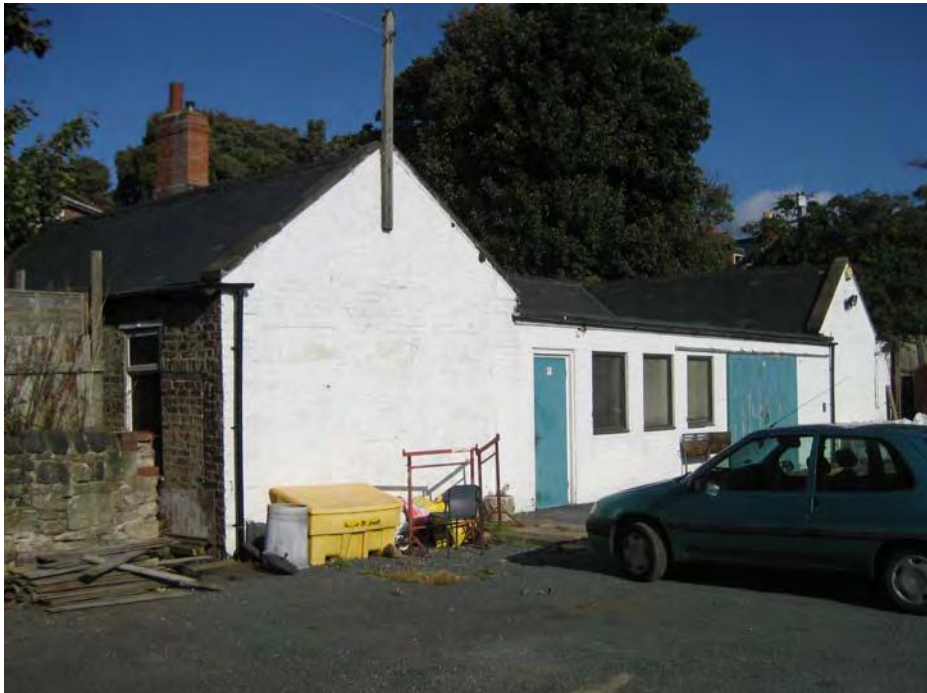
Plate 2. Brick building in northern boundary, looking north-east.
