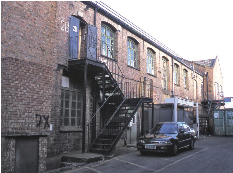
Plate 16 View of south elevation of Building 3, Peel Shed, looking north-east
