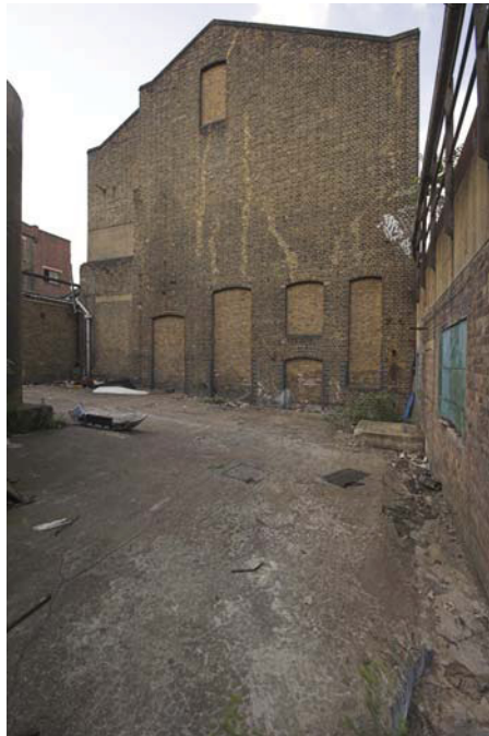
Plate 30 View of east elevation of Building 6, Engine House, looking west
