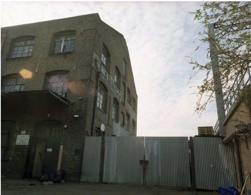
Plate 4 View of north-east corner of Building 1, Starch Department, looking south-west
