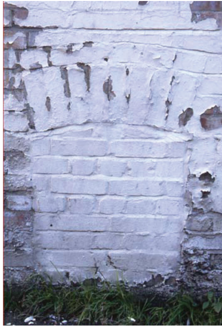
Plate 11 Detail of blocked fireplace at east end of north elevation of Building 2, Lozenge Department, looking south
