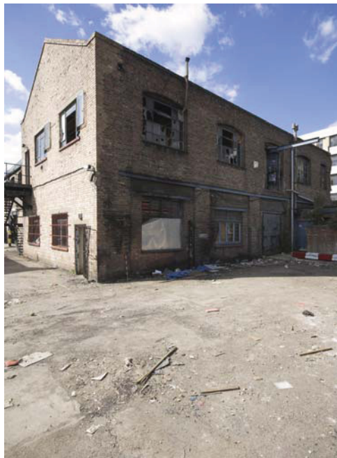
Plate 17 View of east elevation of Building 3, Peel Shed, looking north-west
