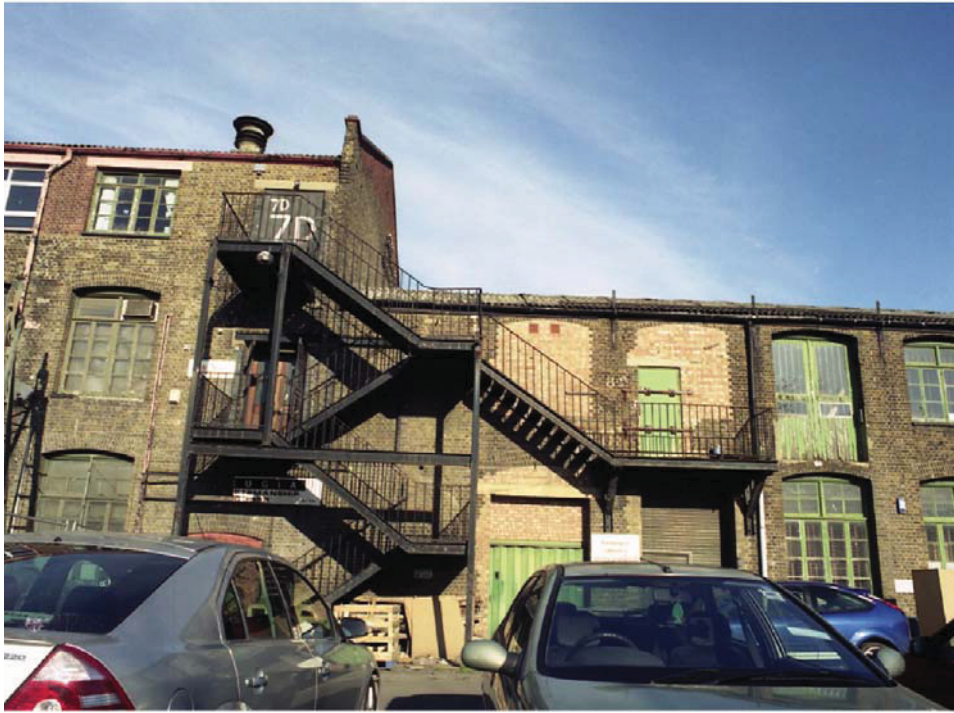
Plate 9 View of south elevation of Building 2, Lozenge Department, looking north
