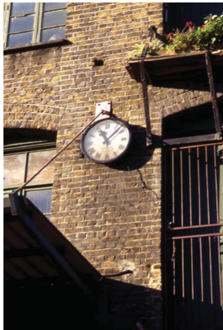
Plate 6 View of Building 1, Starch Department, detail of clock, looking west
