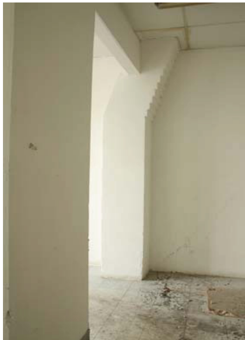
Plate 20 Internal view of Building 3, Peel Shed, detail of angled flue at ground floor, looking south-east
