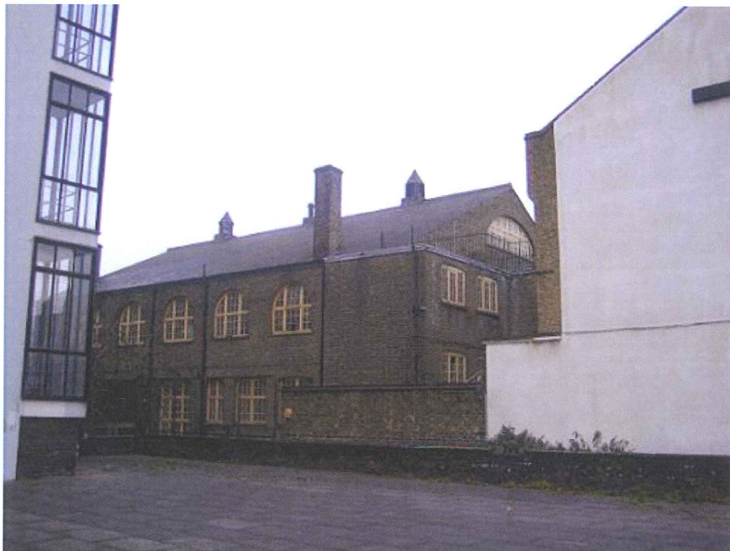
Plate 2: South elevation of the meeting hall building
