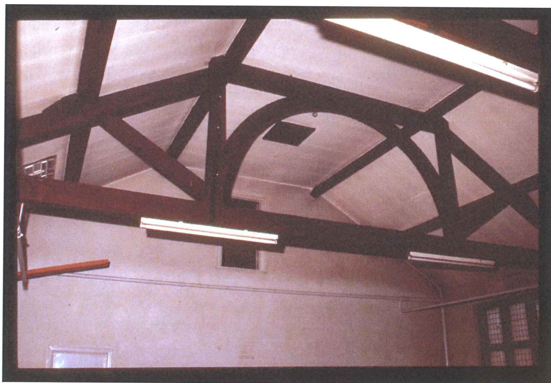
Plate 8: North roof truss in the 1926 building
