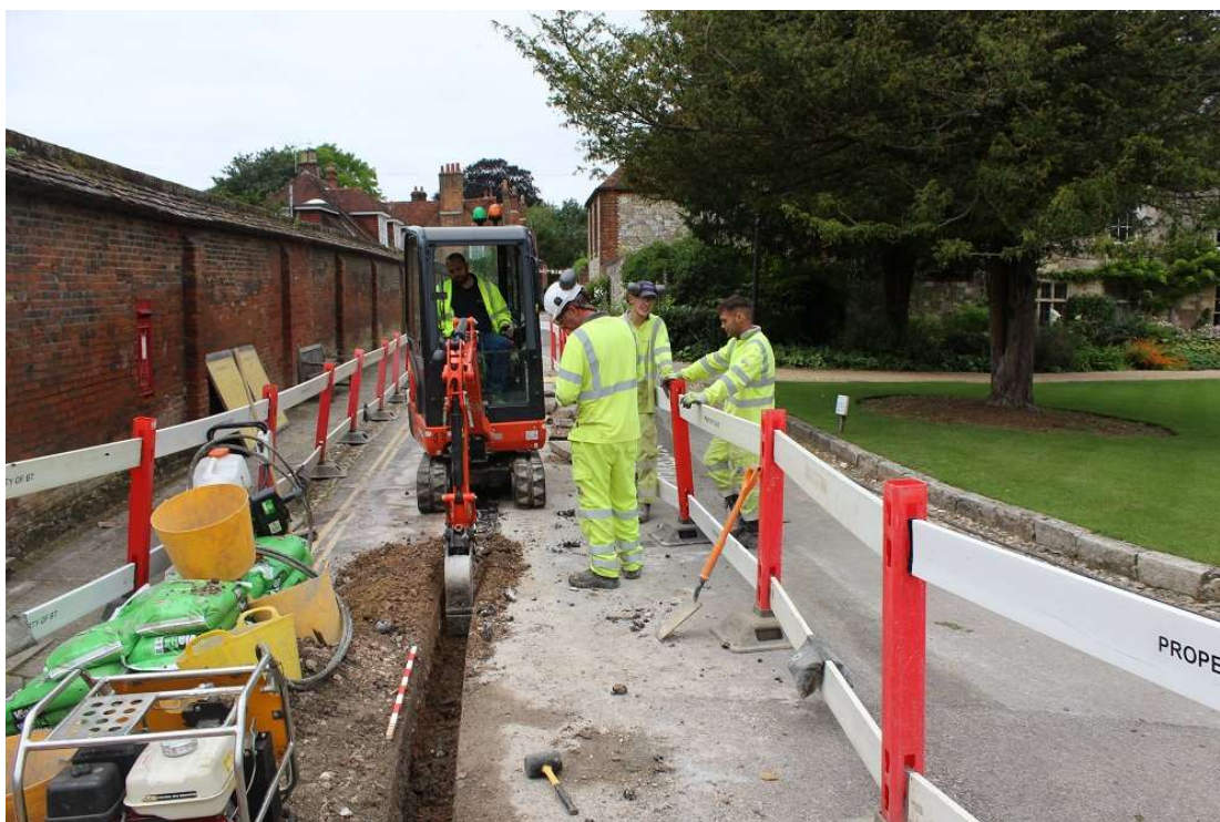
Plate 2. Cable trench excavation by machine in Dome Alley, view to west.
