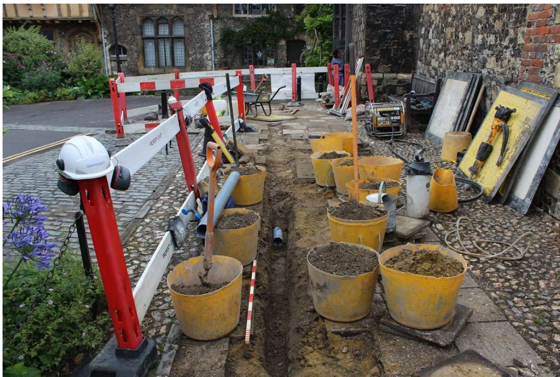
Plate 1. View of cable duct trench between Boxes 1 and 2, view to south.
