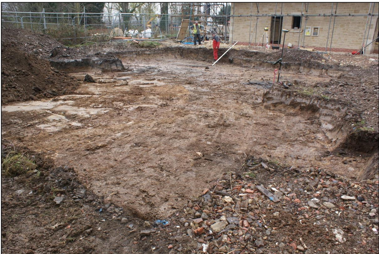
Plate 2: General view of watching brief area (House B), direction of view west.
