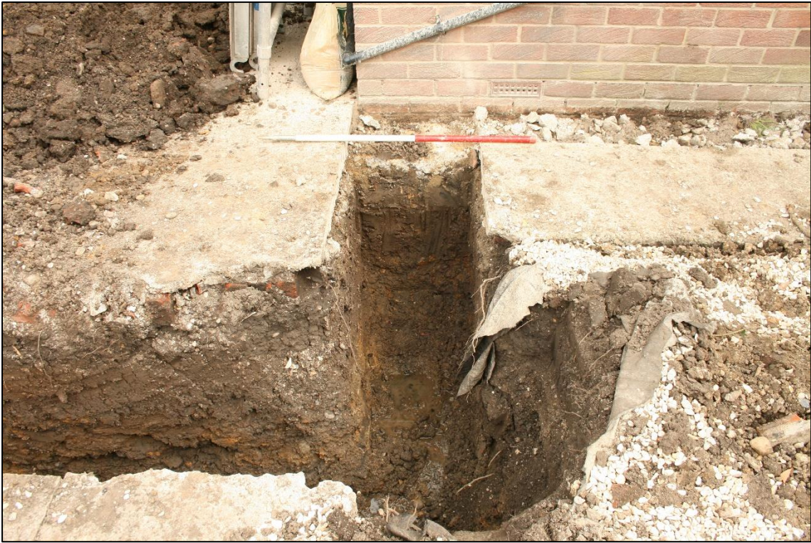
Plate 5-Overview of southern part of foundation trench, view east, 1m scale.
