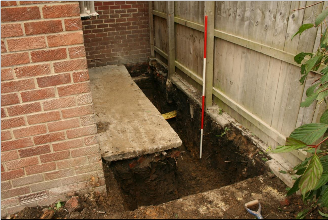
Plate 7-Overview of southern part of foundation trench, view south-east, 2m scale.
