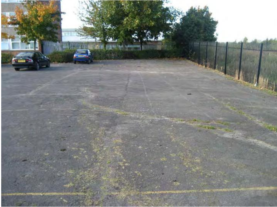
Plate 3. North-eastern portion of car park, looking north.
