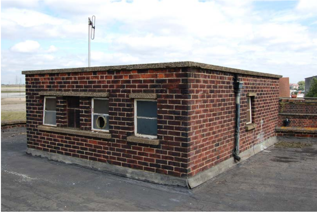
Plate 5: Second floor structure at the north end of the roof
