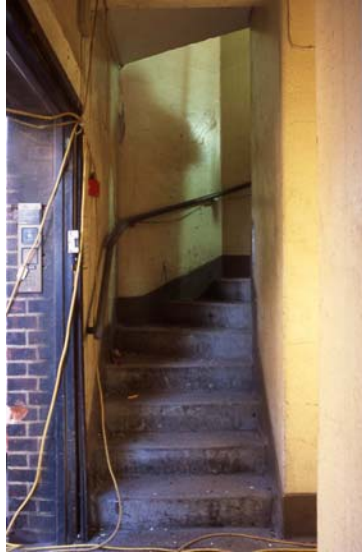
Plate 7: Stairwell from ground to first floor
