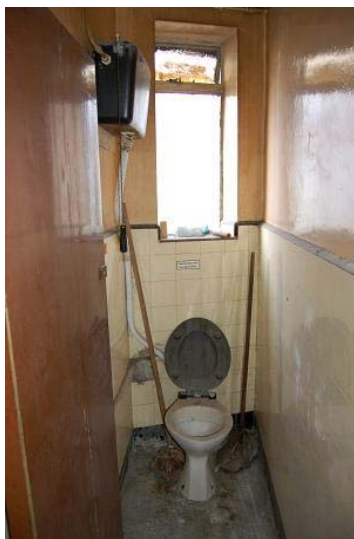
Plate 15: Room F3 on first floor
