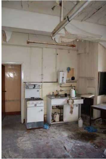
Plate 14: Kitchen area in room F2 on first floor
