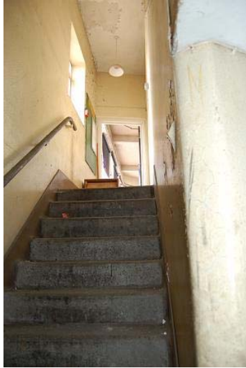
Plate 13: Stairwell and corridor (room F1) on first floor
