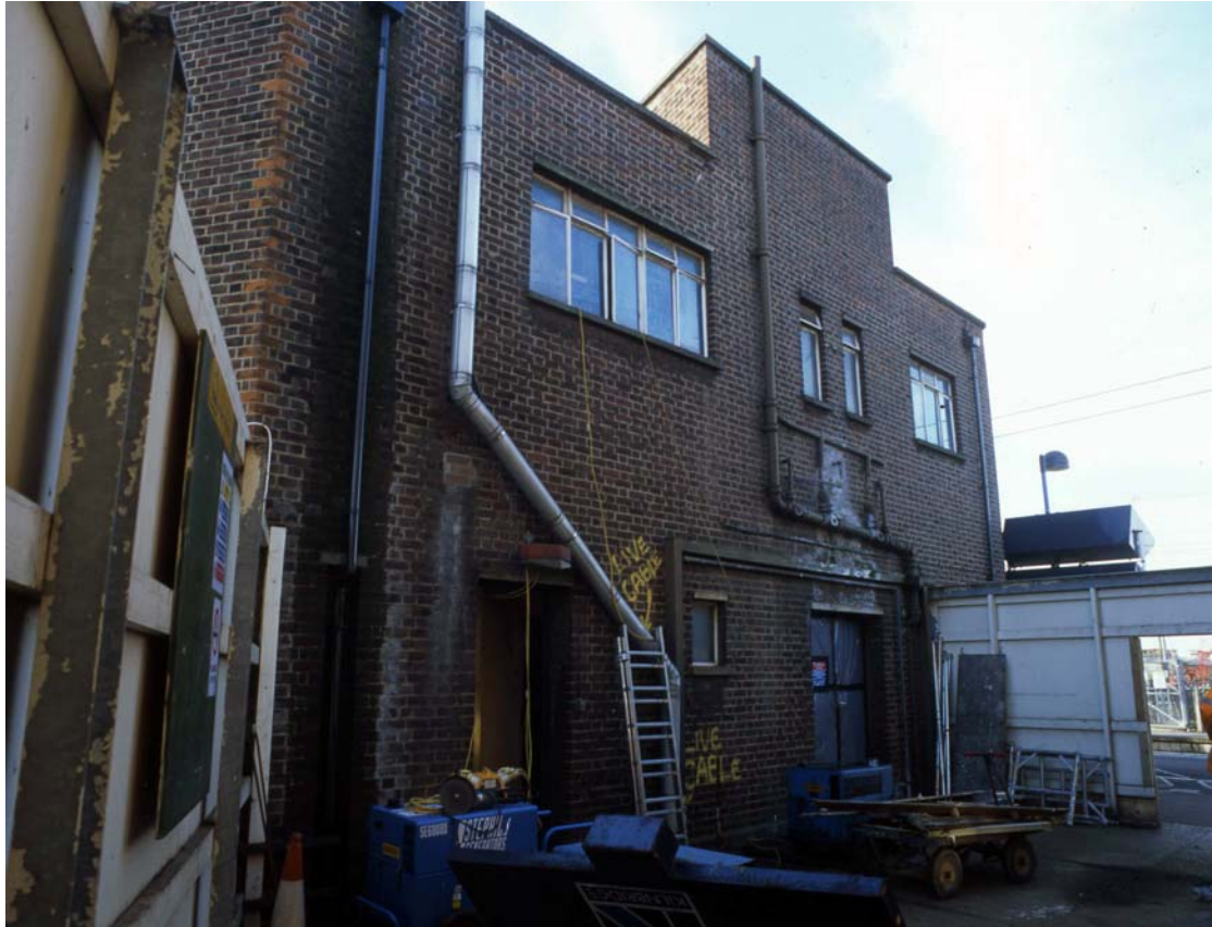
Plate 3: North elevation of signal box
