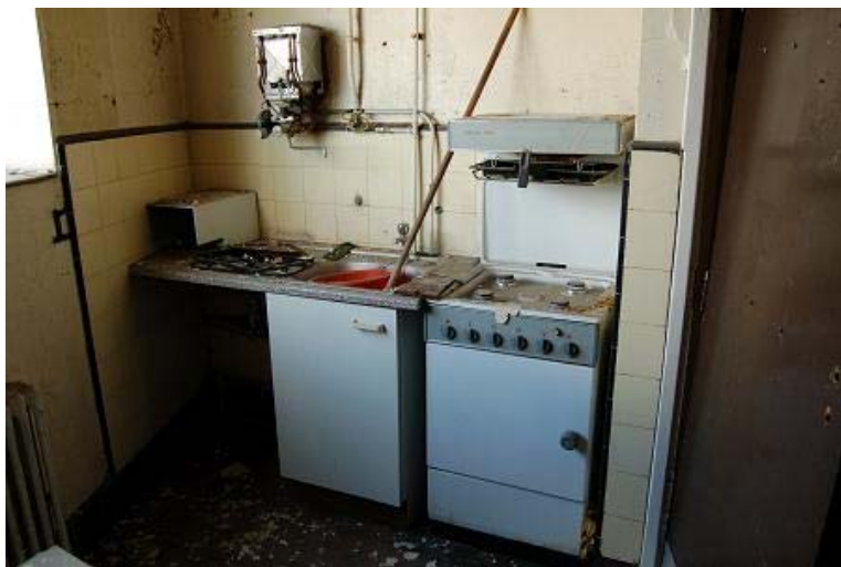
Plate 18: Kitchen area in room F6 on first floor
