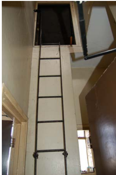
Plate 17: Original metal ladder in room F5 on first floor
