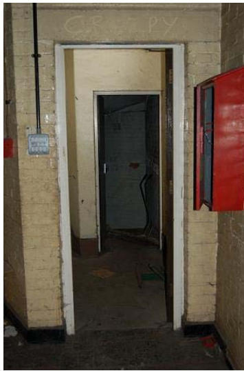
Plate 8: Ground floor corridor and basement access
