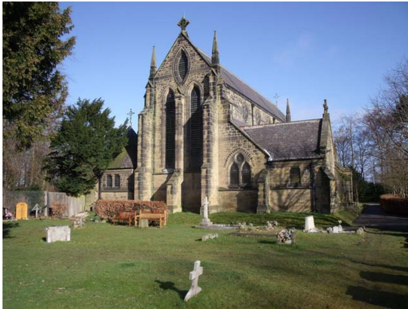
Plate 6. Church of St. John the Baptist, south elevation, looking NNE.
