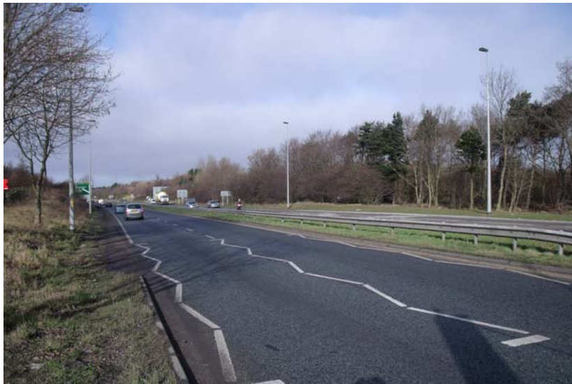
Plate 2. View from Moor Farm Junction along the A19, looking WNW.
