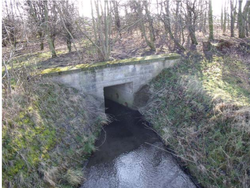
Plate 7. Culverting of Seaton Burn tributary, west of the A189, looking east.
