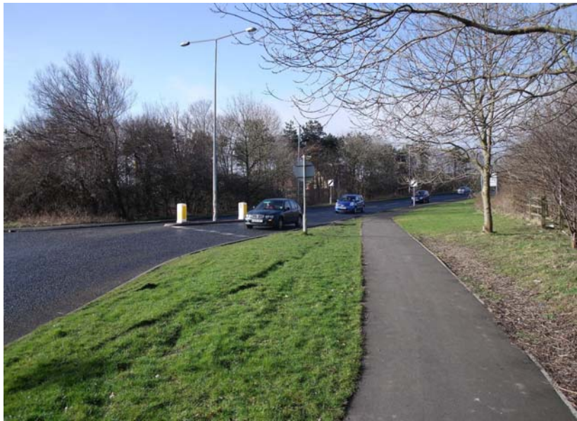
Plate 4. View from Moor Farm Junction along the A1171, looking south-west.
