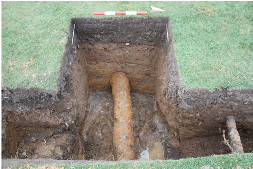
West Facing Shot of Cast Iron Pipe (0.50m Scale)
