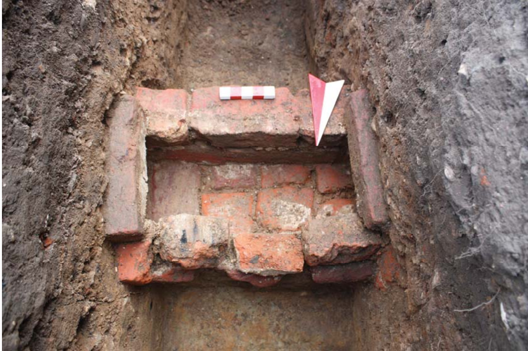
South Facing Shot of Culvert with Capping Removed (0.10m Scale)
