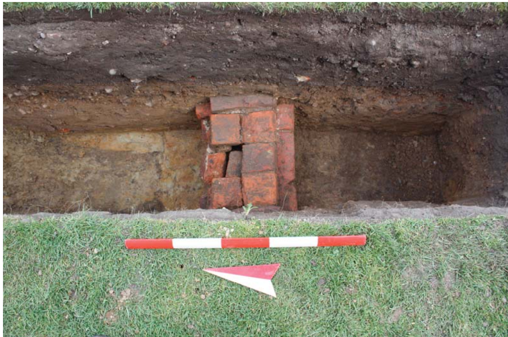
East Facing Shot of Brick Culvert with Capping (0.50m Scale)
