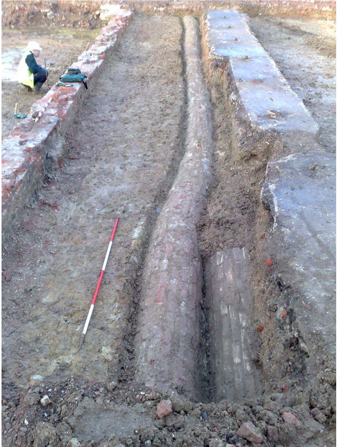
PLATE 7: Culvert [2203] looking north with 2m scale
