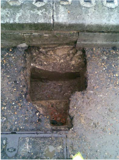
Plate 5: View north in Trench E091 B
