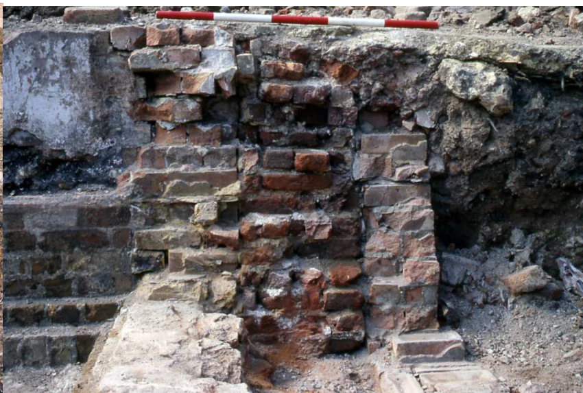
Plate 12 – Detail of wall foundations [10], [11] and [12] in south-east facing section of Trench 8
