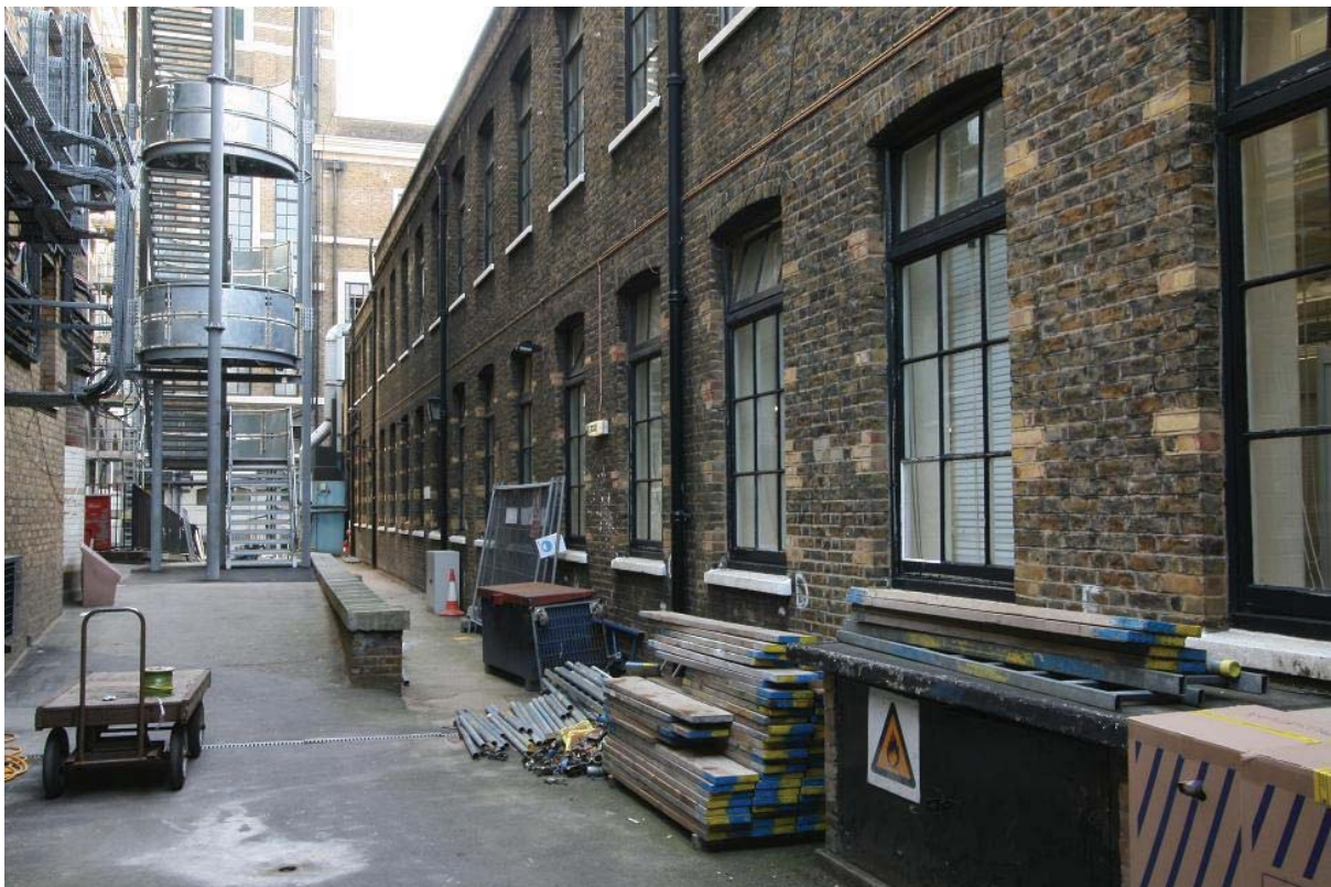
Plate 2: East end of the north elevation of the Bindery.
