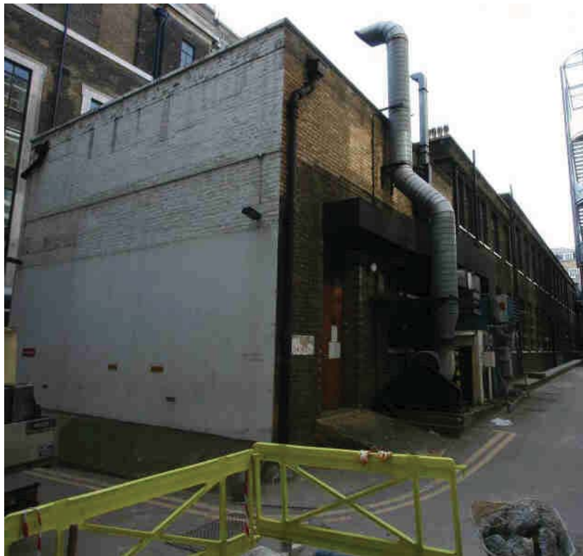
Plate 4: North and east elevations of the Bindery.
