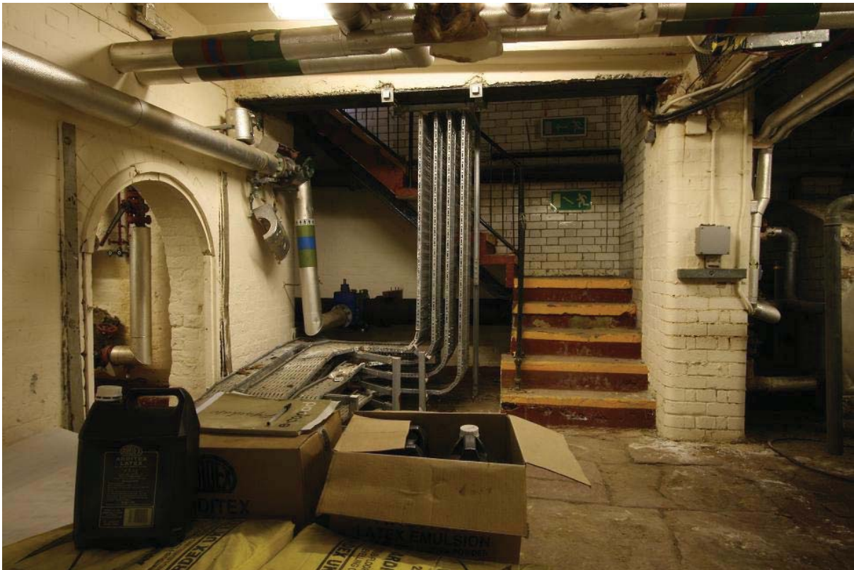
Plate 10: Bindery basement with archway to coal bunker on left.
