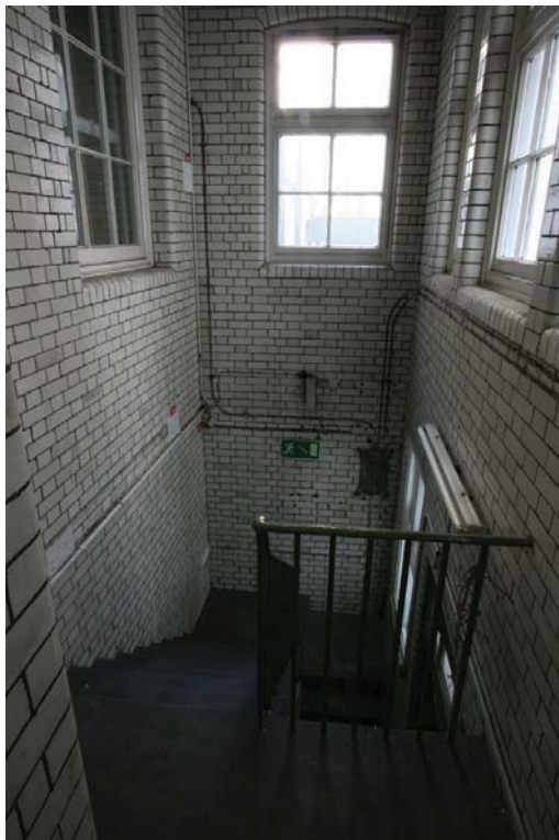
Plate 18: Bindery stairwell BMB/2/6 looking down to ground floor.
