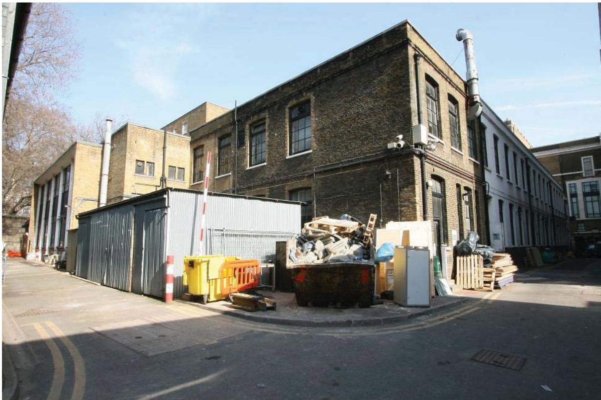
Plate 8: West elevation of the Bindery with modern yellow brick extension on the left.
