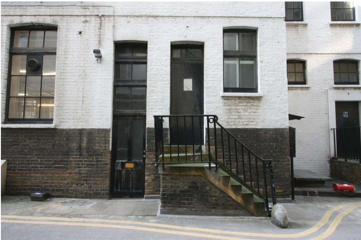
Plate 6: Lowered doorway to basement and steps up to stairwell to first floor.
