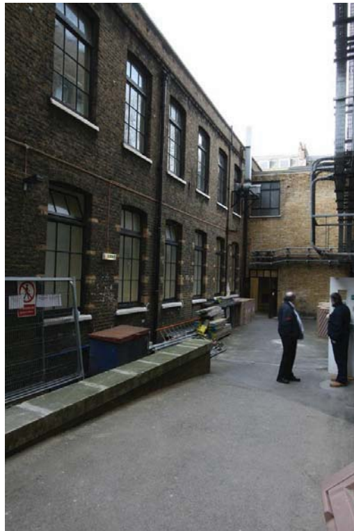
Plate 1: West end of the north elevation of the Bindery.
