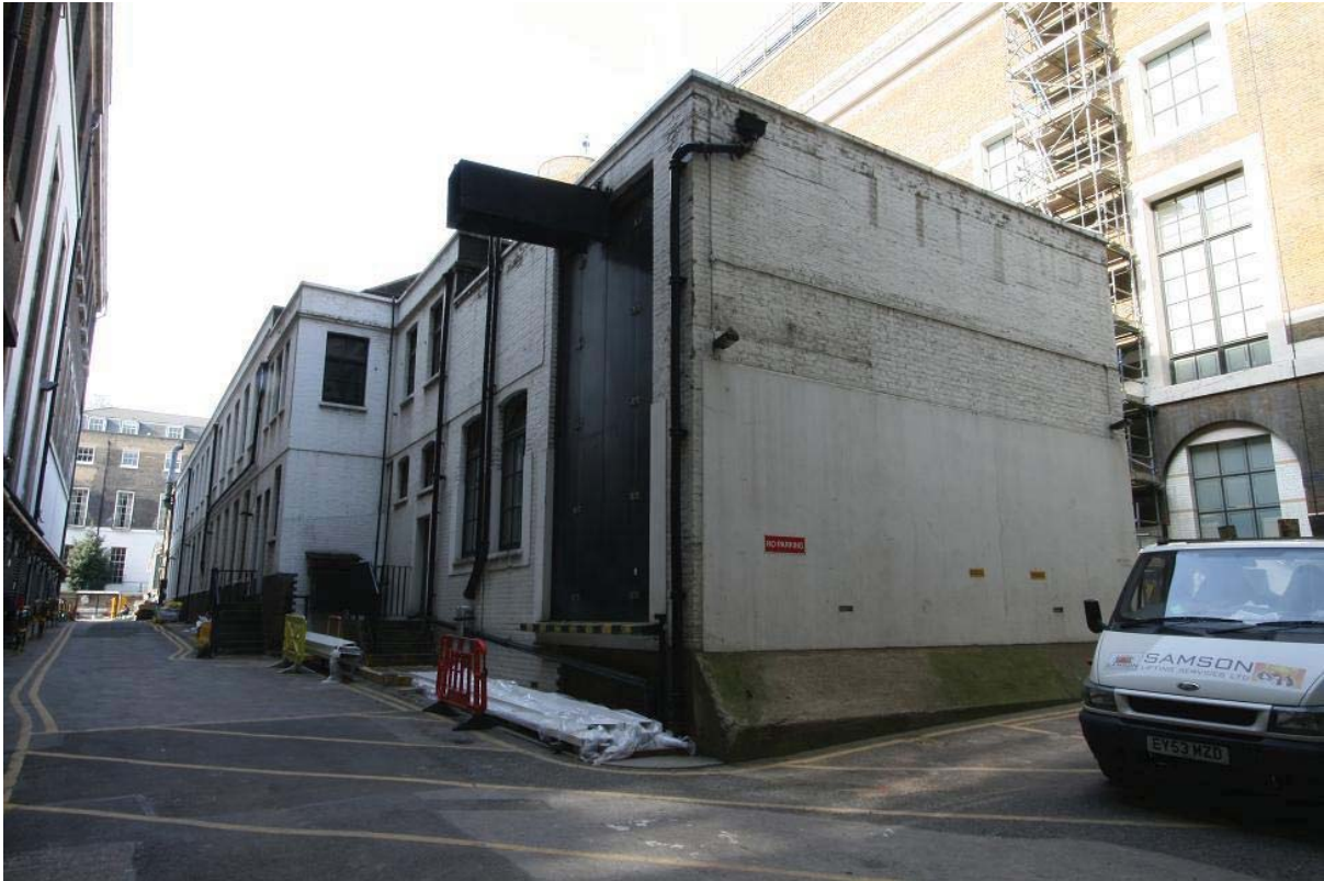
Plate 5: East and south elevations of the Bindery.
