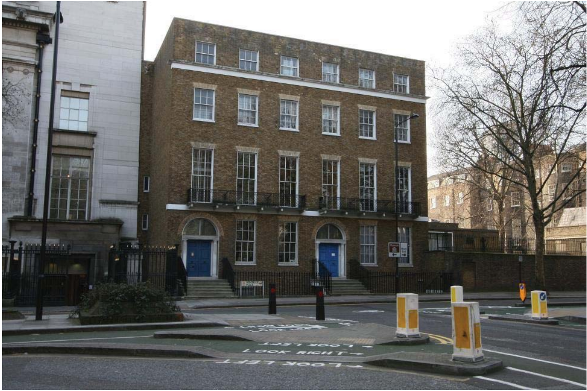
Plate 23: North elevation of 1-2 Montague Place.
