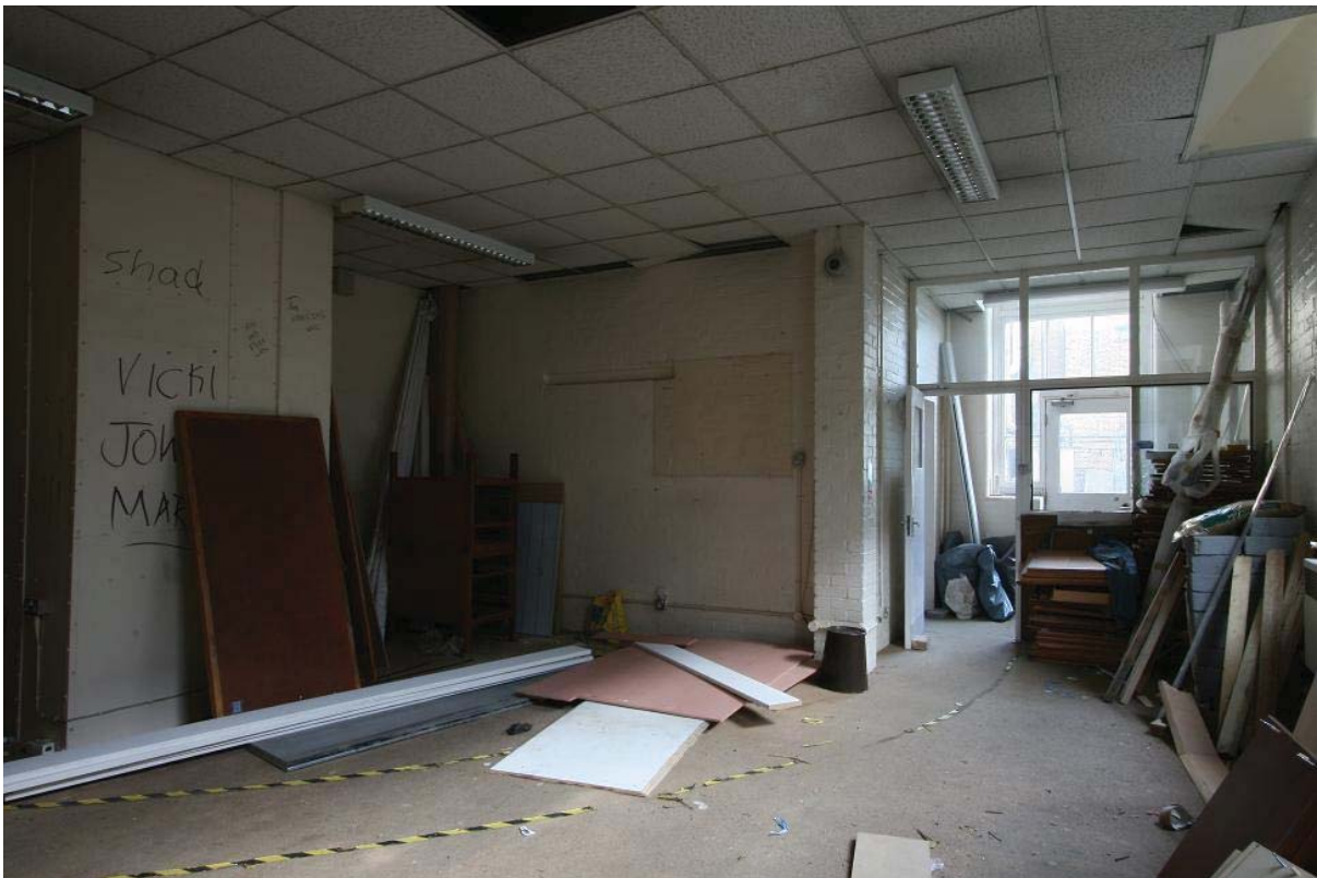
Plate 12: Ground floor office at the west end of the Bindery (BMB/1/1).
