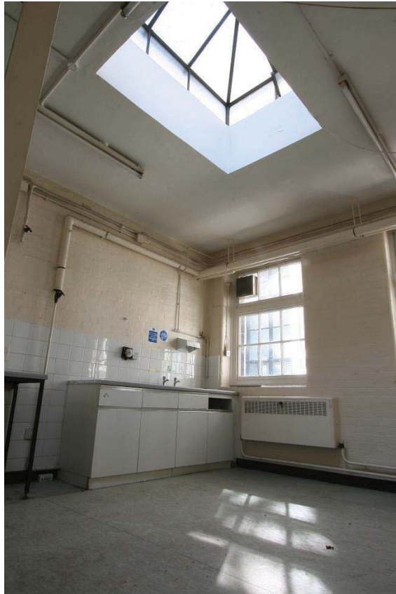
Plate 17: Bindery first floor kitchen BMB/2/8.
