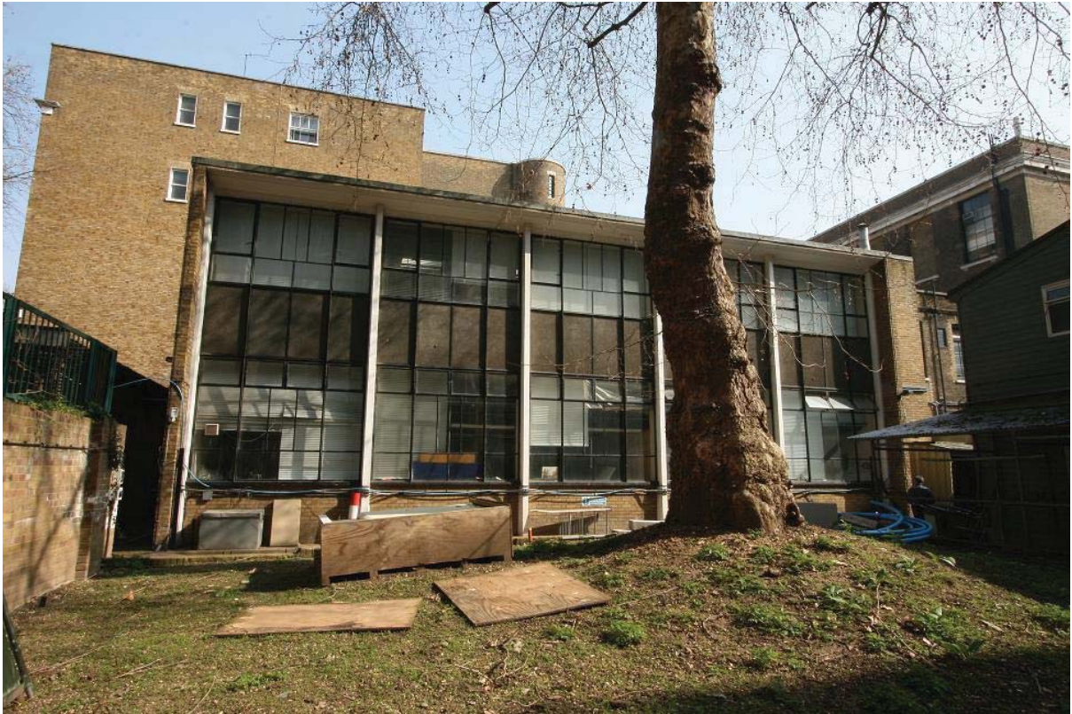
Plate 19: West elevation of the Bindery extension.
