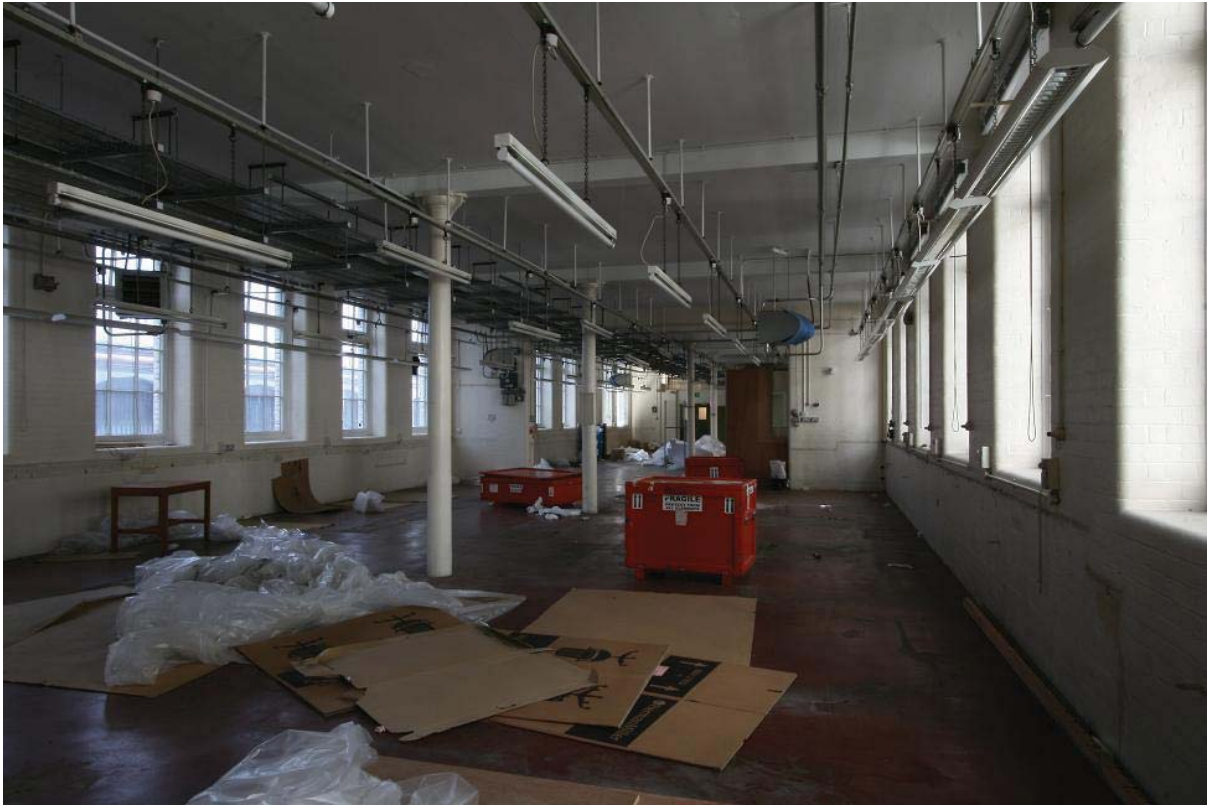
Plate 13: Bindery ground floor workroom, looking west (BMB/1/5).
