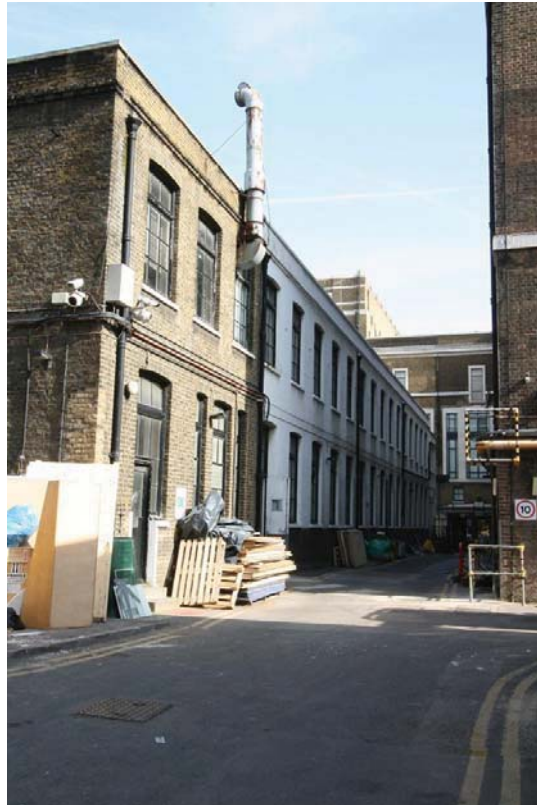
Plate 7: South elevation of the Bindery, looking north east.
