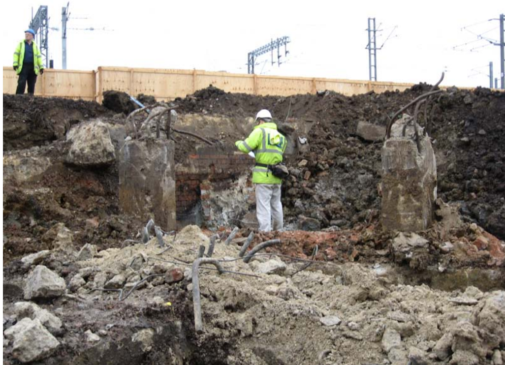
Plate 4 The Water Softening Plant
