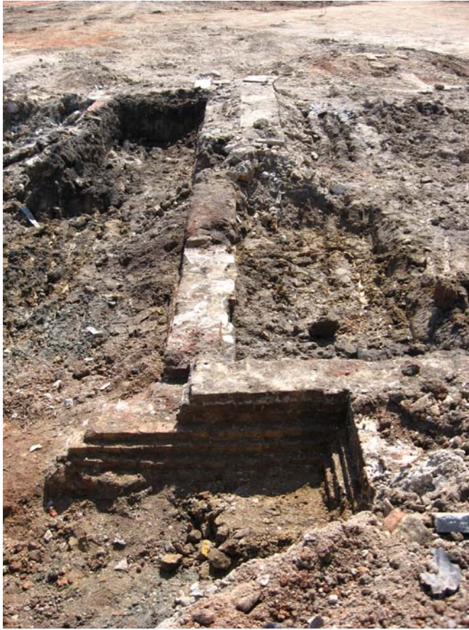
Plate 1 Wall foundation [220] looking south (wall of Saddler's Shop)
