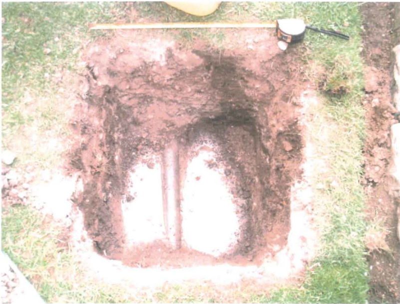
Plate 1: Trench E198 A, facing north.
