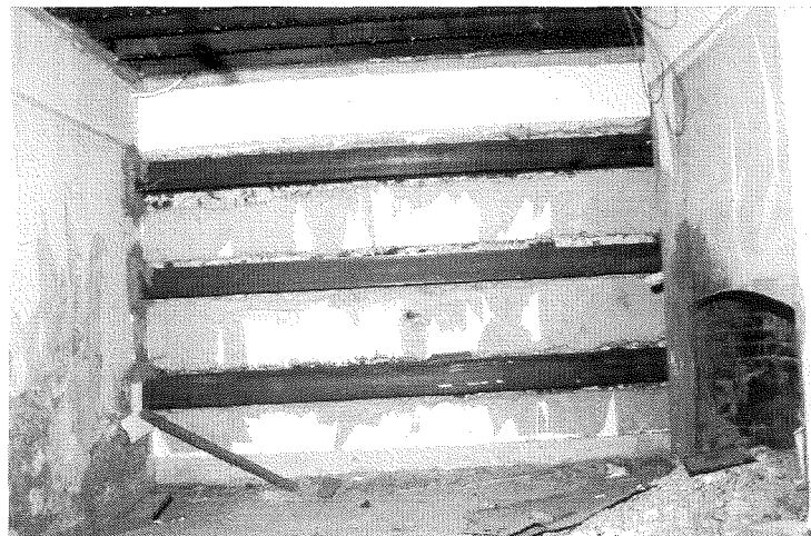
Plate 2: 'I' section beams in the north of the basement
