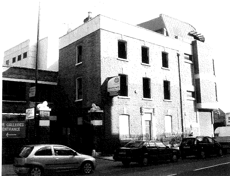
Plate 1: 15 Dock Street from the south
