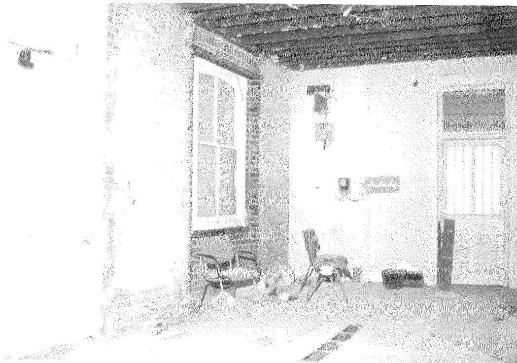
Plate 3b: Interior, ground floor, looking north
