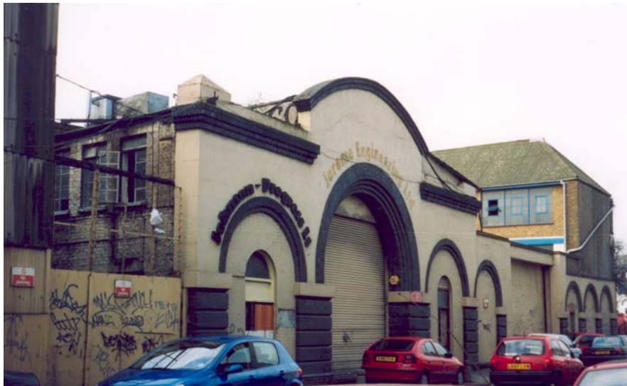
Plate 6b: East elevation of Buildings J1-J5
