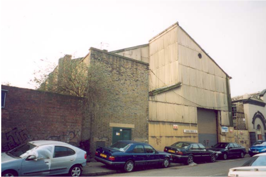
Plate 6a: East elevation of Buildings J1-J5
