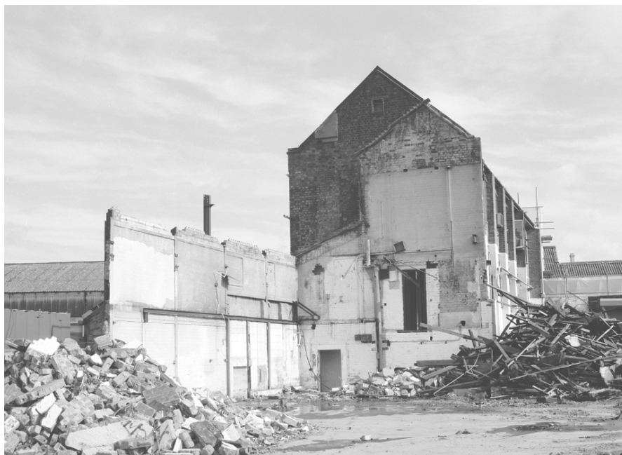
Plate 5: West elevation of Building J5
