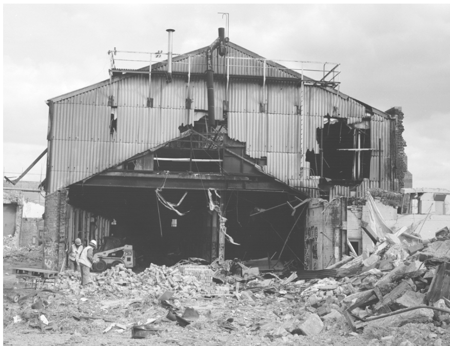
Plate 1: West Elevation of Building J1
