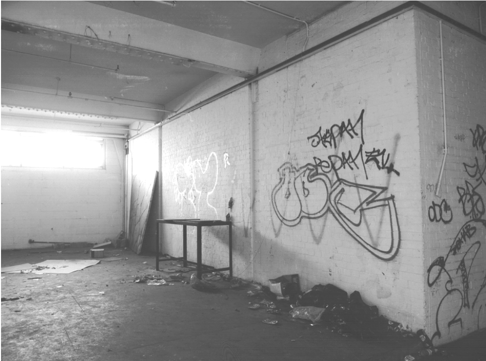
Plate 9: East ground floor of Building Y3
