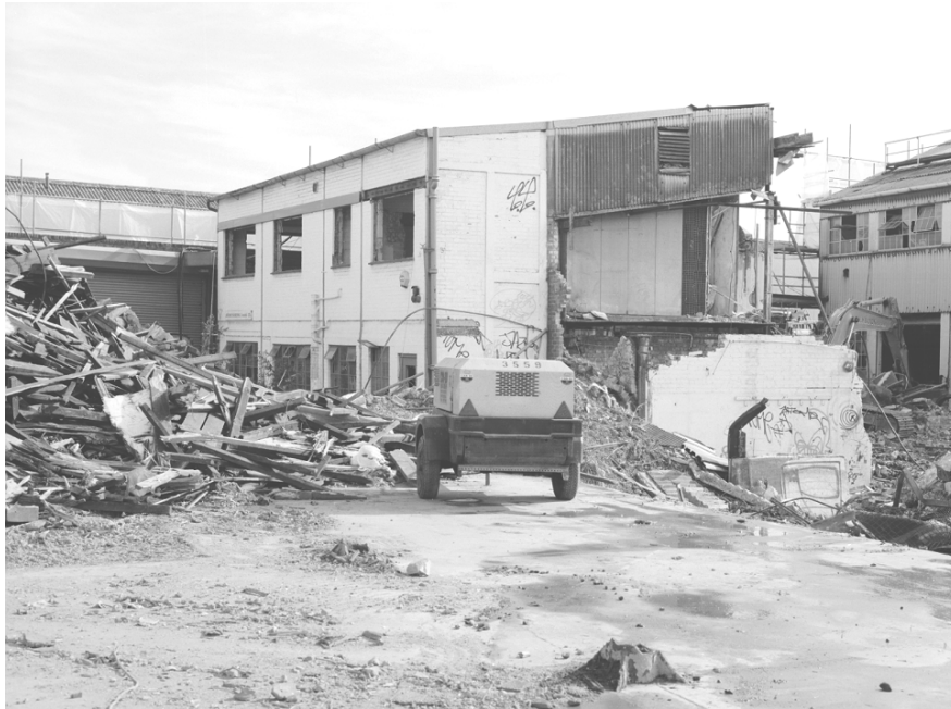
Plate 4: West elevation of Building J3
