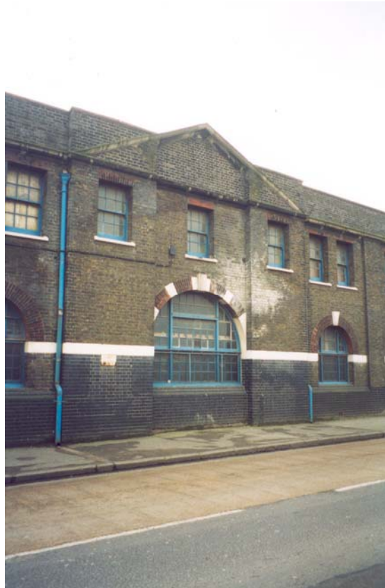
Plate 15: Centre of east elevation of Building Y5
