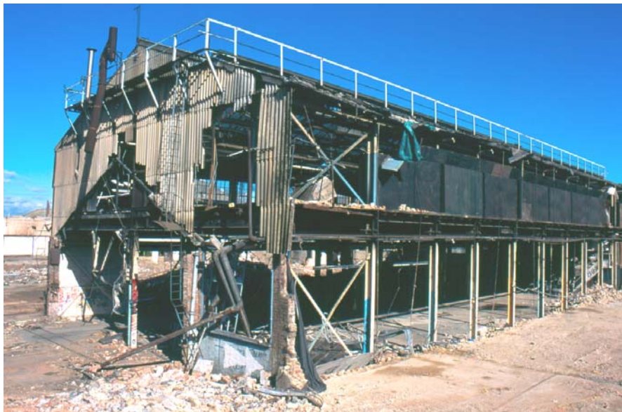
Plate 3: South Elevation of Building J1 showing exposed steel framing
