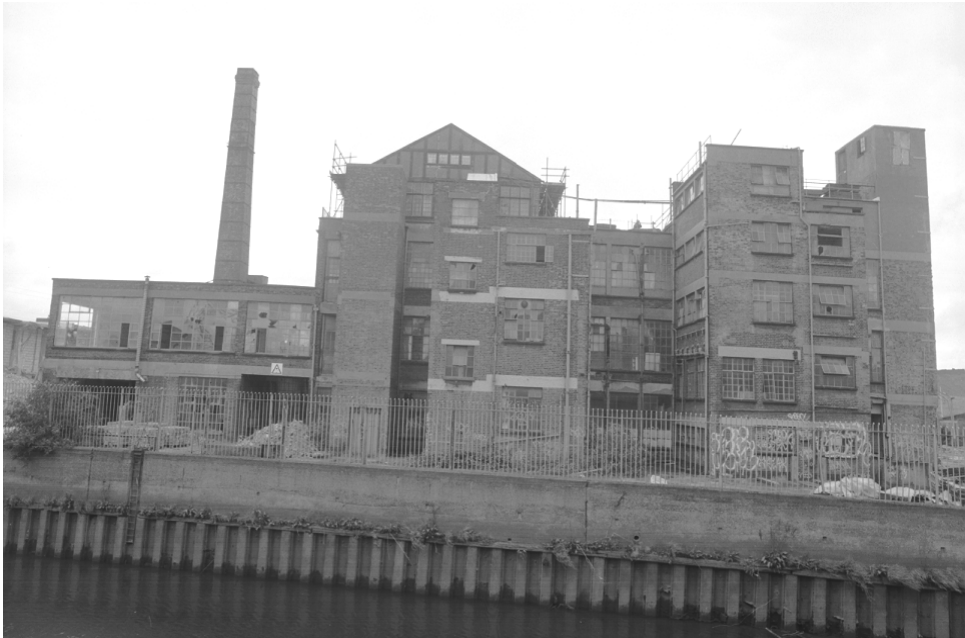
Plate 14: West elevation of Buildings Y3 and Y4
