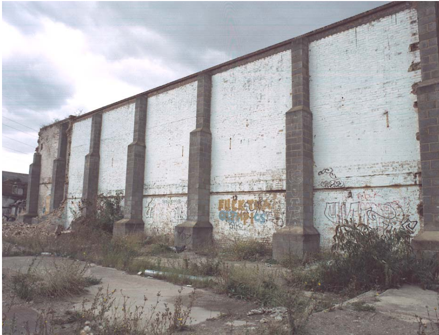
Plate 2: South Elevation of Building J1
