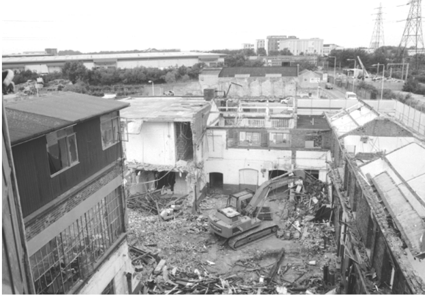
Plate 16: Buildings Y5 and Y6 during demolition
