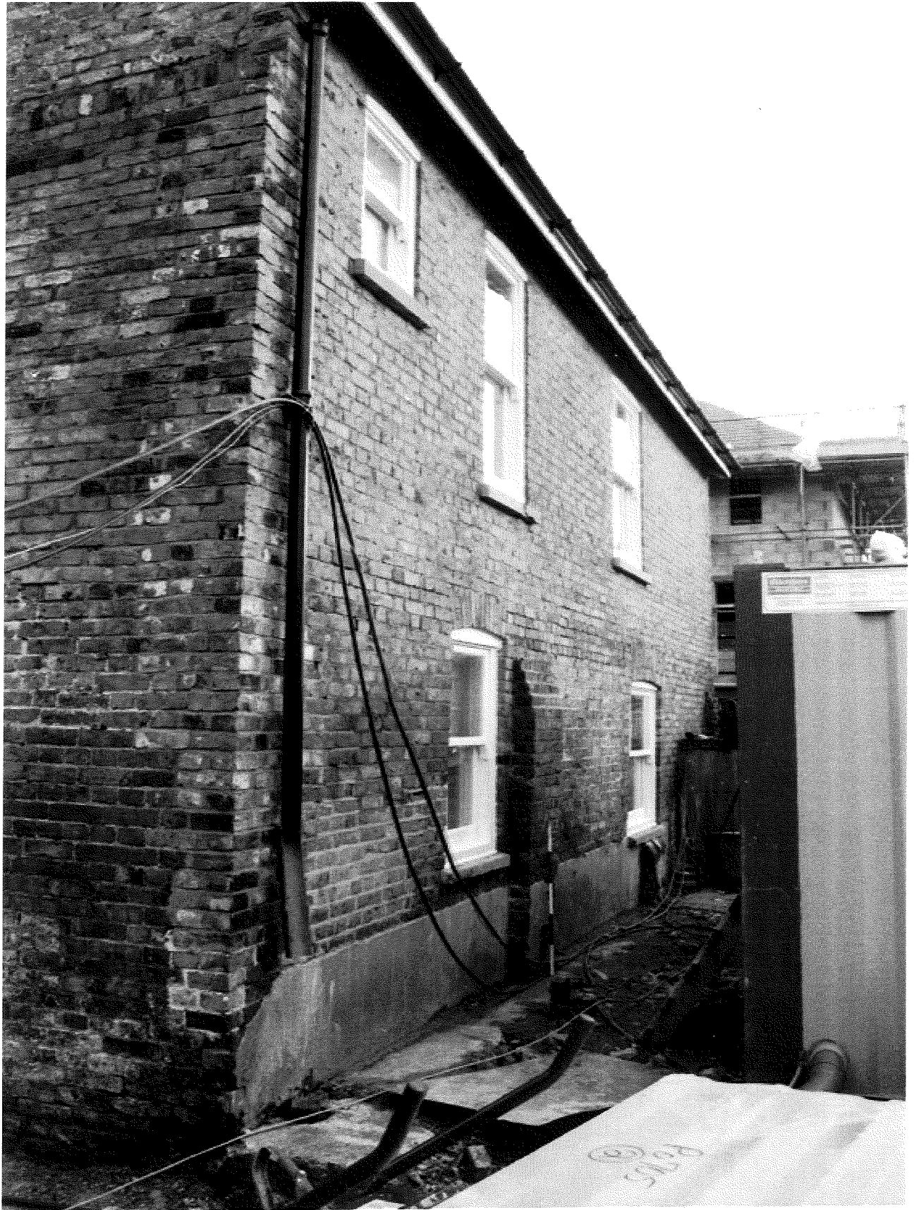
Figure 33 North elevation of the cottage
