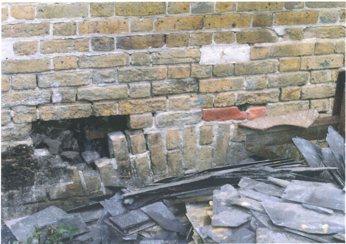
Figure 9 Details of the eastern elevation of the boiler house
