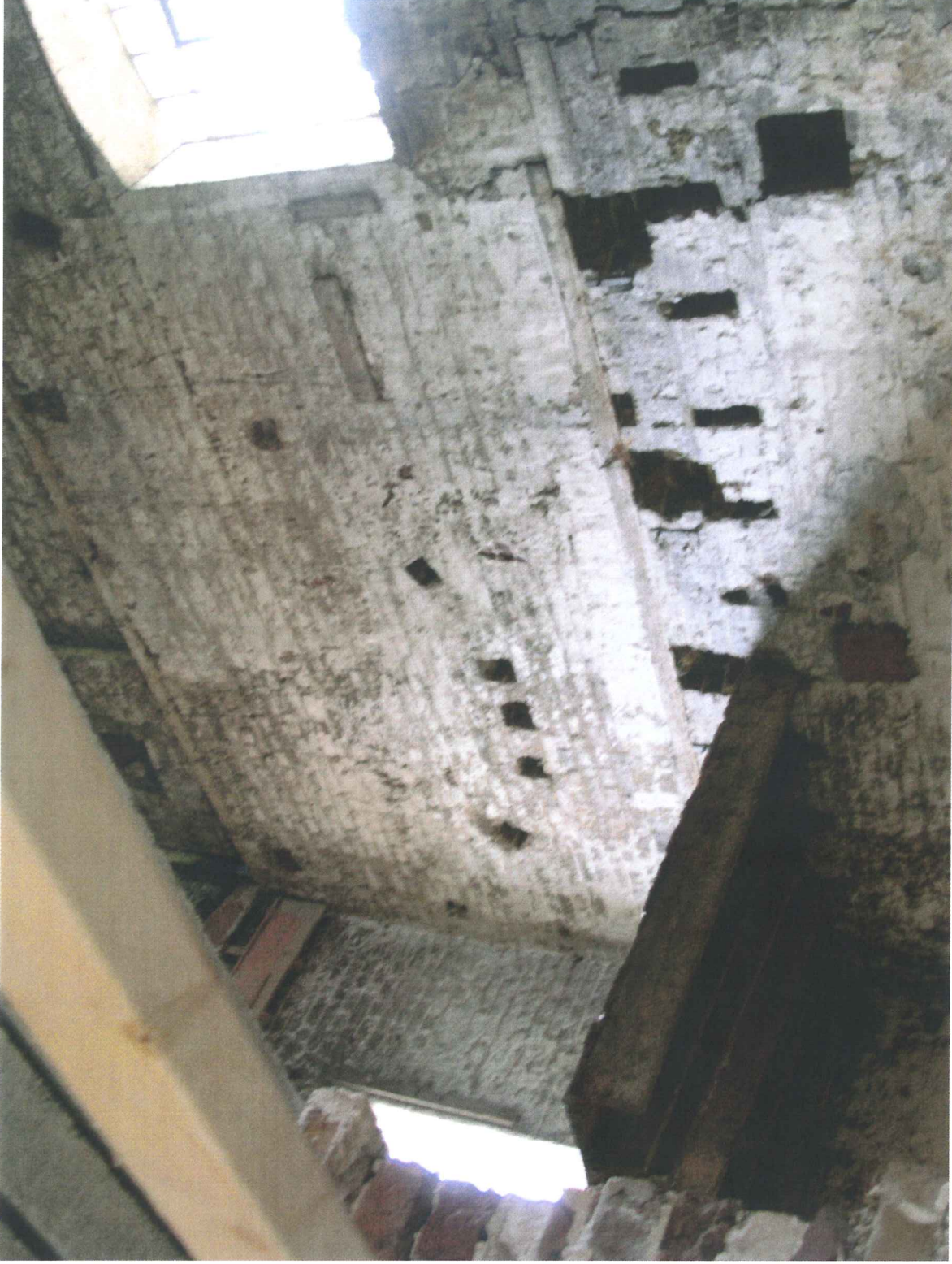
Figure 13 Mortices in the eastern wall of the engine room
