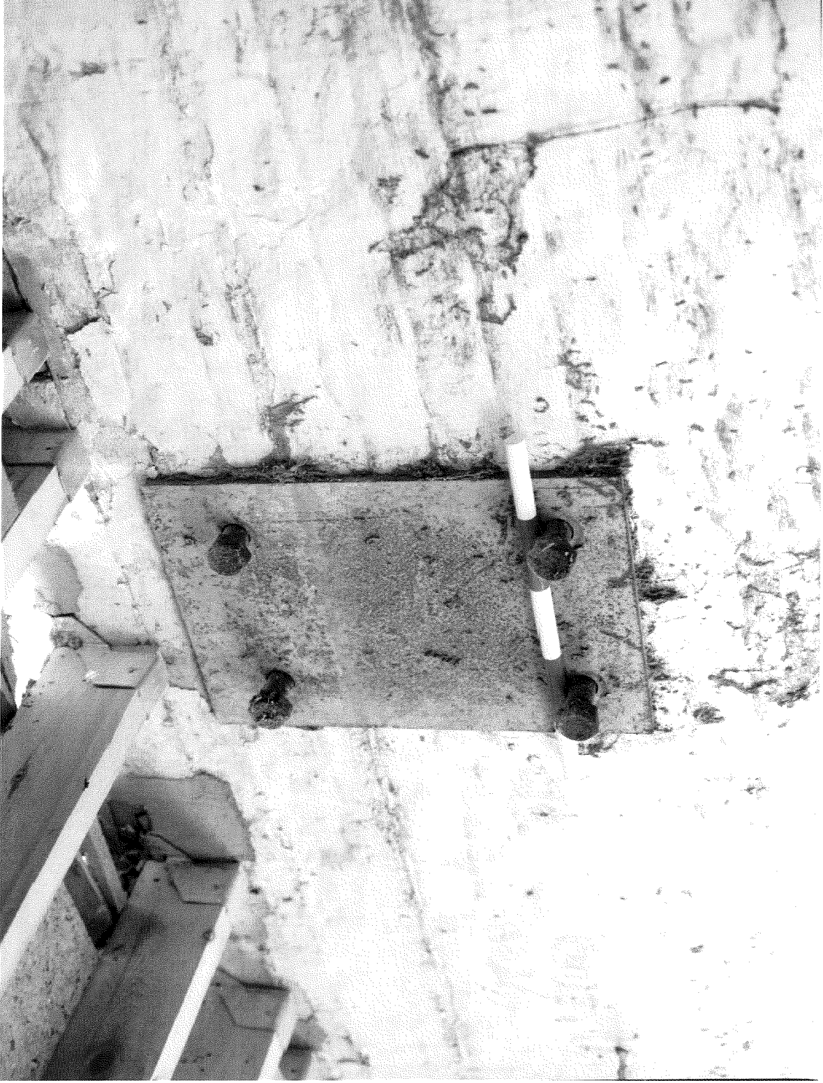
Figure 12 Steel plates for the engine room fittings
