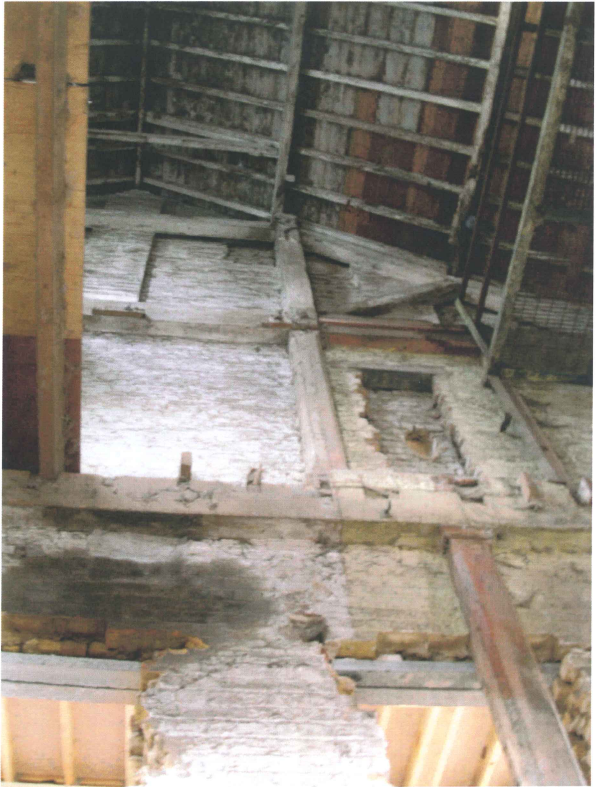
Figure 10 Post structure on the western side of the engine room
