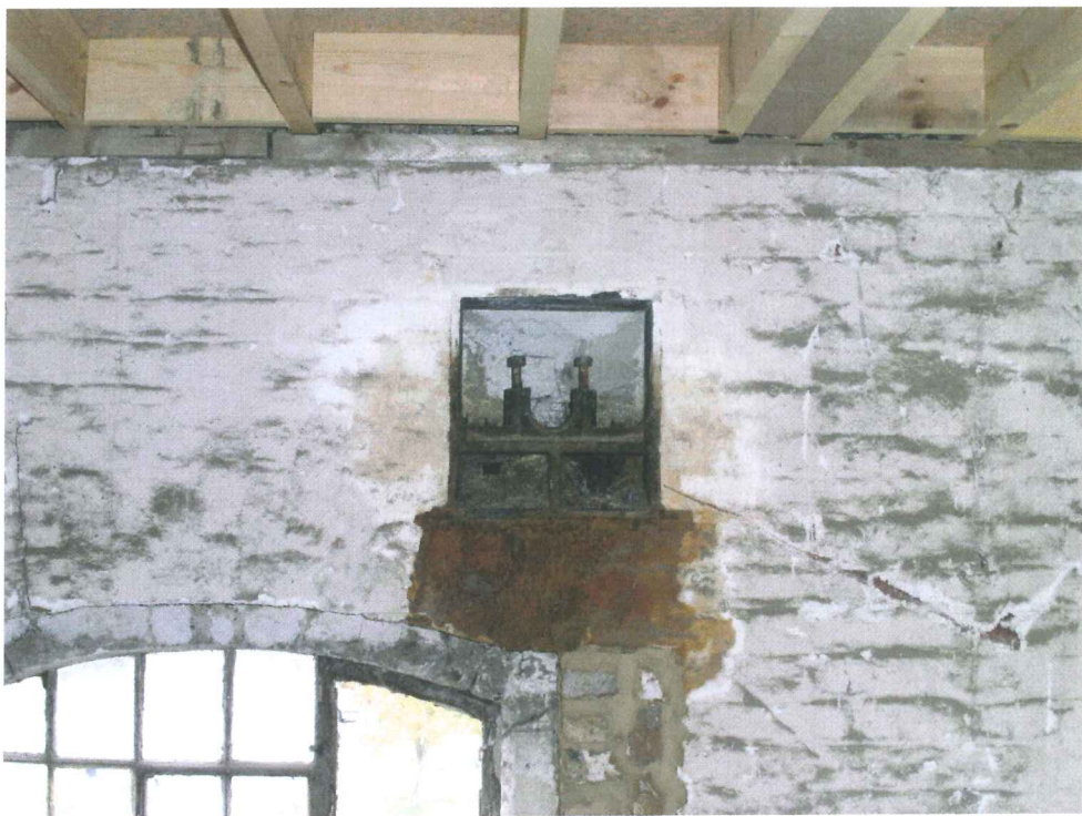
Figure 17 Bearing housing on the western wall of the mill, second floor
