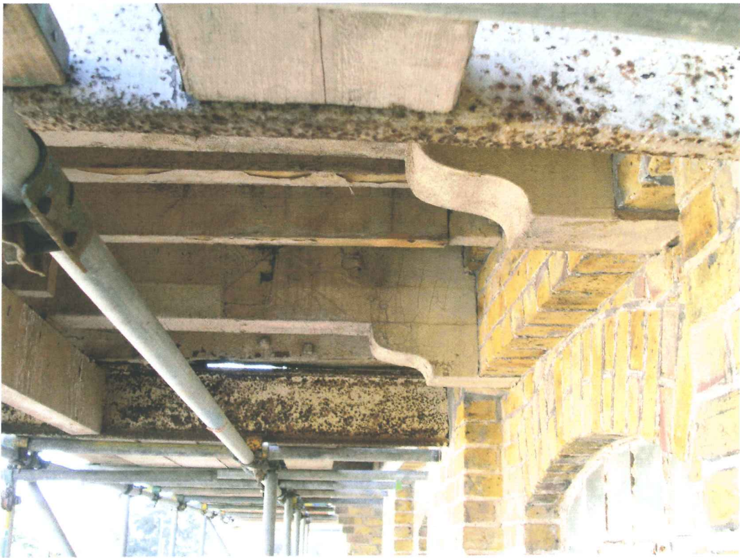
Figure 19 Moulding on the corbels beneath the northern lucam
