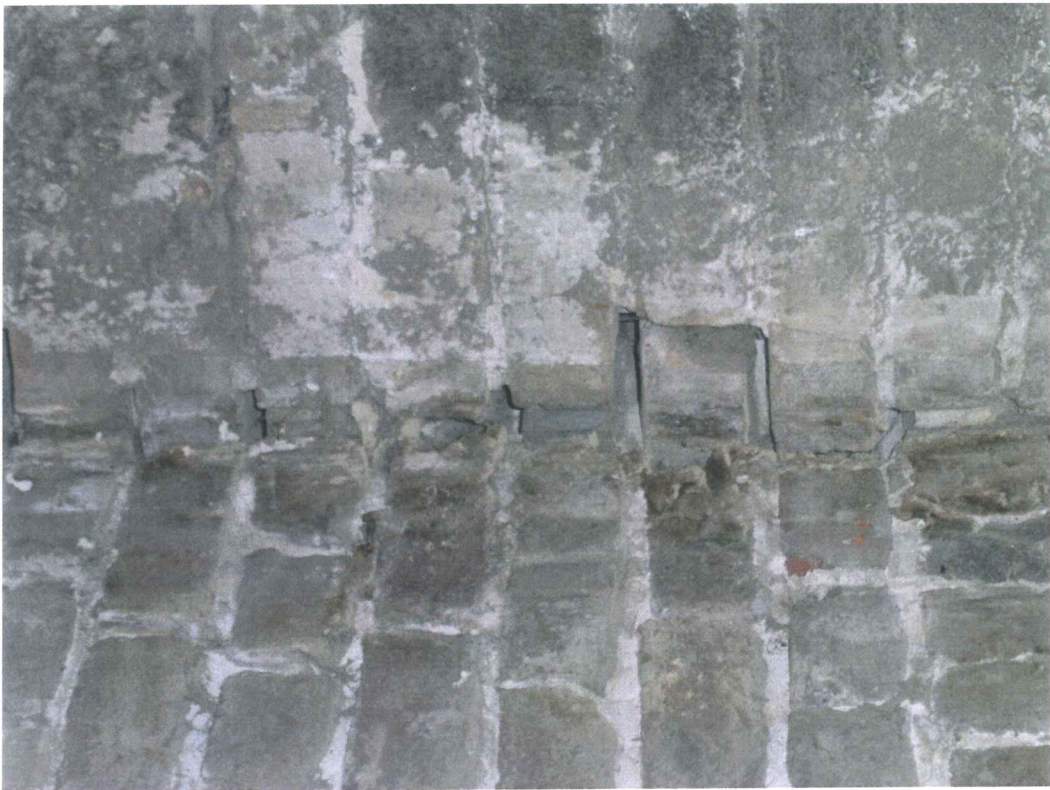
Figure 27 Joint between the firewall and the southern mill wall
