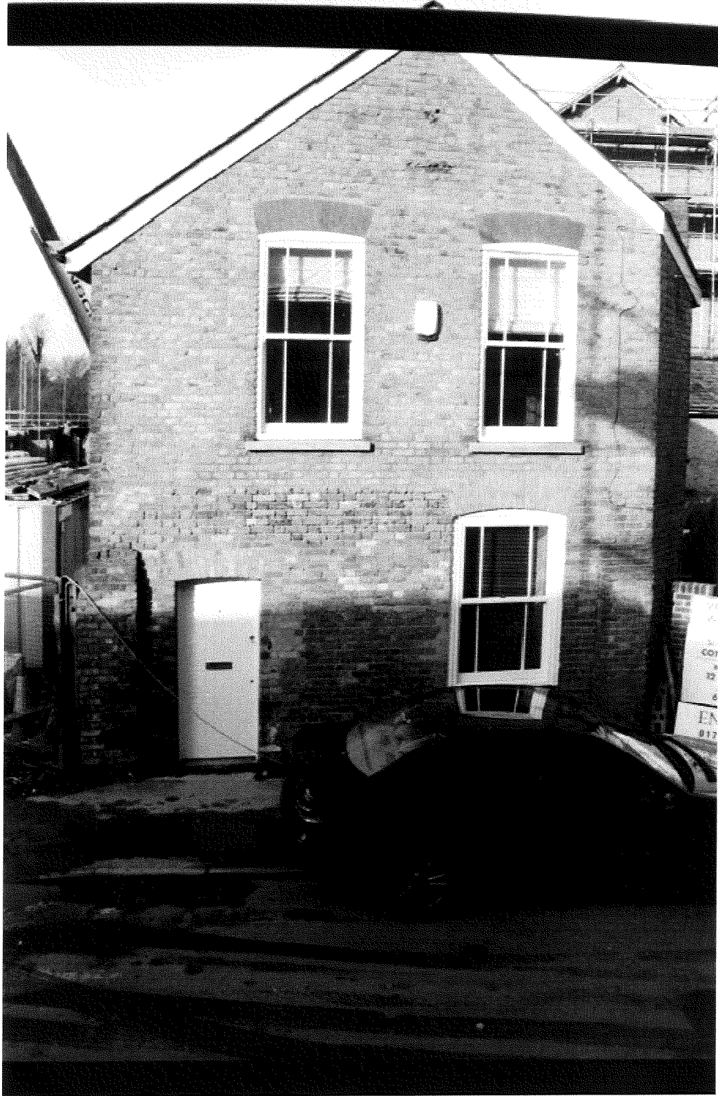
Figure 31 East Elevation of the cottage
