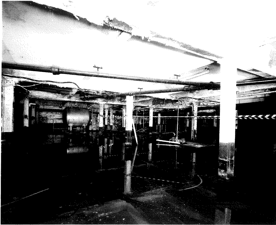
Plate 9: View Of The Flooded Cask Store Basement Looking Southwest
