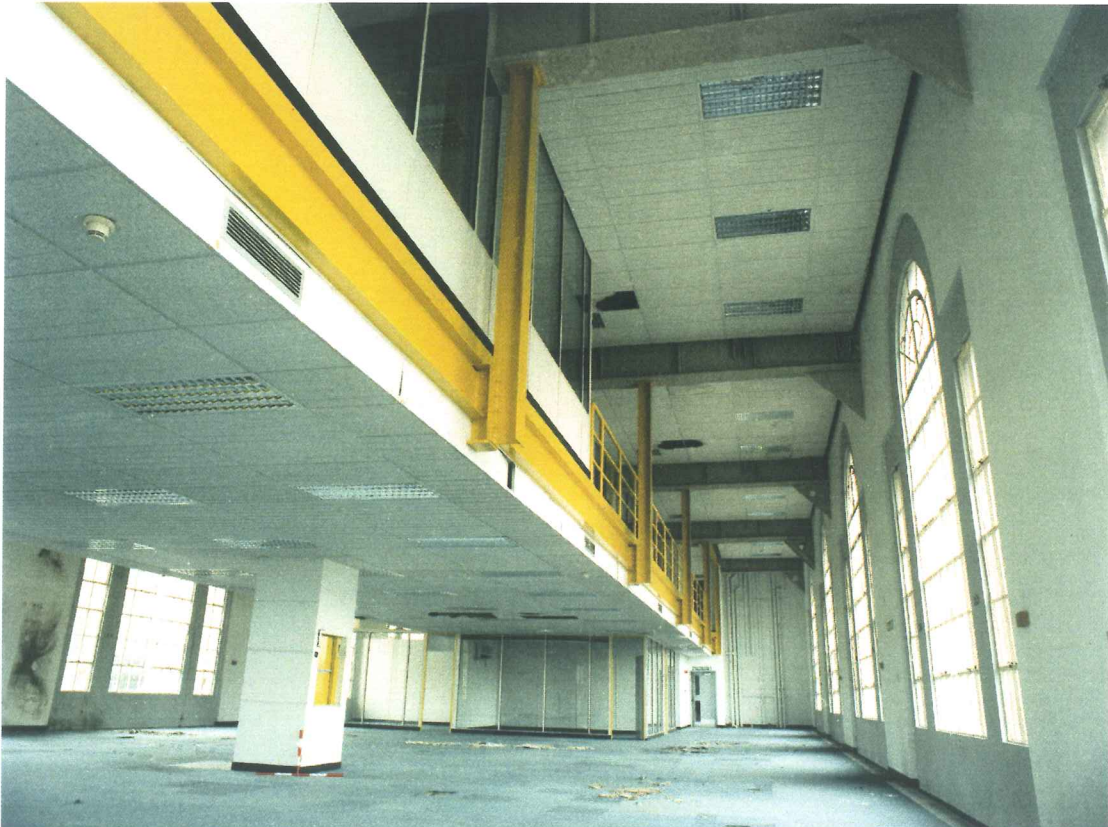
Plate 6: Third Floor Of The Tramway Generator Building
