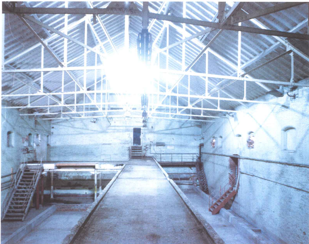
Plate 15: The First Floor Of The Fermentation Building, Southern End
