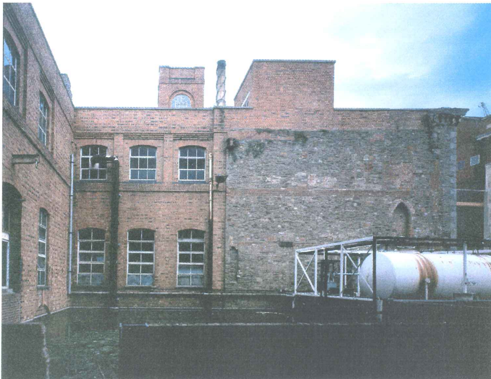
Plate 7: Southwest Elevation Of Georges Building And Cask Store
