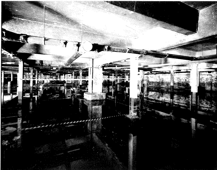
Plate 8: View Of The Flooded Cask Store Basement Looking Southeast
