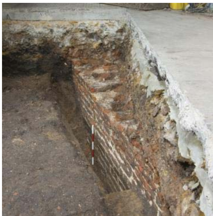
Plate 4. Trench 5, detail of exposed Montagu House boundary wall, looking east.
