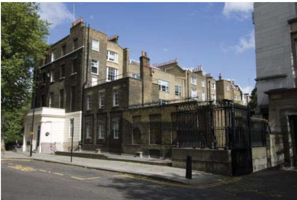
Plate 10. Trench 6, location of workshop looking south east from Montague Place. On the left are the Georgian terraces facing onto Russell Square and on the right is the north eastern corner of the King Edward VII Gallery, with vehicle access to the rear of the British Museum.
