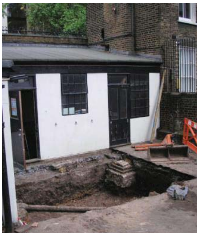
Plate 12. Trench 6, external view of workshop and excavations looking northeast.
