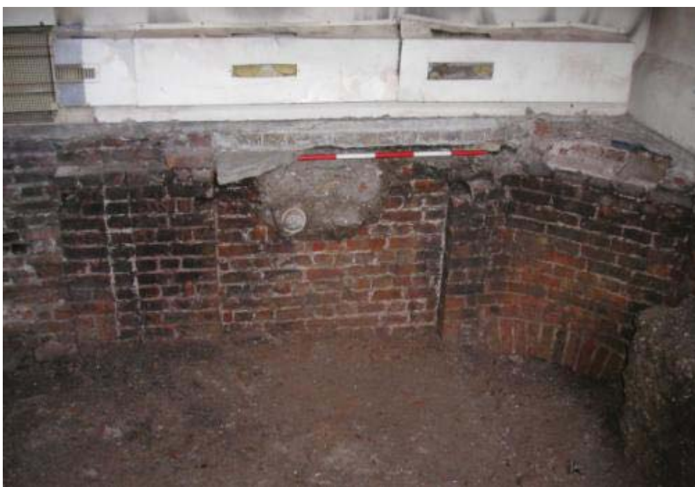
Plate 14. Trench 6, east end of south facing elevation of workshop north wall exposed after porters lodge structure removed. On the right is an angled section of wall forming the chimney breast of a small arched fireplace. In the centre is a blocked doorway that provided access to the basement from Montague Place. On the left is an infilled slot for a partition wall and on the very left the infilled window seen in plate 13.
