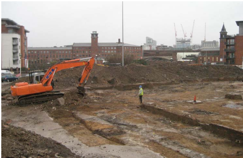
Plate 2. Machine excavation February 2008, north-western part of excavation area, looking north.
