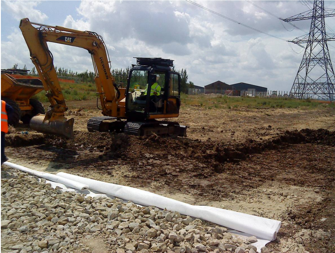
Plate 1: Excavation of the trench for pile caps
