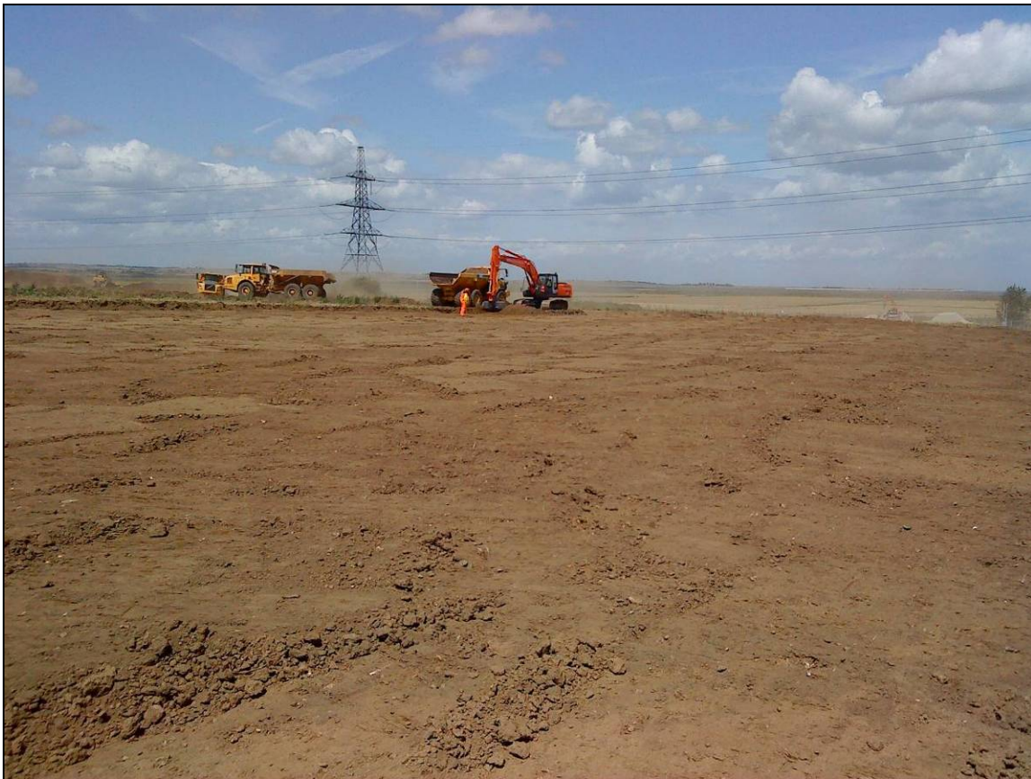
Plate 2: Topsoil stripping
